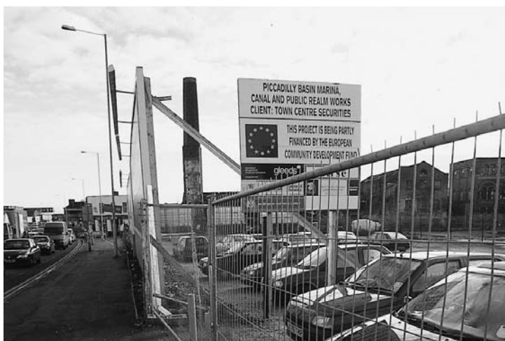
3.3 View of Ancoats in 2001, looking towards the Retail Park (Quarter 2) Source: Gten Photography & Design
