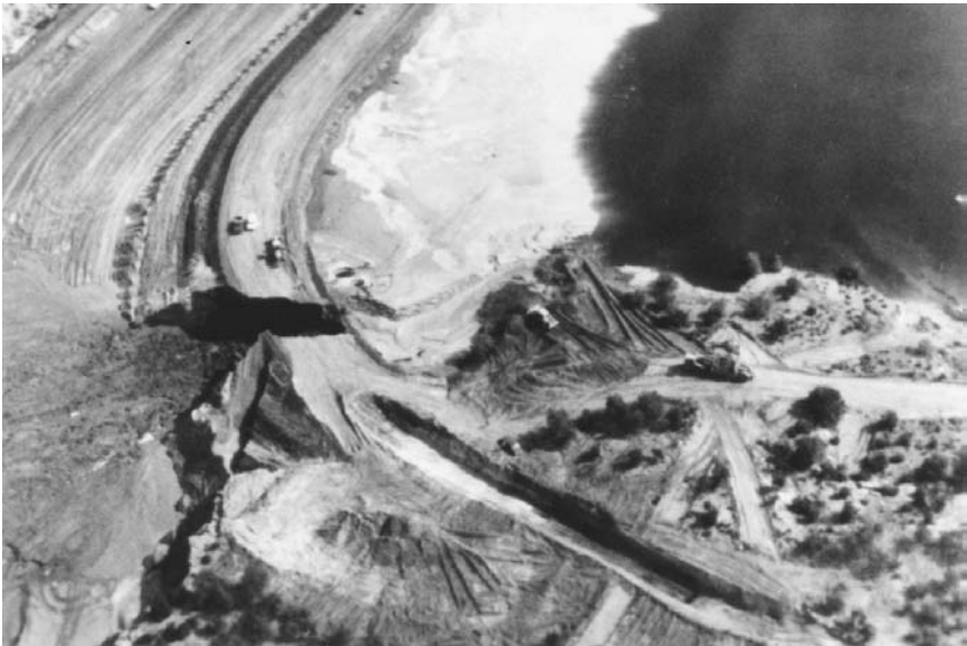
FIGURE 14.16 Breaching of Church Rock Uranium Mill Tailings Dam.
