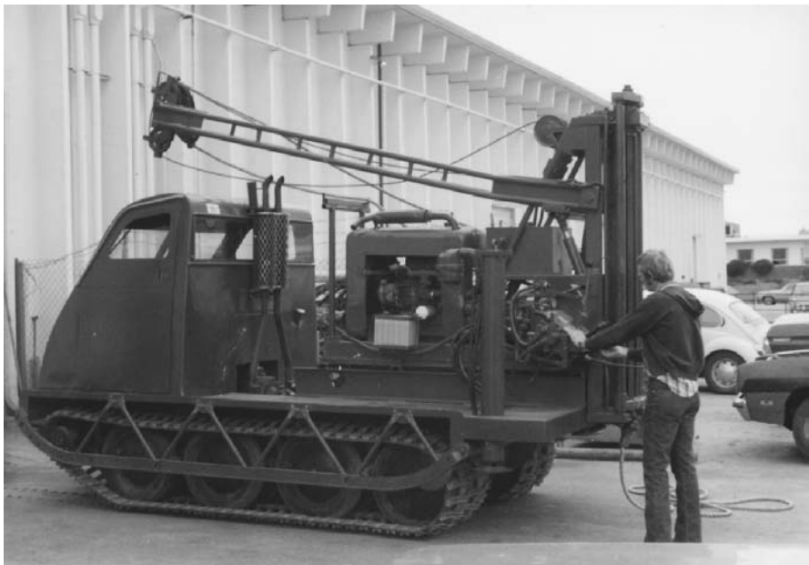
FIGURE 2.3 Tractor-mounted auger drilling rig.
