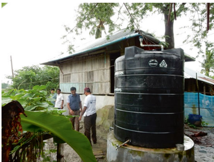
Fig. 15.2 Water tank to collect rainwater
