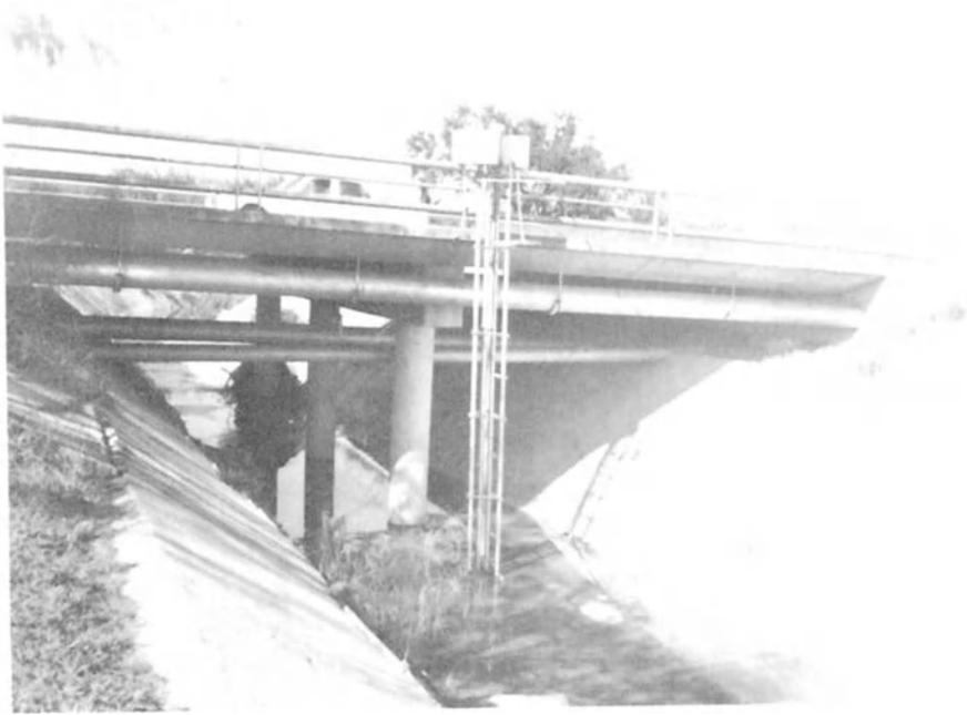
Fig. 2. Conventional urban hydrology gaging system, Alazan Creek, San Antonio, Texas. Photo U.S. Geological Survey.
