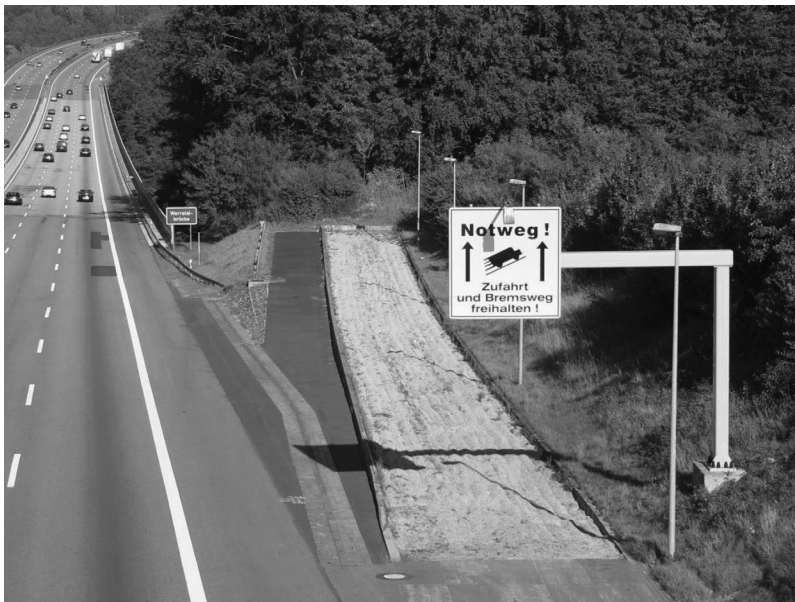
Figure 13.21 Arrestor bed on A5 in Germany.
