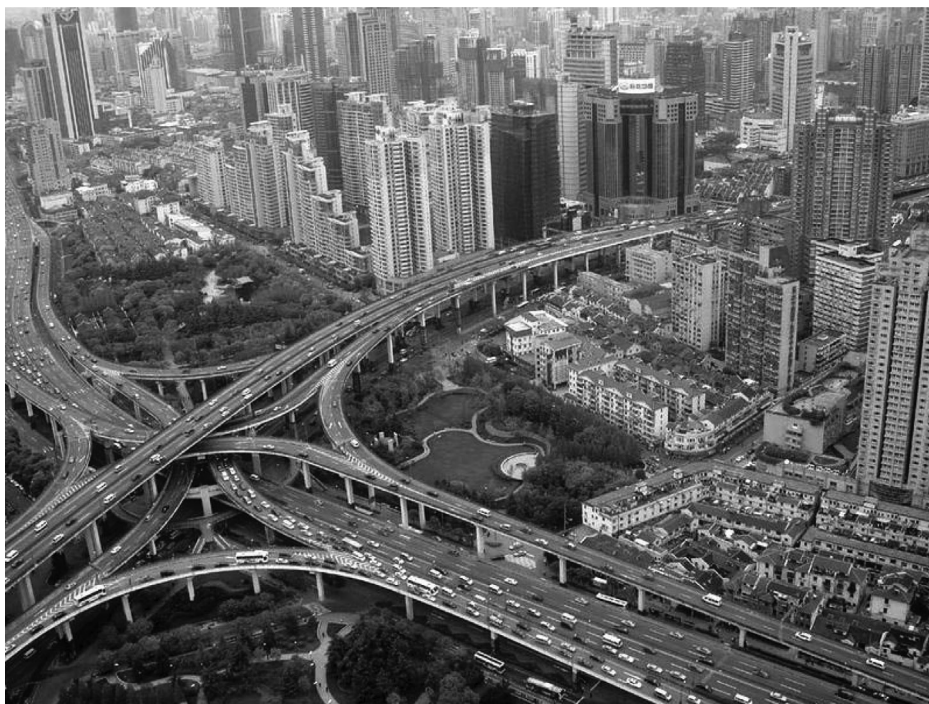
Figure 11.12 A typical four-legged directional interchange.
