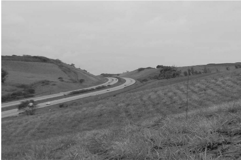
Figure 9.8 The horizontal curve leading the crest curve. (Photo courtesy of RC Burrell.)
