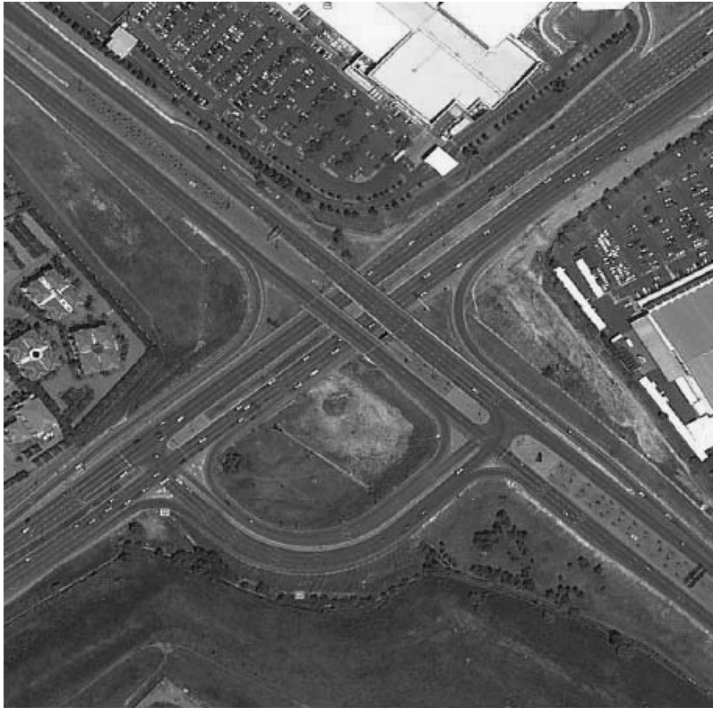
Figure 11.23 Jug handle interchange. (From Leisch JP. Service interchange forms: Adaptability, design features and operational characteristics . Transportation System Planning, Boise, 2002.)
