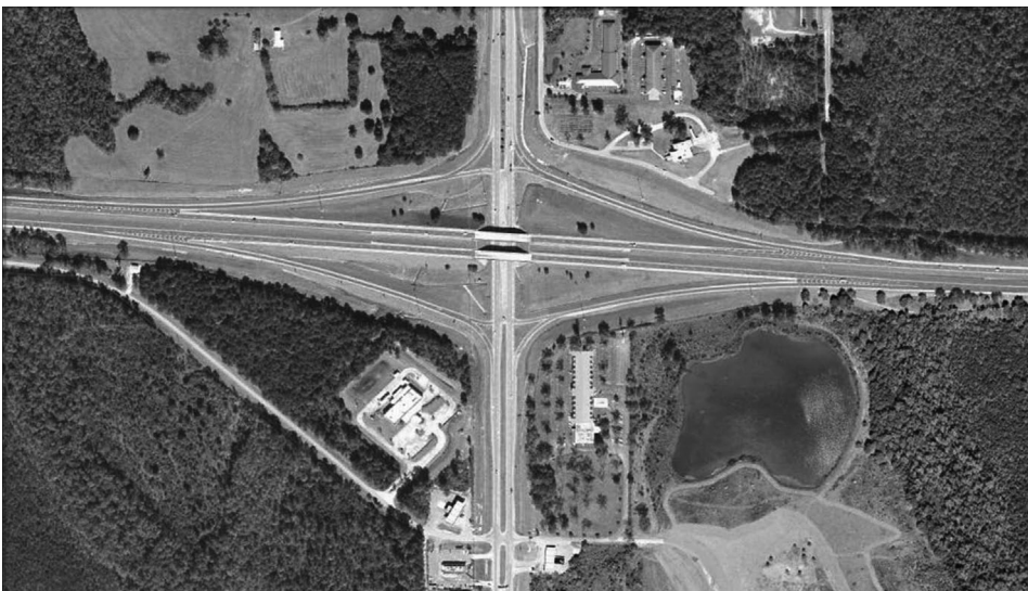
Figure 11.13 The typical diamond interchange in a rural area. (From Leisch JP. Service interchange forms: Adaptability, design features and operational characteristics . Transportation System Planning, Boise, 2002.)
