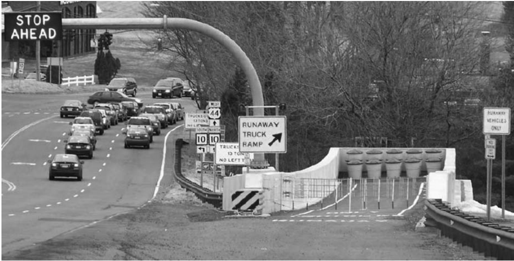
Figure 13.22 Safety net arrestor bed.
