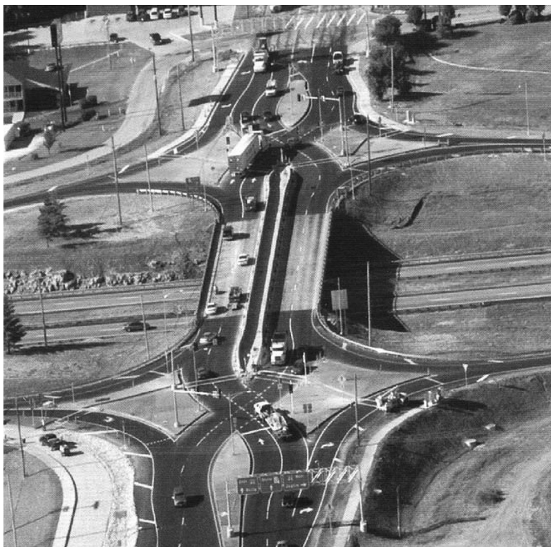
Figure 11.21 The diverging diamond interchange. (From Bared JA. Drivers' evaluation of the diverging diamond interchange . Techbrief FHWA-HRT-07-048, Federal Highway Administration, Washington, DC, 2007.)
