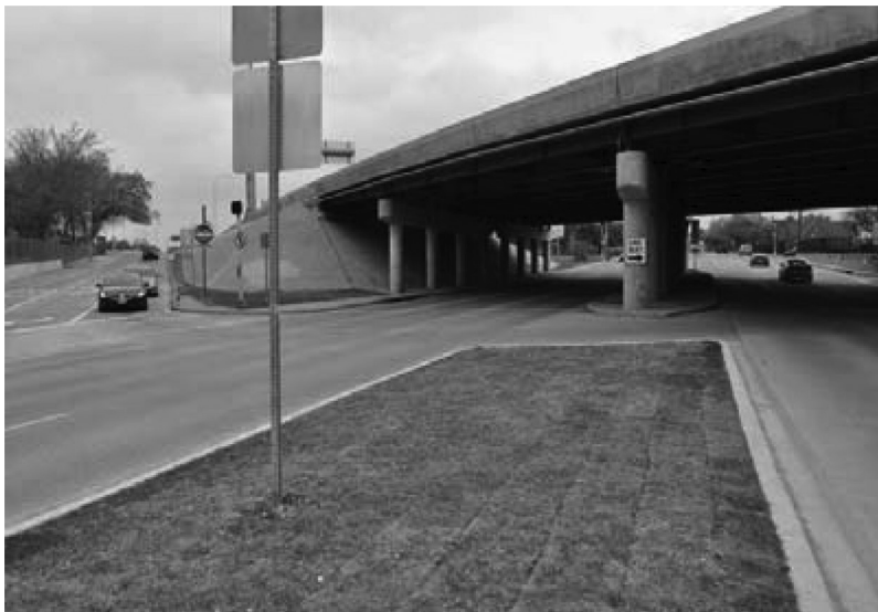
Figure 11.28 A median inhibiting wrong-way driving.
