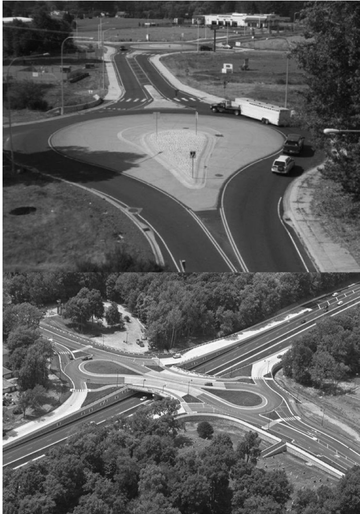
Figure 10.10 The teardrop central island. (From Rodegerdts L et al., Roundabouts: An informational guide . National Cooperative Highway Research Program [NCHRP] Report 672, Transportation Research Board, Washington, DC, 2010.)
