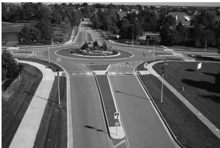
Figure 10.16 Landscaping of the central island. (From American Association of State Highway and Transportation Officials [AASHTO]. A policy on the geometric design of highways and streets . Washington, DC, 2011a.)
