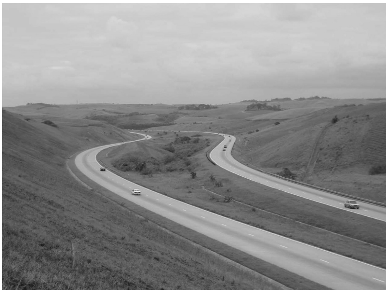
Figure 9.9 Landscaped curvilinear alignment with stream in variable width median. (Photo courtesy of RC Burrell.)
