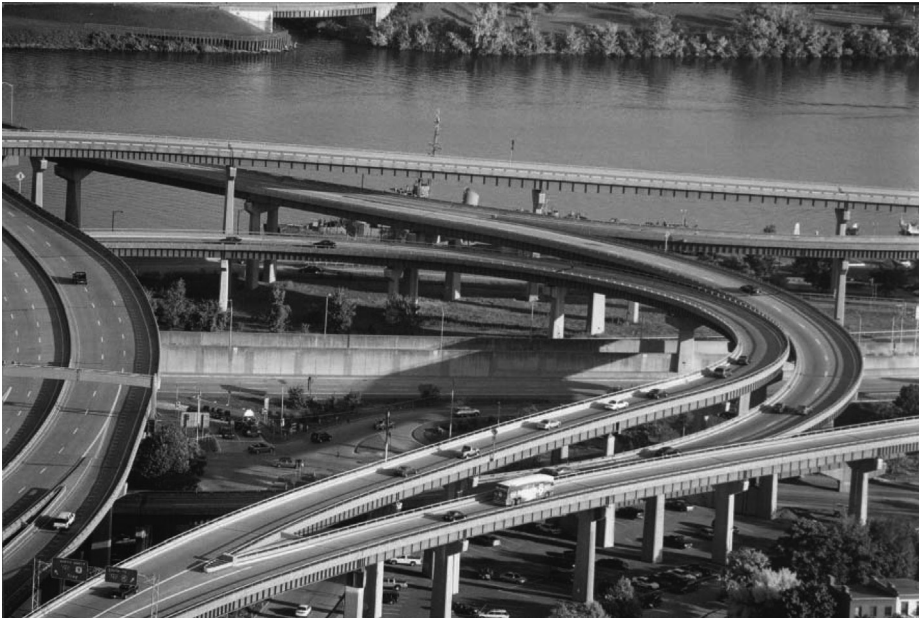
Figure 11.3 Viaduct cross-sections. (From American Association of State Highway and Transportation Officials [AASHTO]. A policy on the geometric design of highways and streets . Washington, DC, 2011a.)
