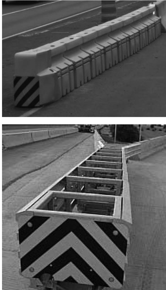
Figure 13.18 Typical proprietary impact attenuators. (From Washington State Department of Transportation. Design manual . Olympia, 2014.)
