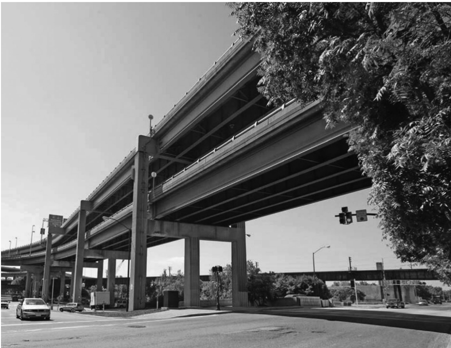
Figure 11.4 Double-decker viaduct. (From American Association of State Highway and Transportation Officials [AASHTO]. A policy on the geometric design of highways and streets . Washington, DC, 2011a.)
