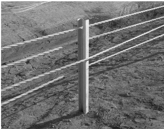
Figure 13.6 Four-cable braided cable system.
