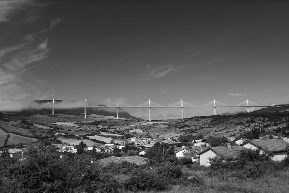
Figure 11.1 Milau Viaduct. (From Wikipedia 2013.)
