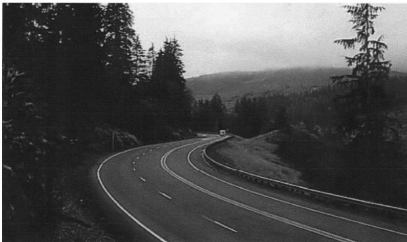
Figure 8.1 A typical passing lane. (From Potts IB and Harwood DW. Benefits and design/location criteria for passing lanes . Missouri Department of Transportation, Kansas City, 2004.)
