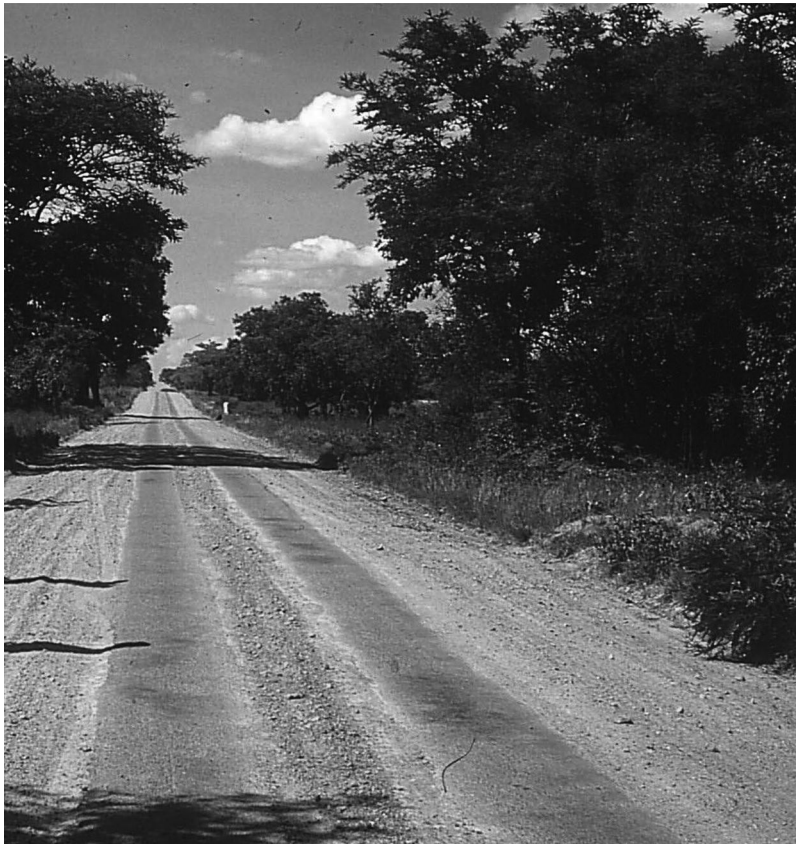
Figure 12.2 Rhodesian strip road. (From Rustyproof, 1963.)
