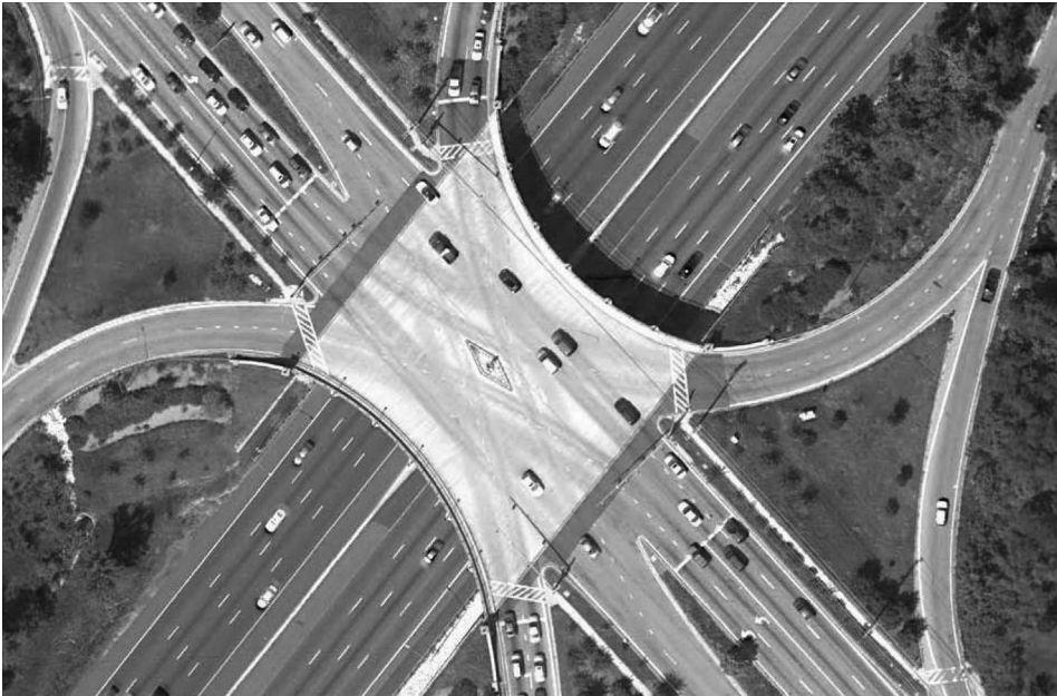
Figure 11.17 The single-point interchange. (From Leisch JP. Service interchange forms: Adaptability, design features and operational characteristics . Transportation System Planning, Boise, 2002.)
