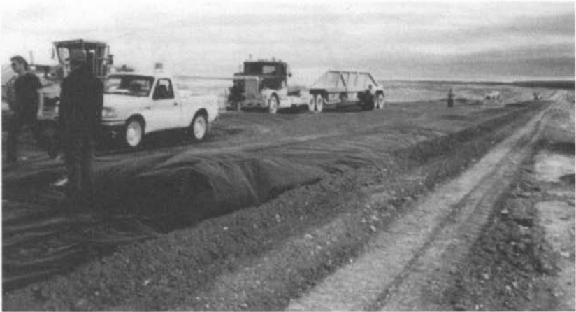
Figure 11-4. A moisture barrier Wyoming project.
