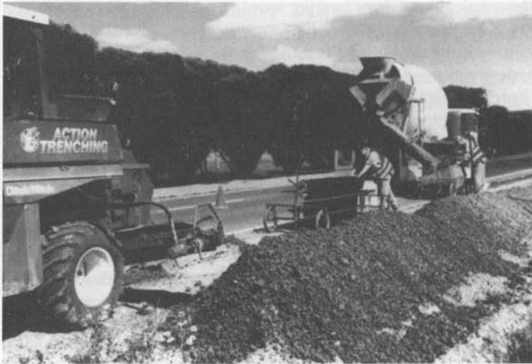
Figure 11-8. Australian trenching for geomembrane placement.
