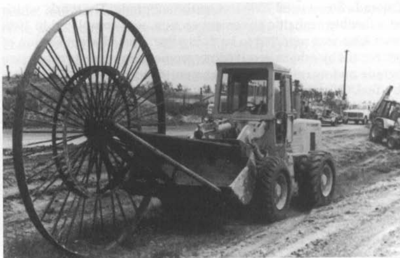
Figure 10-11. A trench compactor on a Texas highway.
