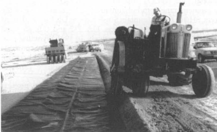
Figure 11-5. Compacting the trench backfill on a Wyoming highway.
