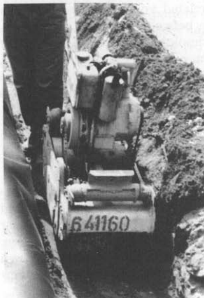
Figure 11-15. A trench compactor on an Israeli highway.
