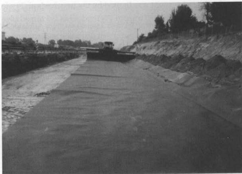
Figure 11-14. An Israeli geomembrane project.
