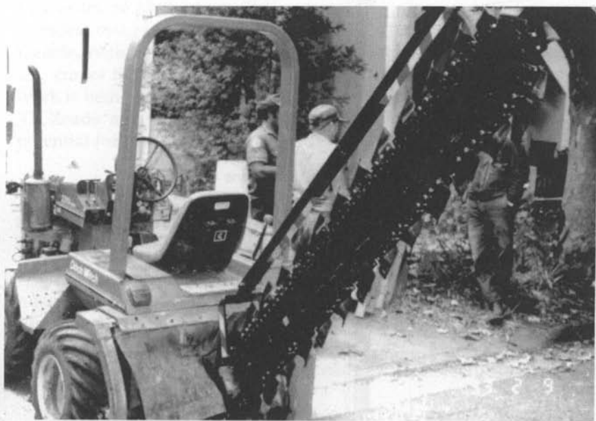
Figure 8-7. New Australian slim-line trencher boom.
