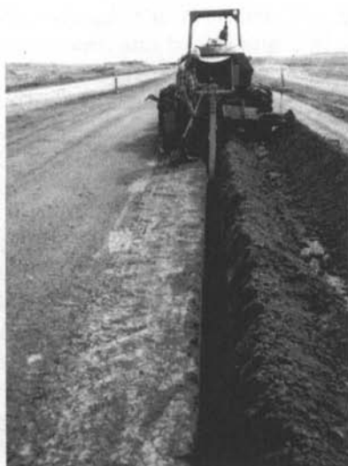
Figure 11-6. Trenching for a vertical barrier on a Wyoming highway.
