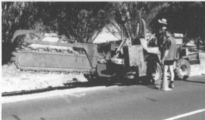
Figure 11-9. An Australian trencher.
