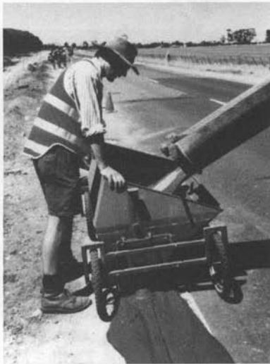
Figure 11-13. Placing a flowable backfill in Australia.
