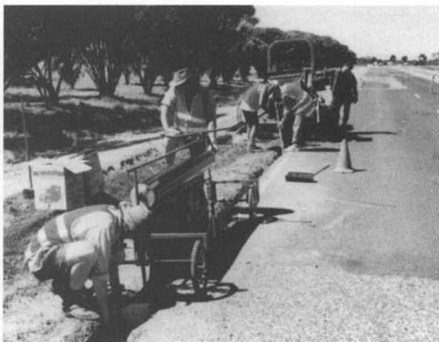
Figure 11-10. The Australian trenching train.
