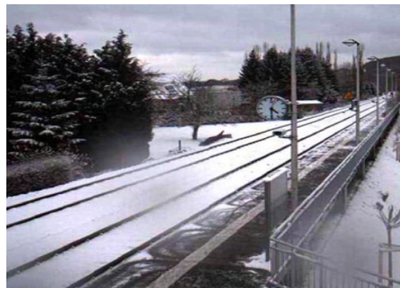
FIG. 10. The Harz platform heating in operation (Eugster, 2007).
