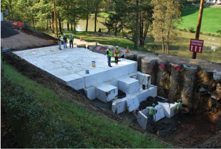
FIGURE 6.3 EPS geofoam as a fill material. (Credit: www.epsindustry.org .)
