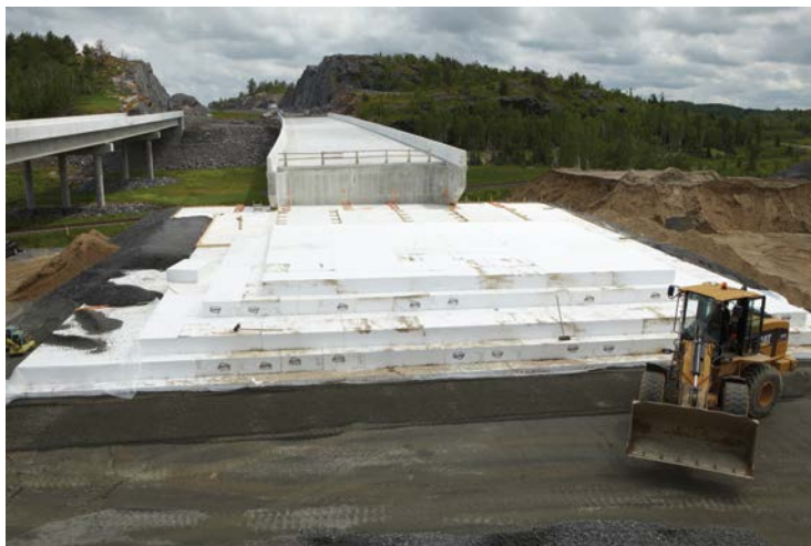
FIGURE 6.2 EPS geofoam as a fill material. (Credit: www.epsindustry.org .)
