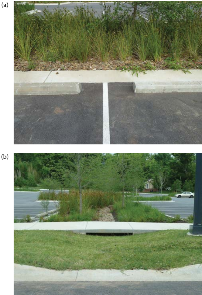
FIGURE 5.4 (a) Water can run directly from parking spaces into a bioretention cell since curbs are not installed. (b) In some locations, curbs direct water to openings that flow to the bioretention cell. Note the sidewalk required a small bridge so pedestrians can cross water flow during heavy rains. (Continued)
