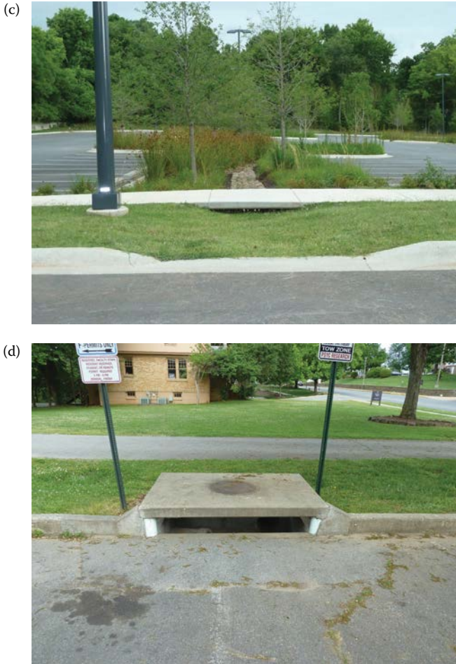
FIGURE 5.4 (Continued) (c) Curbs can divert water to the bioretention cell. (d) A traditional drain leading to the storm sewer, where water is diverted from one location and moved to an alternate location. (Courtesy of A. Braham.)
