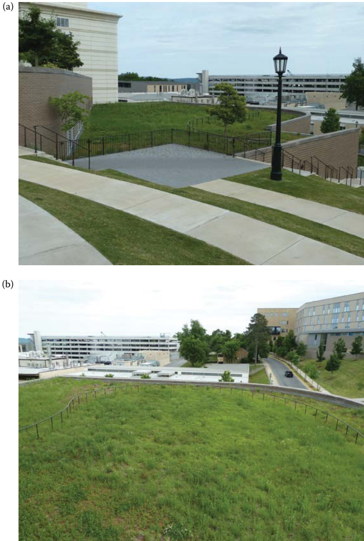
FIGURE 5.1 (a) University of Arkansas Hillside Auditorium green roof. (Credit: A. Braham.) (b) University of Arkansas Hillside Auditorium, green roof foreground, traditional roof background on the Mechanical Engineering building. (Credit: A. Braham.)
