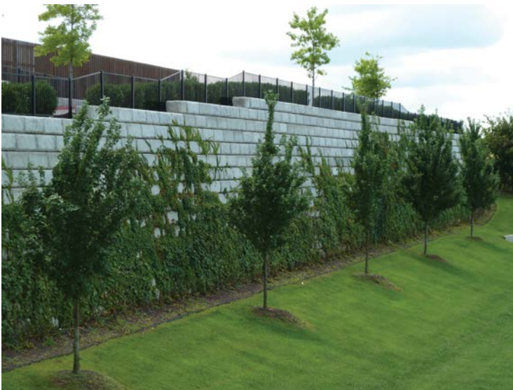
FIGURE 6.11 Stepped MSE wall. (Credit: A. Braham.)
