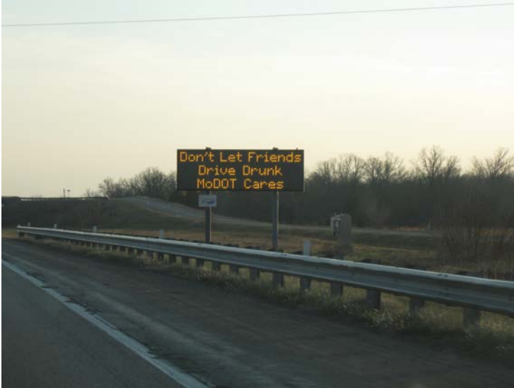
FIGURE 8.5 ITS variable message sign in Missouri. (Credit: A. Braham.)
