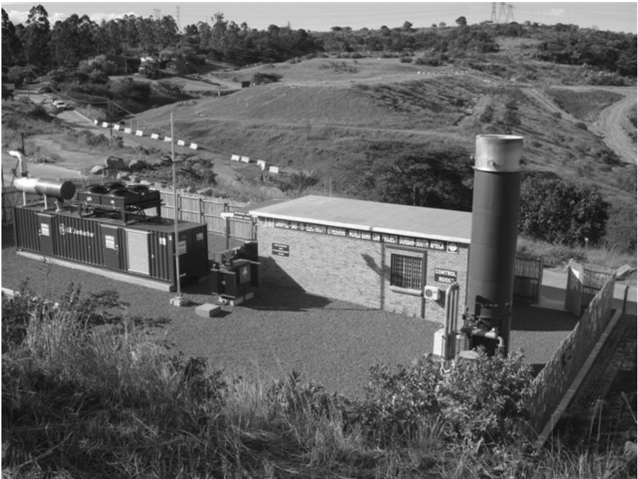
Figure 11.2 Landfill gas-to-electricity installation
