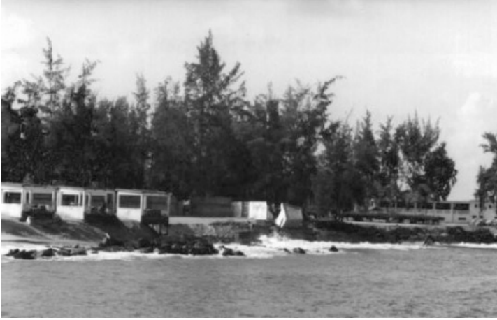
Figure 5.5 Hotel infrastructure (holiday village) being destroyed by coastal erosion
