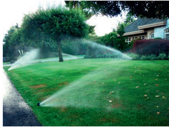
Figure 8.6 Automatic sprinkler system for lawn irrigation in the single-family residential district of Oakridge, Vancouver, Canada (see also Figure 8.7) (Credit: A. Christen).
