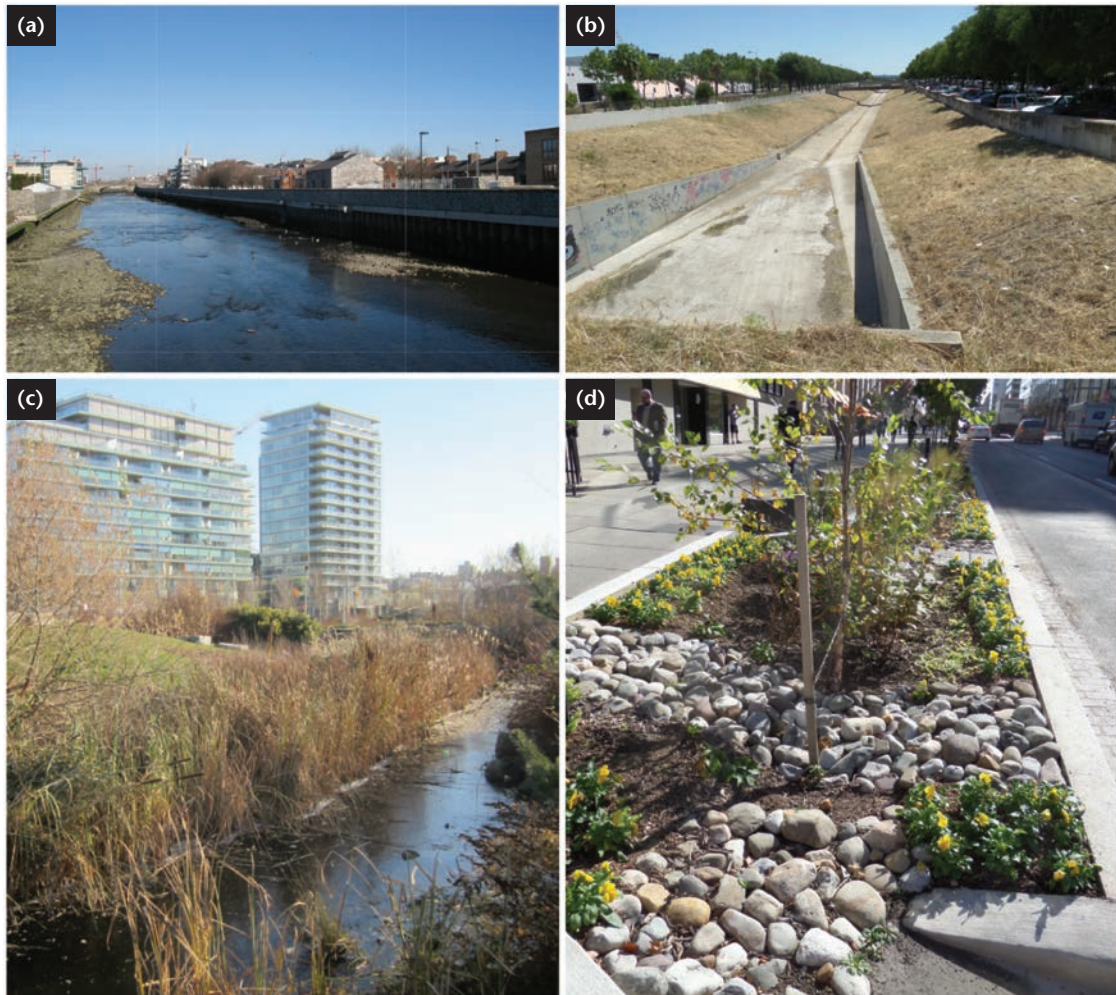
Figure 15.33 Examples of urban runoff management: (a) Conventional flood protection along a river estuary subject to fluvial and coastal flooding in Dublin, Ireland (Credit: G. Mills); (b) a concrete channel used to facilitate the runoff of excess water in Nimes, France (Credit: G. Mills); (c) a managed urban river in Vancouver, Canada, that provides a riparian bank environment and green embankments (Credit: A. Christen) and; (d) a small rain ‘garden’ along a busy street in Washington DC, United States, that allows water to permeate the surface cover (Credit: G. Mills).
