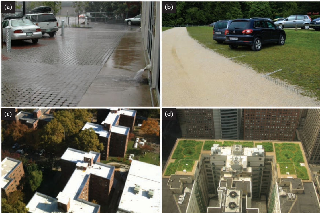
Figure 15.14 Facet interventions to manage water and energy exchanges. (a) Permeable paving using modular blocks (Credit: B. Wenk). (b) Permeable car park with a grass cover (Credit: A. Christen). (c) White painted rooftops or cool roofs New York (United States). (Credit: White Roofs Project). (d) An extensive green roof on Chicago City Hall, United States, as part of a cool roof project (Credit: Tony the Tiger, July 2008).
