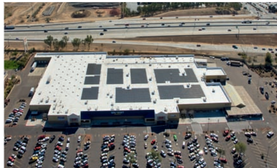
Figure 14.18 A large retail shop in Arizona, United States, that has taken steps to reduce its energy demand by using a white-coated roof to reflect solar radiation and installing solar panels to generate a portion of the building's energy needs (Source: Walmart; CC2.0).
