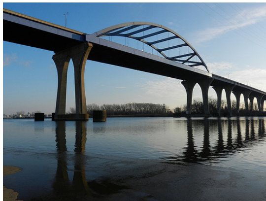
Fig. 8 Leo Frigo Memorial Bridge, Green Bay, Wisconsin
