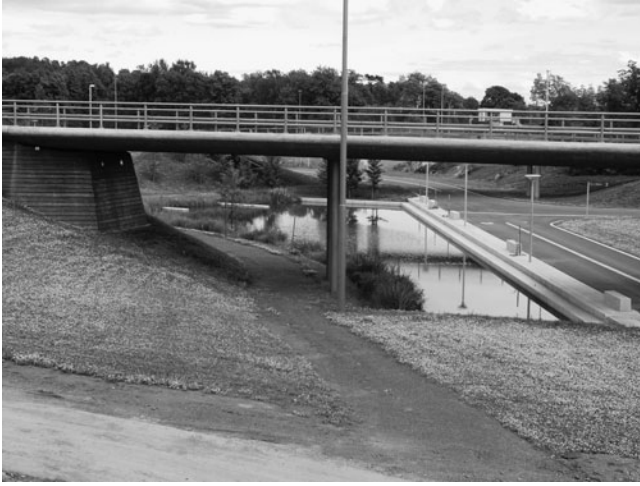
FIGURE 9.2 A wet pond receiving highway runoff. The pond is located in a property development, Fornebu, in Oslo, Norway. The area was, until 1998, the airport of Oslo. The “permanent water volume” is in this case dominating compared with the “storage volume” (cf. Example 9.1).
