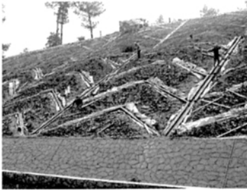
Photo 1. Treating slope with root pile
