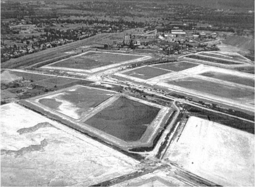
Figure 4: A typical complex of hydraulic-fill ring-dyke impoundments for gold tailings at a South African gold mine. The impoundment at lower left is being reclaimed for further gold extraction.
