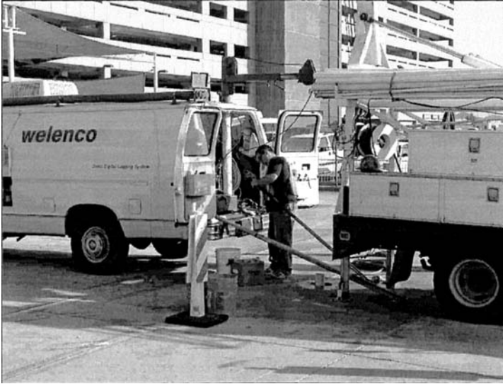
Figure 3. Downhole geophysical methods operation.
