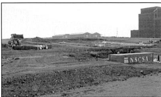
Figure 3. Lysimeters during construction (project trailer is on the right).
