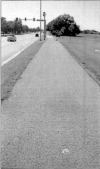
Figure 2a. Test section showing no cracks, looking west.
