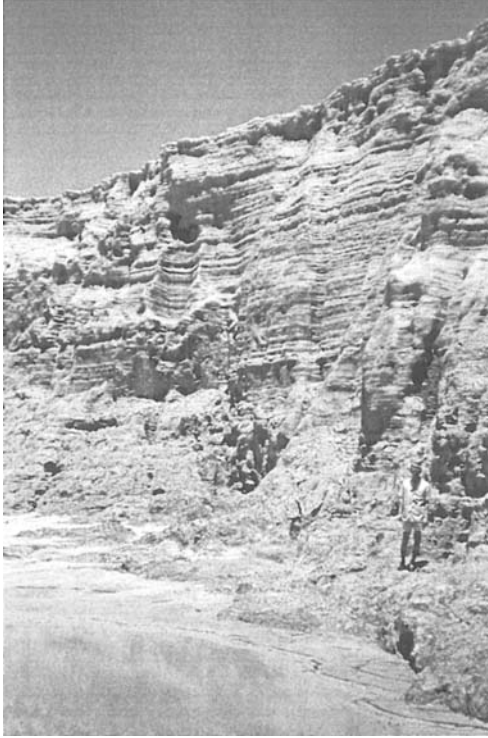
Figure A2: Photograph of a vertical tailings slope 8 m high, with the phreatic surface at its base.
