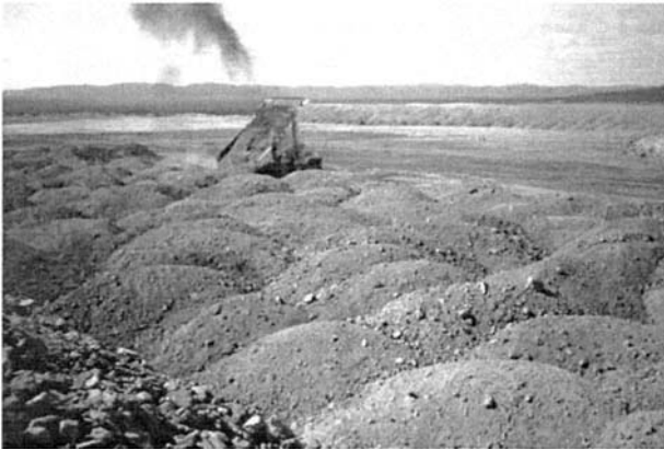
Figure 2. Placement of rocky soil mulch layer on South Dump cover trial.
