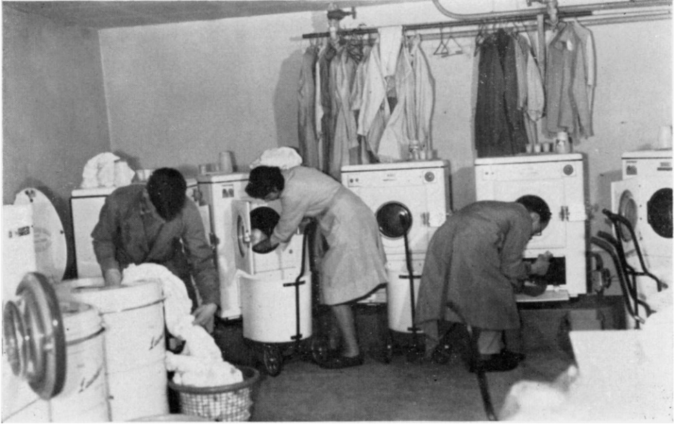
Fig. 2. The laundry wash-house. Simple Bendix equipment is installed.
