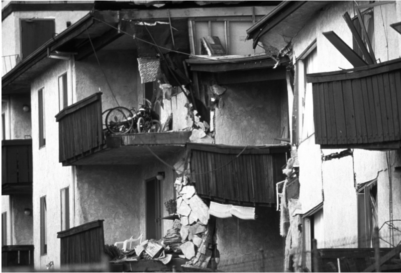
Figure 2.3 Northridge Earthquake, California, January 17, 1994. Buildings, cars, and personal property were all destroyed when the earthquake struck. Approximately 114,000 residential and commercial structures were damaged, estimated at $25 billion. (From FEMA.)
