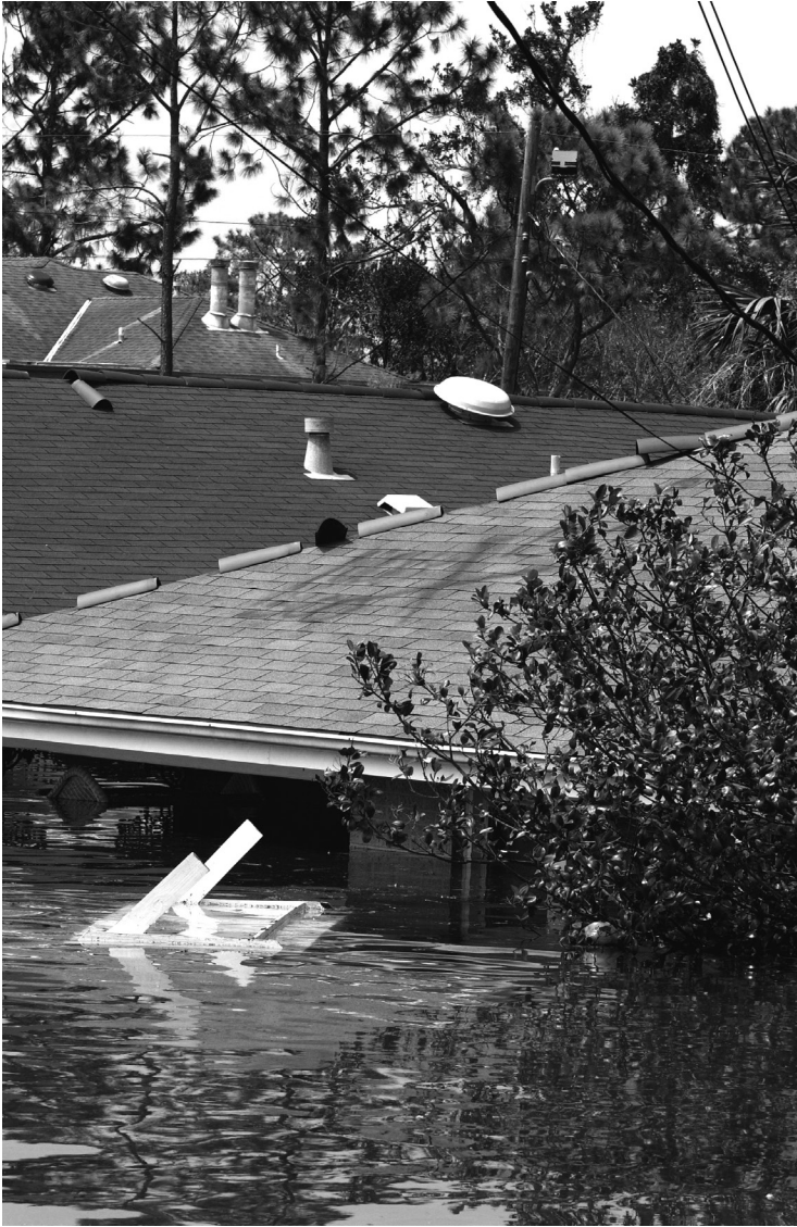
Figure 2.6 New Orleans, Louisiana, August 30, 2005. A New Orleans neighborhood inundated with floodwaters to the eaves of homes. The roof was marked by a FEMA Urban Search and Rescue (USR) team telling authorities that the structure has been searched for people. (Photo by Jocelyn Augustino/FEMA.)
