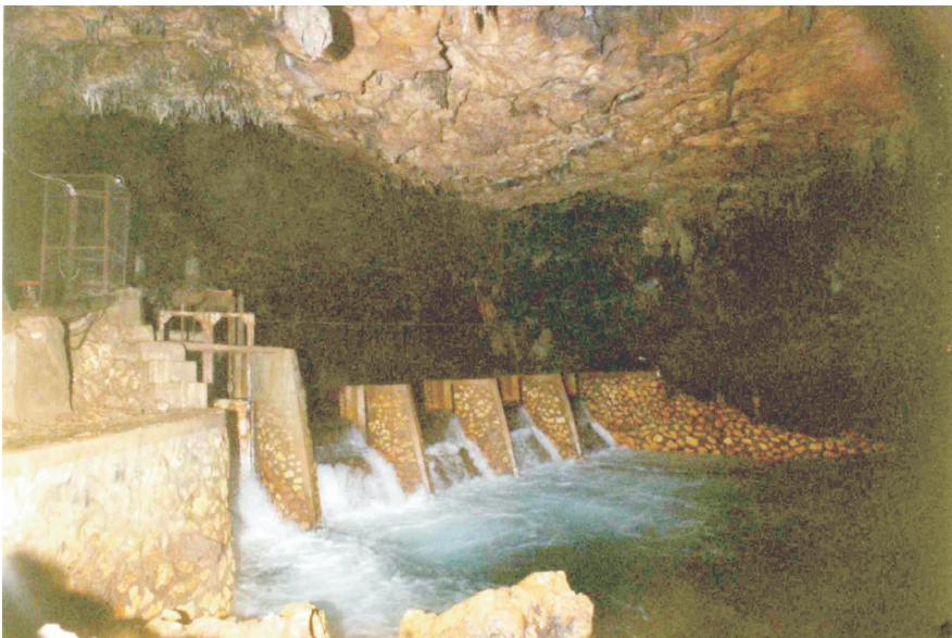
Figure 4. Underground dam of the Bribin scheme built in 1981. (From University of Karlsruhe, University of Karlsruhe, Institute of Aquatic Environmental Engineering, http://www.hoehlenbewirtschaftung.de/English/English.html .)
