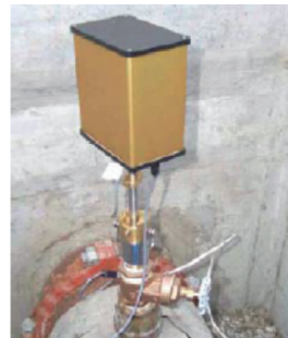
Six-CENSE™ Insertion into Pipe
