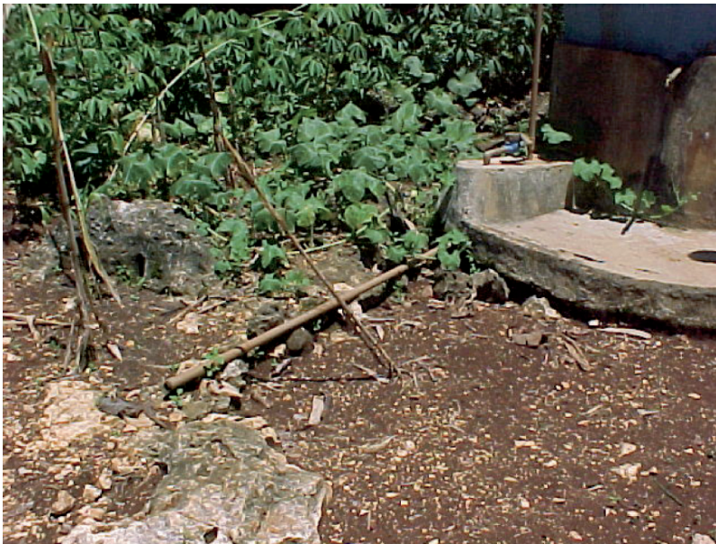
Figure 7. Demounted water pipe at the foot of a cistern in Gunung Sewu. (Courtesy of H. Lehn.)
