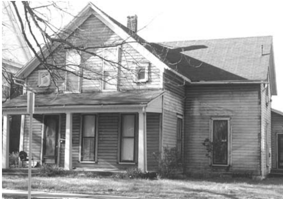
Figure 2.12 Old house with exterior lead-based paint.
