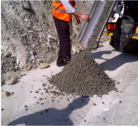
Figure 3. Returned Ready-Mix concrete
