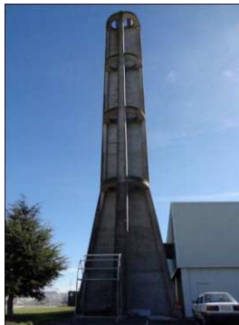
Figure 1. Chimney with rocking ability.
