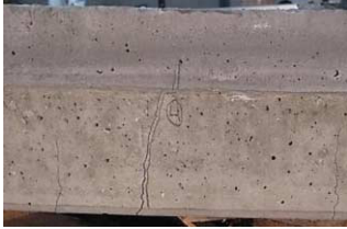
Figure 7. Crack offset
