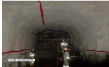
Figure 4. Finished tunnel with the TSL product[4]
