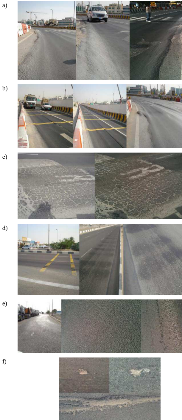
Figure 2. Pavement problems field study in Abu Dhabi, UAE: a) Mix rutting (Al Salam Street), b) Subgrade rutting (Al Salam Street), c) Fatigue cracking (Musaffah M10), d) Bleeding (Mohammad Bin Zayed) e) Raveling (Musaffah M15) and f) Potholes (Khalidiyah Street).
