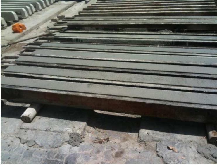
Figure 4. Following the completion of casting, elements were placed in a pre-designated area, and allowed to cure
