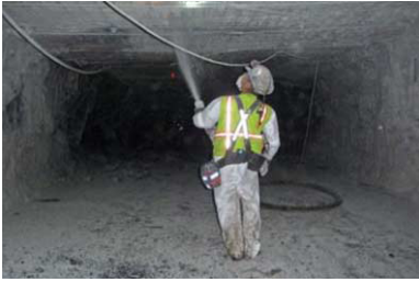
Figure 1. Thin sprayed rock liner being sprayed[4]
