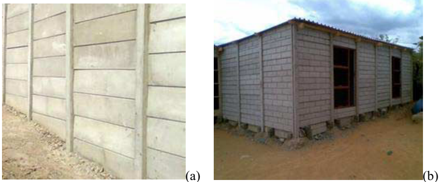
Figure 1. (a) Precast concrete fence wall and (b) Complete precast concrete fence walled house
