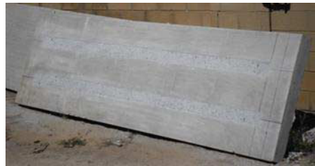
(b) Completed scabbled surface
