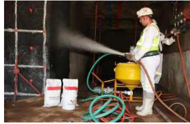
Figure 2. TSL layer easily applied by one person[4]
