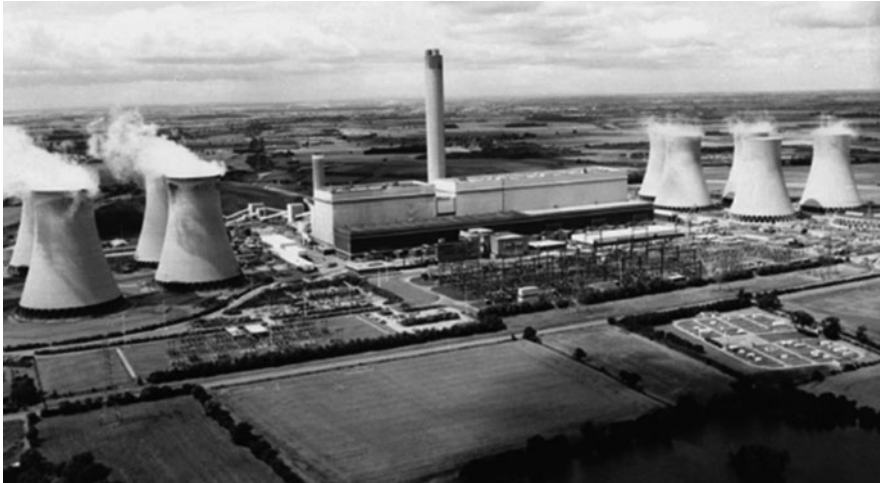
Fig. 15 Atmospheric cooling tower
