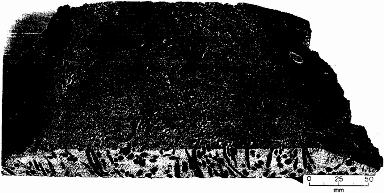
Fig. 13.1 Teredo attack on timber. (Crown copyright reproduced with the permission of BRE, Princes Risborough Laboratory.)
