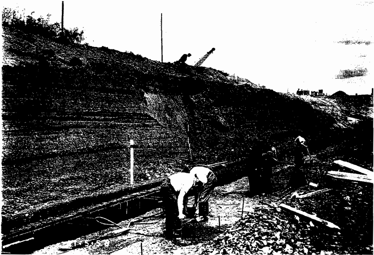
Fig. 9.3 Minor slipping from 1 : \frac{1}{2} slope in stiff-fissured London Clay, Middlesex. Note smooth appearance of fissure planes.
