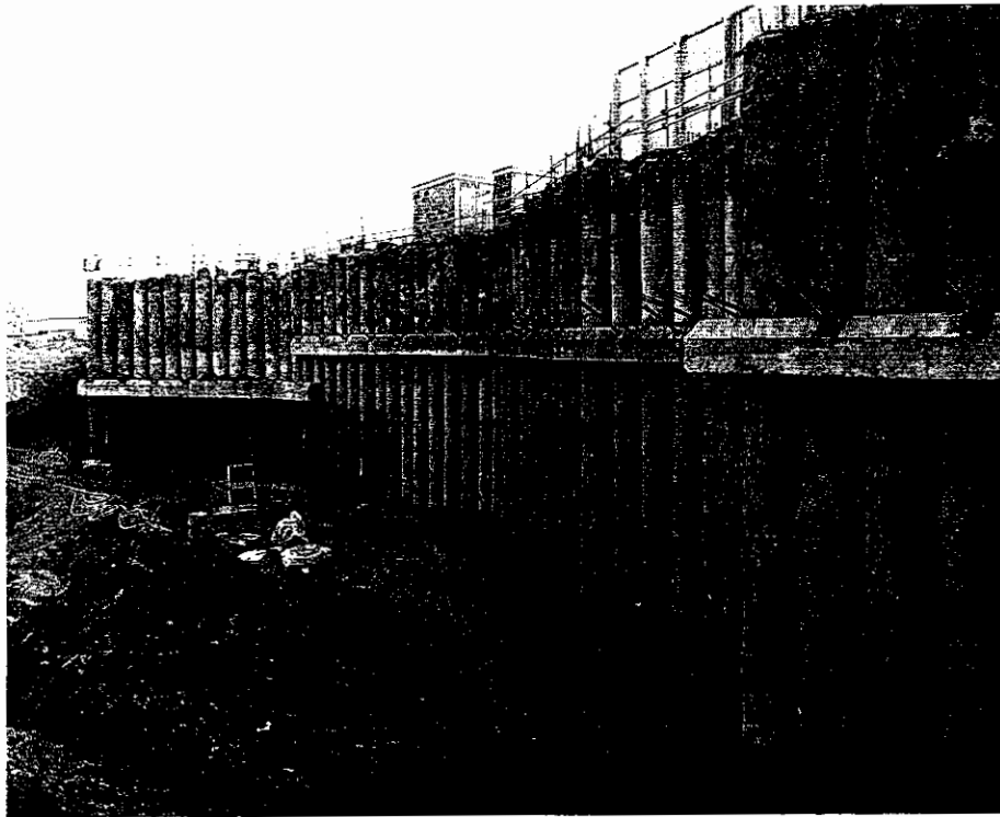
Fig. 10.30 A contiguous bored pile retaining wall supported by ground anchors and reinforced cast-in-place walings.
