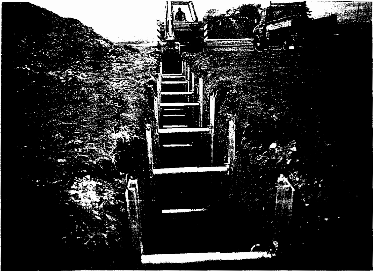
Fig. 9.18 A movable support system for trench excavations.
