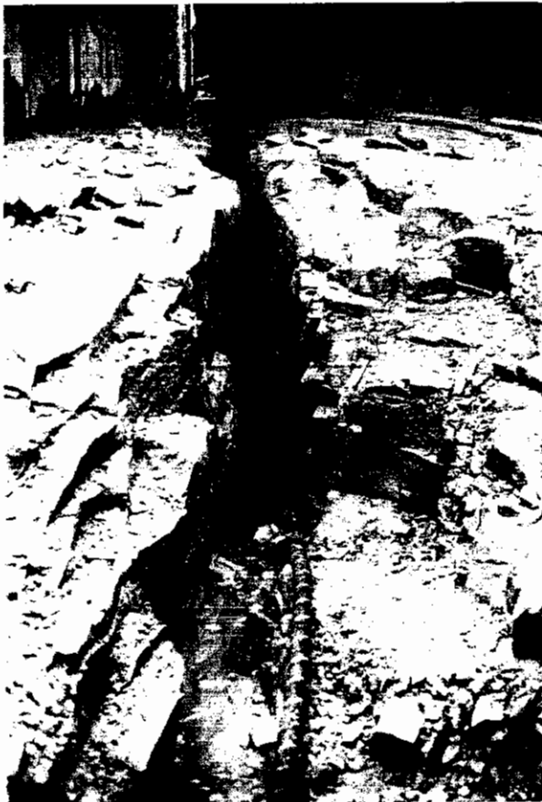
Fig. 6.20 Fissure in rock surface at foundation level of west abutment, Twizel Bridge (courtesy of Director of Technical Services, Northumberland County Council).
