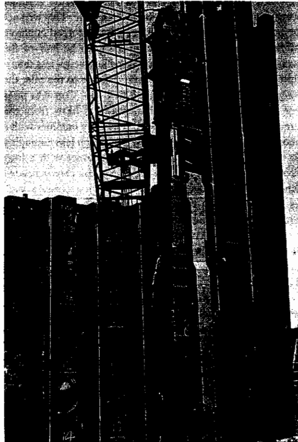
Fig. 8.8 The BSP HH7 hydraulic hammer driving steel sheet piles.
