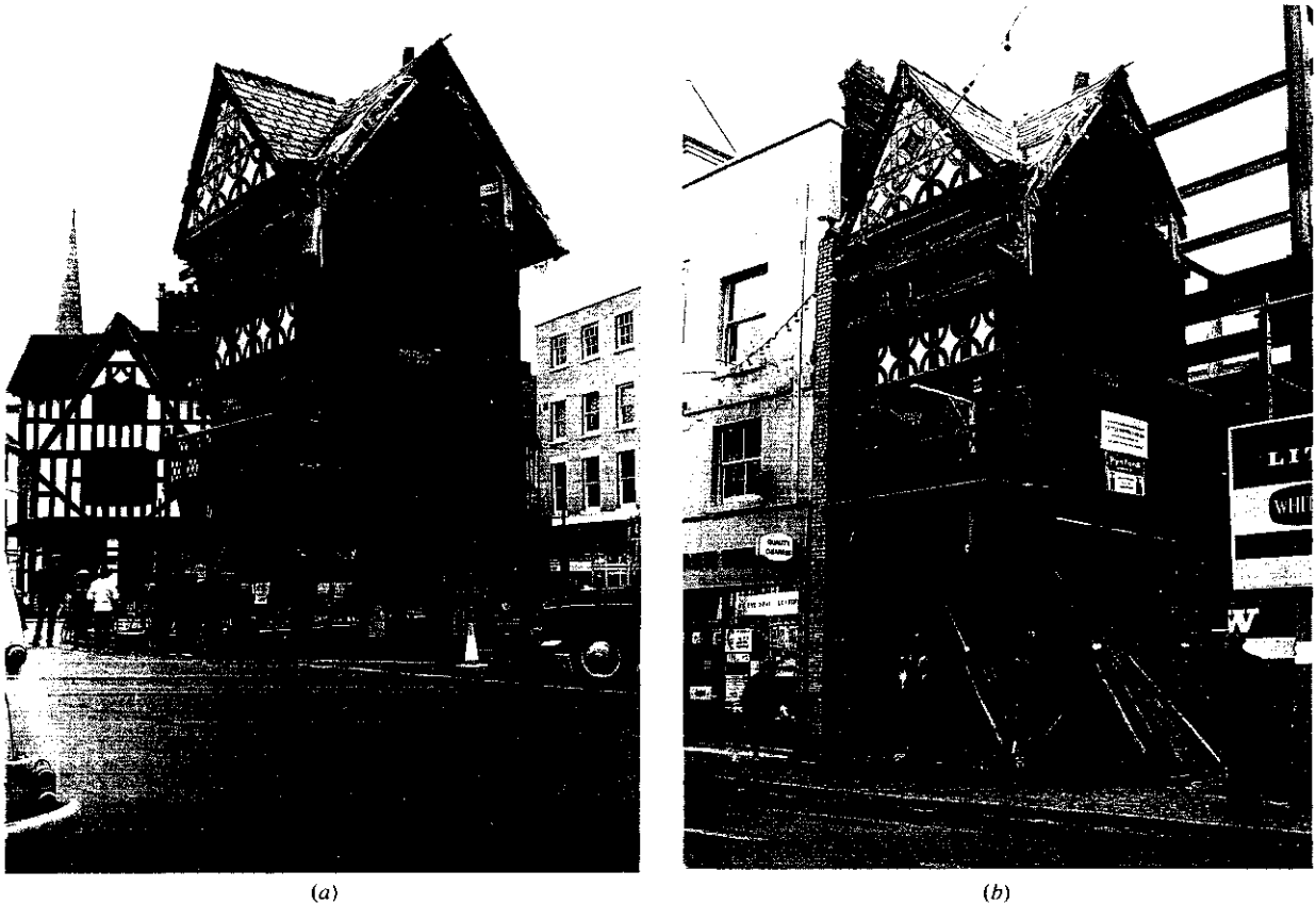
Fig. 12.24 Moving an old building at Hereford. (a) Building supported on a temporary timber chassis before moving to new location. (b) Building being jacked into its final position.
