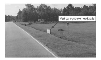
• Do the headwalls need to be this tall? If so, should a reflector of some type be installed to indicate its presence? Should the pipe under the driveway be this size? A drainage study may determine a smaller diameter.
