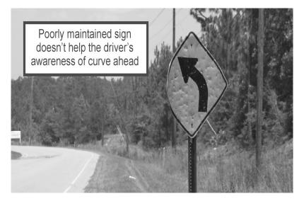
• Include low-cost improvements, like replacing roadway sign that meet M.U.T.C.D current requirements in a project, can vastly enhance the appearance of a project as well aid the driver's decision making. Signs should command respect of the action being advised to the user.
