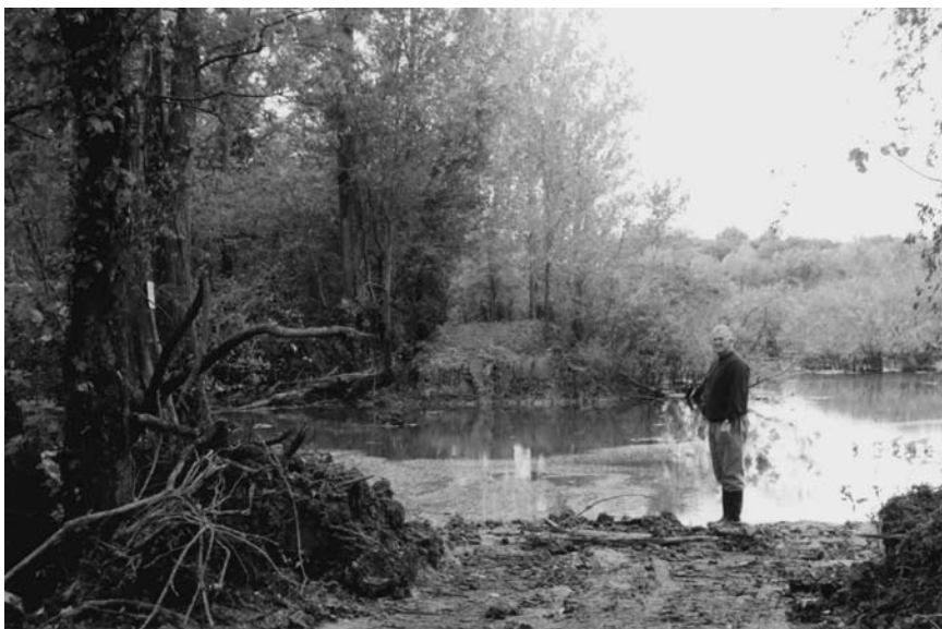
Figure 7-11. Breached levee, Brushy Lake Mitigation Site, Arkansas Department of Transportation, Arkansas. Henry Langston pictured. (Photograph by Phillip Moore; used by permission.)
