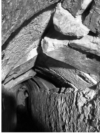
FIGURE 5.17 The support masonry lining between Ch. 178 and Ch. 183 before the intervention.
