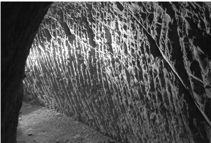
FIGURE 11.19 Excavation traces on the side wall of an unfinished secondary tunnel.
