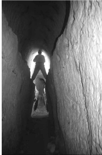
FIGURE 11.13 Errors in height calculation: Above, the tunnel that was laid too high.
