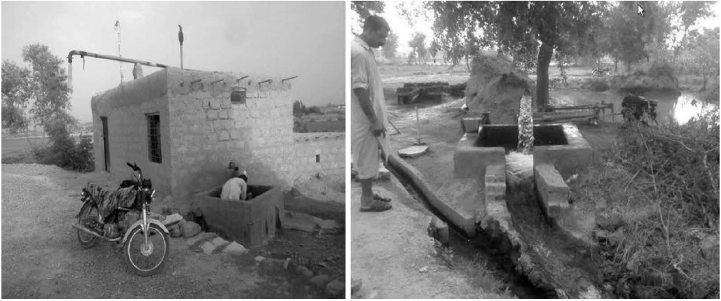
FIGURE 25.14 Modern structure of tube wells in Balochistan. (From GoP, The irrigation and power department, Balochistan, 2013, http://www.balochistan.gov.pk/index.php?option=com_content&view=category&id=1093&Itemid=65 . With Permission.)
