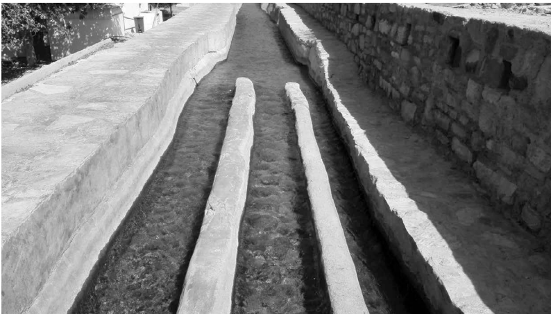
FIGURE 12.1 Water divider of Falaj Al-Khatmeen: It separates the water for the government's benefit from the water for the local farmers' benefit. (Courtesy of Megdiche-Kharrat 2015.)
