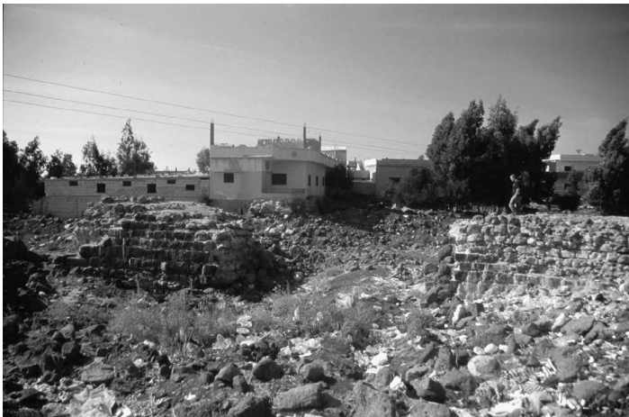
FIGURE 11.5 The west dam made from basalt blocks.
