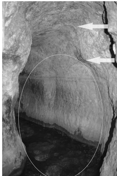
FIGURE 10.3 Tunnel VI at Jerusalem carried water from the Gihon Spring to the bottom of Warren's Shaft (Frumkin and Shimron 2006, 234), and it predated Hezekiah's Tunnel. This tunnel had a hewn barrel-shaped vault ceiling. At a later stage, the ceiling was raised and cut in a square style. (Photography by Frumkin.)
