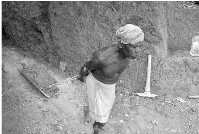
FIGURE 24.3 A suranga under construction.
