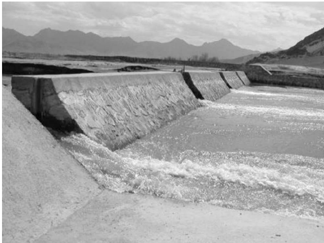
FIGURE 22.5 New dam on the Logar River.
