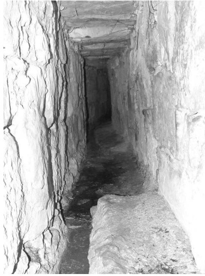
FIGURE 10.10 Naqaa spring. A built spring tunnel from field stones, roofed with stone slabs, and a drainage ditch. (Photography by Yechezkel.)
