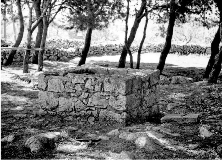
FIGURE 2.17 Shaft no. 7 of Navalja aqueduct tunnel. (From Ilakovac, B. VAMZ , 3.s., XLI, 129–166, 2008. With Permission.)
