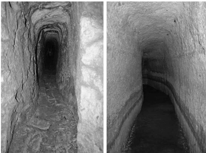
FIGURE 2.15 Navalia aqueduct tunnel. (From Ilakovac, B. VAMZ, 3.s., XLI, 129–166, 2008.)
