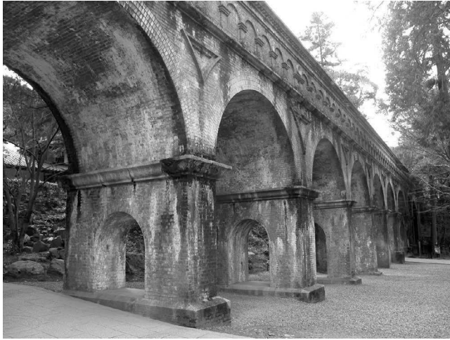
FIGURE 21.15 Brick-masonry arch bridge in Biwako Canal.
