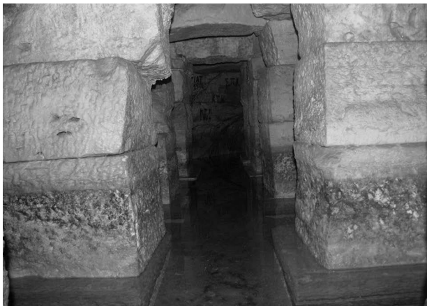
FIGURE 5.3 The interior of the cistern. The mineral and organic deposits on the surface of the pillars indicate the variation of the water level.
