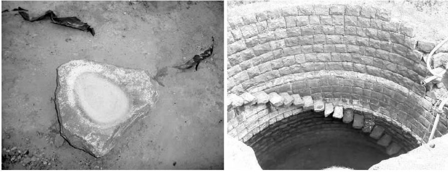
FIGURE 25.7 Storm water storage in rock tank and dry well at Dholavira and Lothal. (From Wales, J., Dholavira, Wikipedia, the free encyclopedia, 2010, http://en.wikipedia.org/wiki/Dholavira#cite_note-frontline-1#cite_note-frontline-1 . With Permission.)
