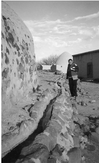
FIGURE 14.3 Author next to an open channel of the qanāt in the village of Shallalah Saghirah. (Reprinted with permission of the photographer J.I. Wessels copyright 2000.)
