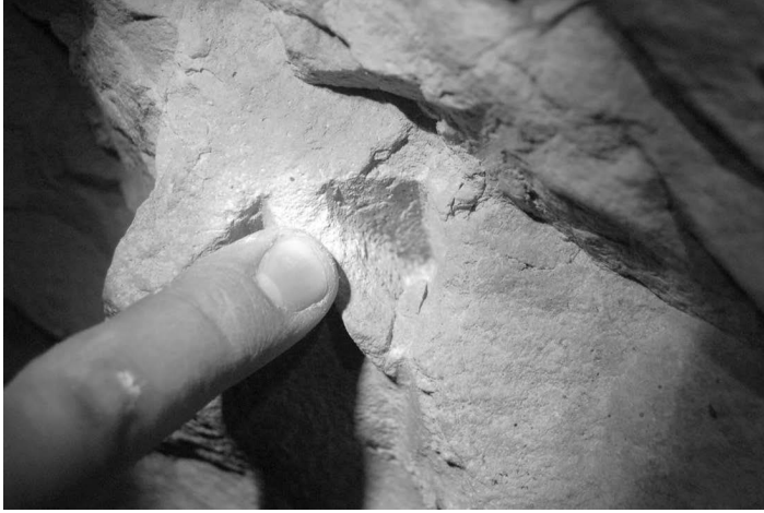
FIGURE 11.18 Mark left by a quadratic moil chisel.
