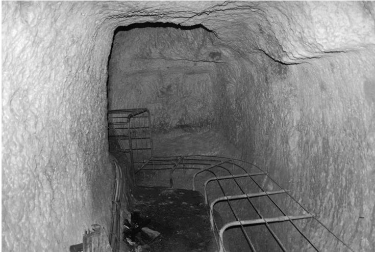
FIGURE 5.9 The south face at the meeting point. The marks of the two miners working side by side are visible. The north bore emerges at the left side of the picture.
