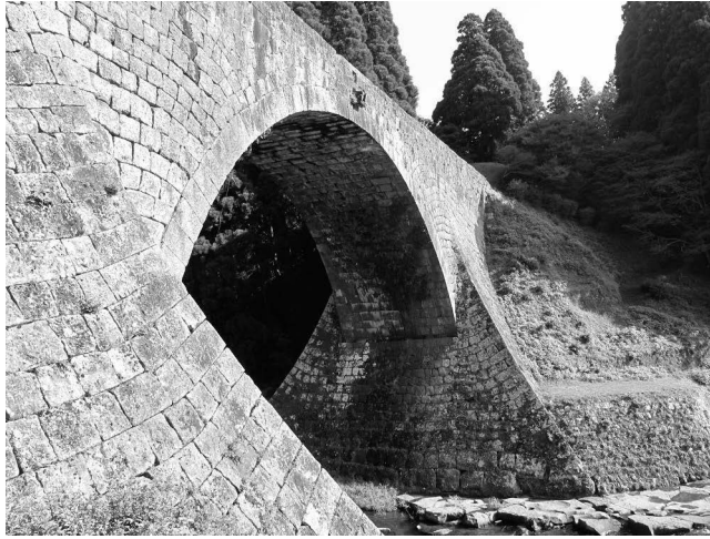
FIGURE 21.12 Tsujun Bridge and arch structure.
