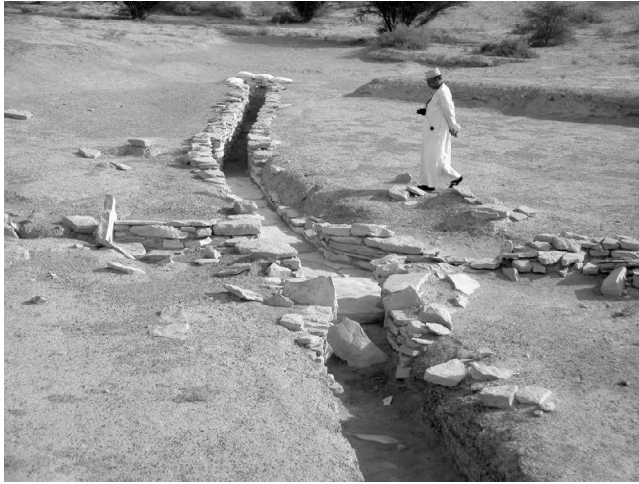
FIGURE 17.3 Falaj Hili 15, Al Ain oasis, Abu Dhabi Emirate, UAE. Water distribution to secondary channels from the outlet of the main channel. (Courtesy of Boucharlat.)
