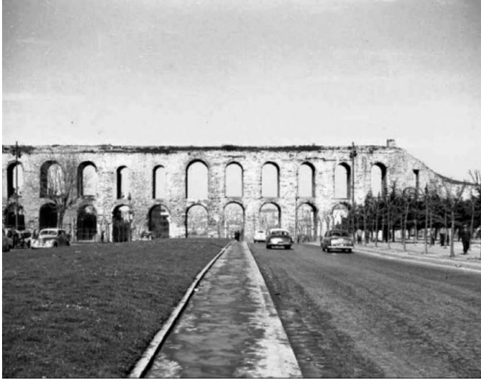
FIGURE 15.7 Bozdoğan (Valens) aqueducts.
