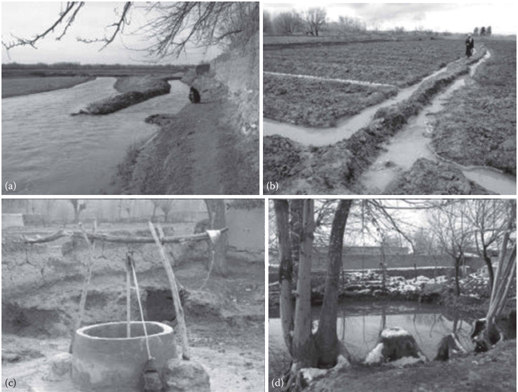
FIGURE 22.4 Typical irrigation facilities in Afghanistan: (a) intake gate in river, (b) earth canals, (c) shallow well, and (d) irrigation pond.
