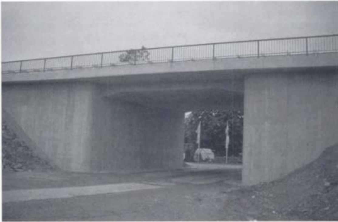
Fig. 2.2 Portal frame bridge
