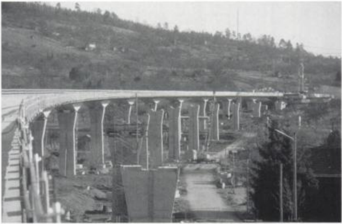
Fig. 2.39 Bridge during construction
