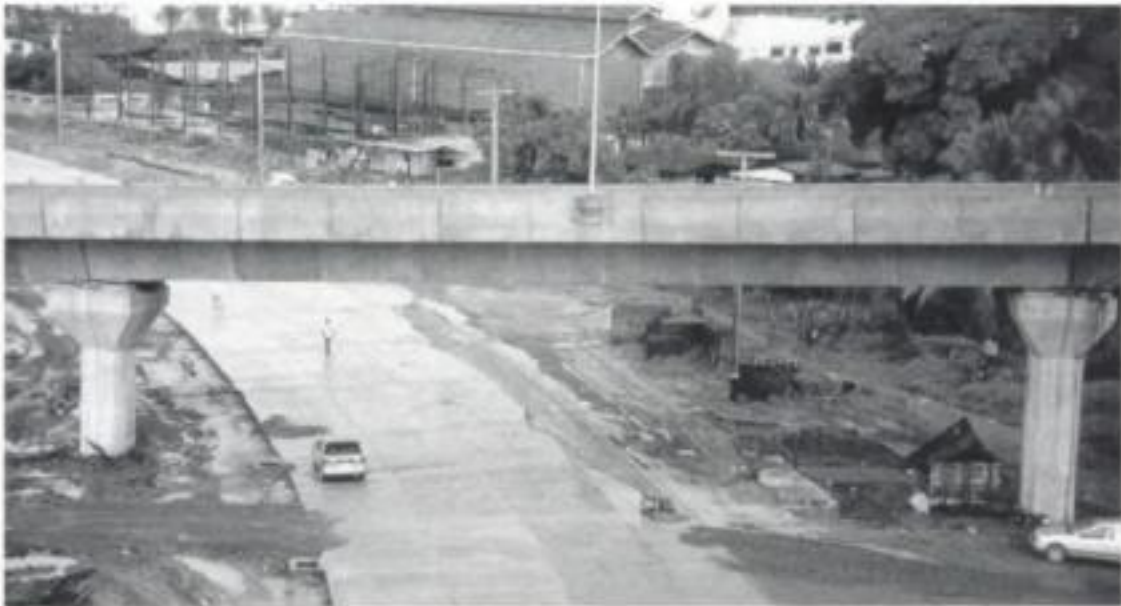
Fig. 2.6 'Standard' span, Second Stage Expressway, Bangkok [12]
