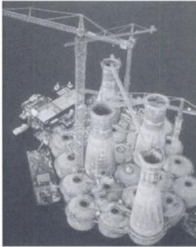
Fig. 1.1 Sleipner A platform (photo NC)
