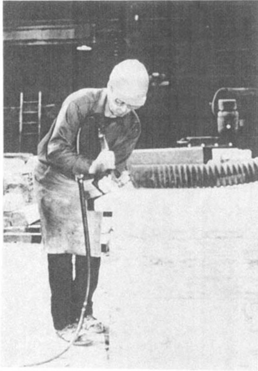
Figure 25.9 Granite cutting with local exhaust ventilation.
