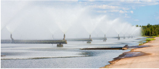
Fig. 18.1 Spray cooling pond
