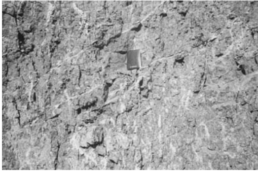
Figure 12.5 A view of the fissures in Ankara Clay.
