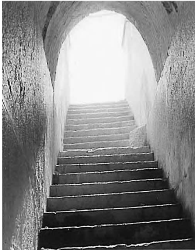
Figure 5.16 Access way to the sewerage networks
