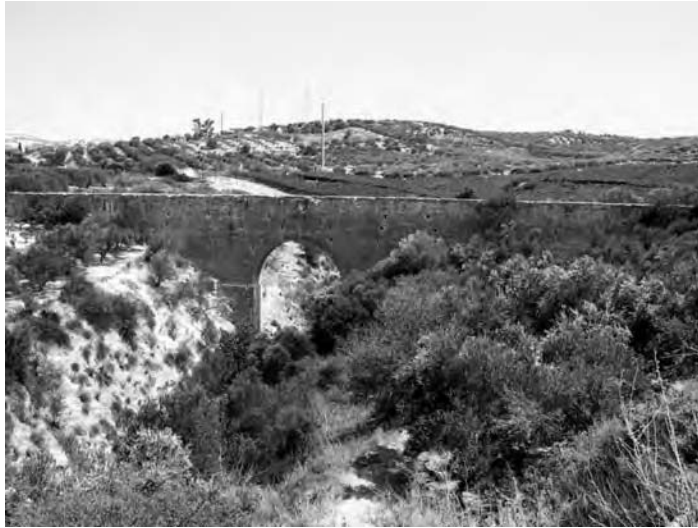
Figure 18.16 The water bridge at Silamos (with permission of N.M. Gigourtakis)
