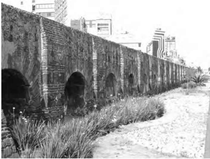
Figure 15.12 Chapultepec aqueduct (also known as the Aqueduct of Belen because of the old Belen convent). Construction of the aqueduct was started in 1620 and completed in 1790, consisting of 904 arches (with permission of Karla S. Estrada Herzfeld)
