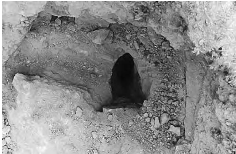
Figure 5.18 Lower segments of the conduits at the sewage outlet
