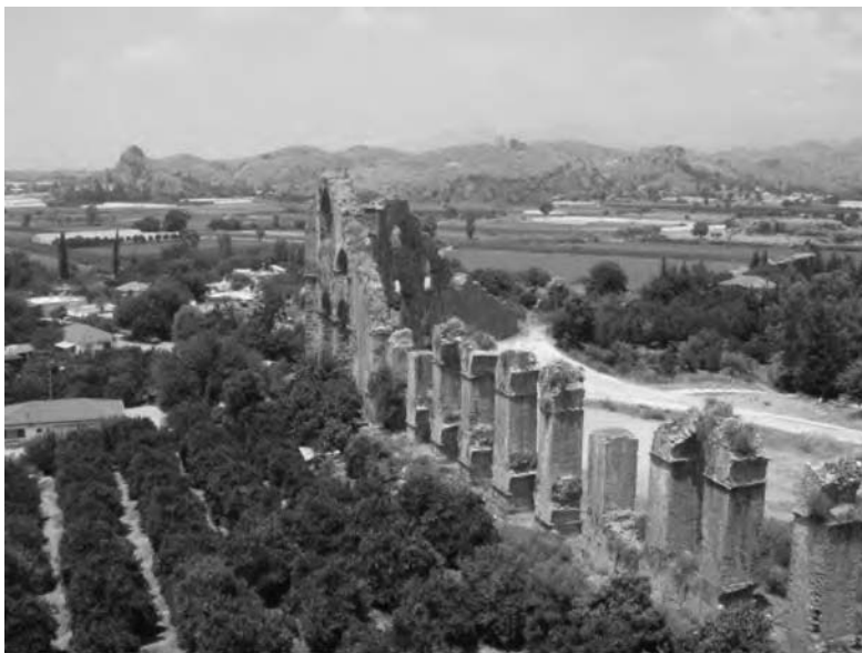
Figure 13.6 Remains of the Aspendos aqueduct (picture taken from the top of the acropolis)
