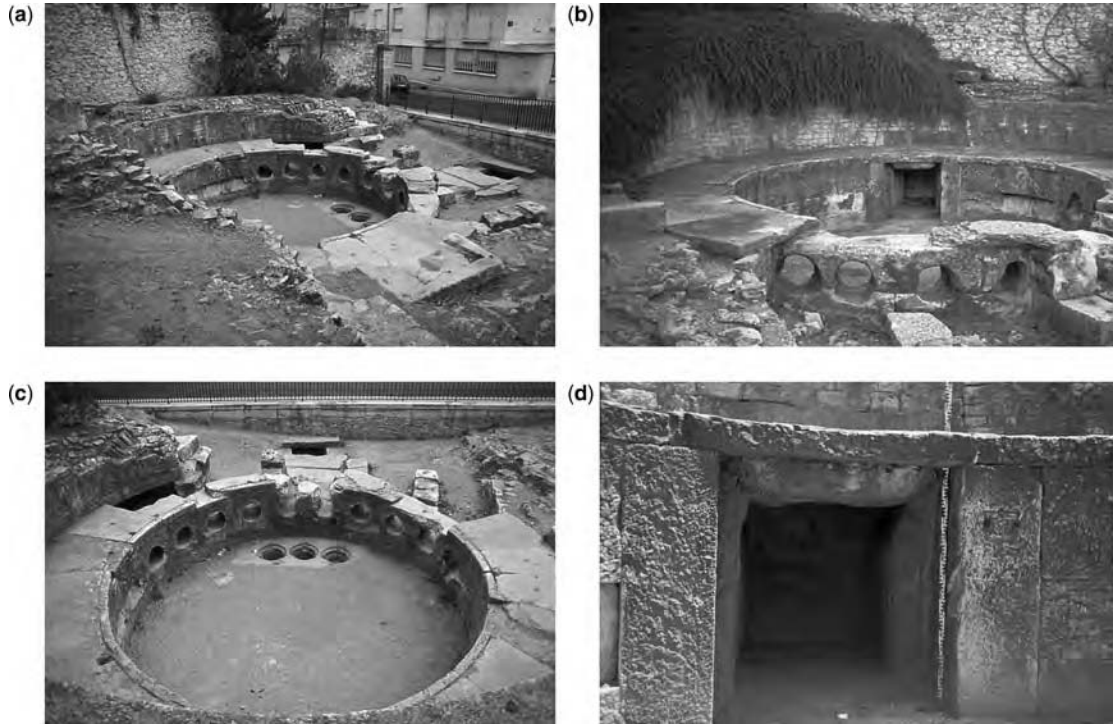
Figure 14.9 Nîmes, remains of the castellum dividiculum : (a) overview over the (10) side openings for (lead) pipes and three bottom openings (with permission of H. Fahlbush); (b) front view (with permission of W. Schram); (c) back view (with permission of H. Fahlbush) and (d) the entrance for the water supply, now closed (with permission of H. Fahlbush)
