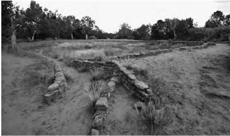
Figure 15.6 Far View Reservoir at Mesa Verde National Park. In the foreground is the restored intake structure (canal) into the reservoir (with permission of L.W. Mays)
