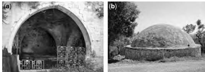
Figure 2.17 Ottoman cistern and fountain: (a) Fountain in Iraklion, Greece and (b) Domed circular cistern in southwest Anatolia (with permission of A. N. Angelakis & L. W. Mays, respectively)
