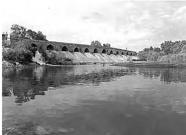
Figure 5.4 Amir multipurpose dam in Fars province (1000 years old)
