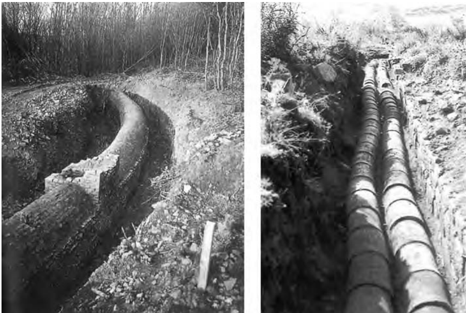
Figure 4.8 Open conduits in Cologne Germany (left). Closed conduits in Pergamos (right) (with permission of G. Karadedos, 2000)
