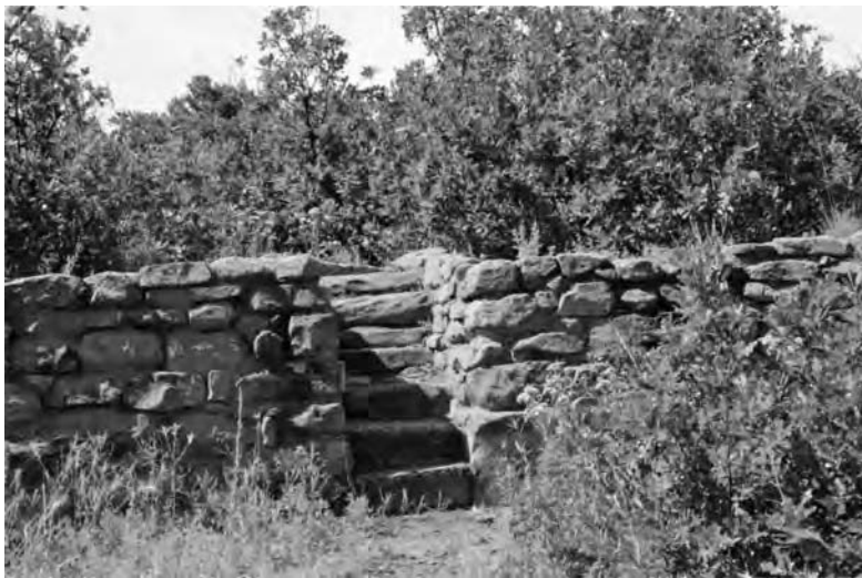
Figure 15.7 Restored stairway at Far View Reservoir in Mesa Verde National Park. Stairway not only functioned as a way to reach the stored water but also may have had special social or religious function (with permission of L.W. Mays)
