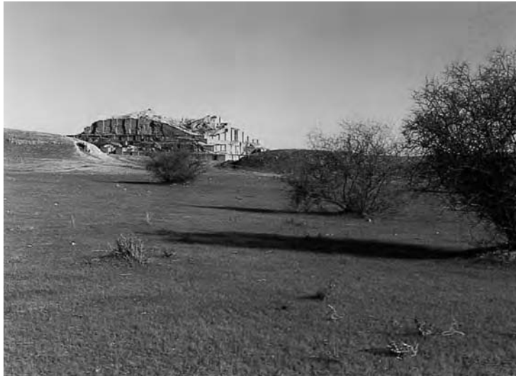
Figure 5.10 Chogha Zanbil Temple enlisted in the list of world culture Heritage by UNESCO
