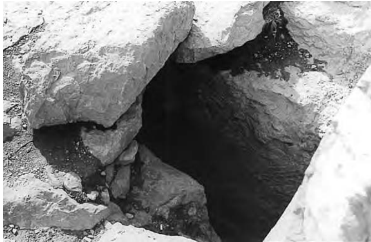
Figure 5.17 Lower segments of the conduits at the sewage outlet
