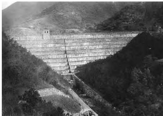
Figure 8.47 Dam (1883–1888) of the Tai Tam Upper Reservoir in Hong Kong (photo of 1907) (Ho Pui Yin, 2001)
