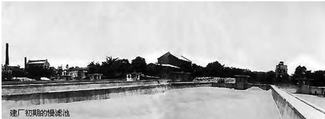
Figure 8.51 Slow sand filter of the 1908 Guangzhou waterworks (Source: http://www.gzwatersupply.com )
