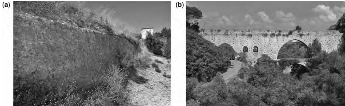
Figure 9.17 Foundana aqueduct: (a) Remnants of aqueduct in Skalani and (b) a water Bridge in Aghia Irini (with permission of M. Nikiforakis, EFIAP)
