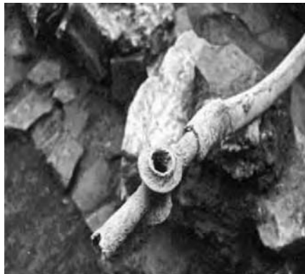
Figure 2.10 Lead water pipe of the Roman period, Greece (Sklivaniotis & Angelakis, 2006)
