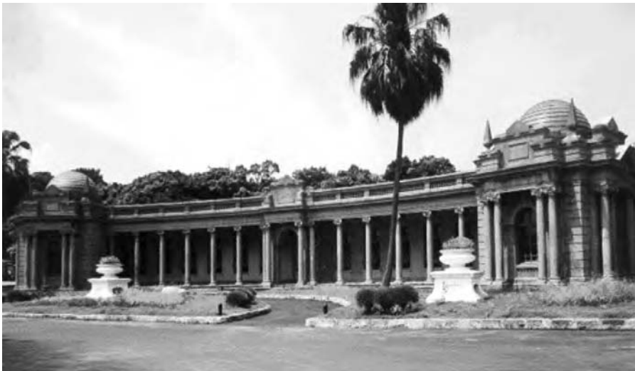
Figure 8.53 Pump Equipment House of Taipei Waterworks of 1908, now Taipei Water Museum ( http://waterpark.twd.gov.tw/english/museum/museum.htm )
