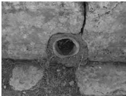
Figure 13.19 Derivation starting from the channel at the centre of Perge's main street
