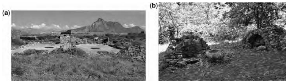
Figure 9.15 (a) Venetian cisterns: on the island of Gramboussa and (b) at the Vamos area (with permission of A.N. Angelakis)
