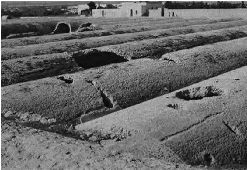
Figure 14.20 Remains of the Roman cisterns (known in French as “ Citernes de la Malga ”) (with permission of A. Bahri)
