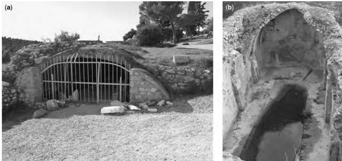
Figure 2.15 Byzantine cisterns in Greece: (a) at the base of the acropolis in Athens and (b) at the castle of Leontari village in Peloponnesos (with permission of L. W. Mays & G. Antoniou, respectively)
