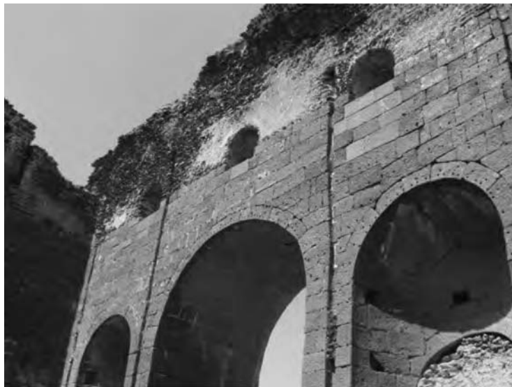
Figure 13.33 Philippopolis baths. Notches can be observed on the room walls
