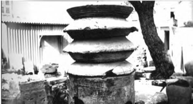
Figure 2.12 Cylindrical terracotta rings, for coating the walls of a Roman well (Sklivaniotis & Angelakis, 2006)
