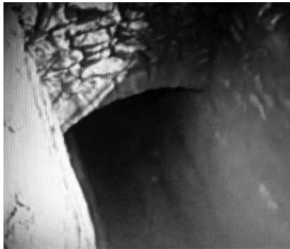
Figure 18.17 The shaft in the underground aqueduct constructed under Morosini's orders (with permission of E.G. Chalkiadakis)
