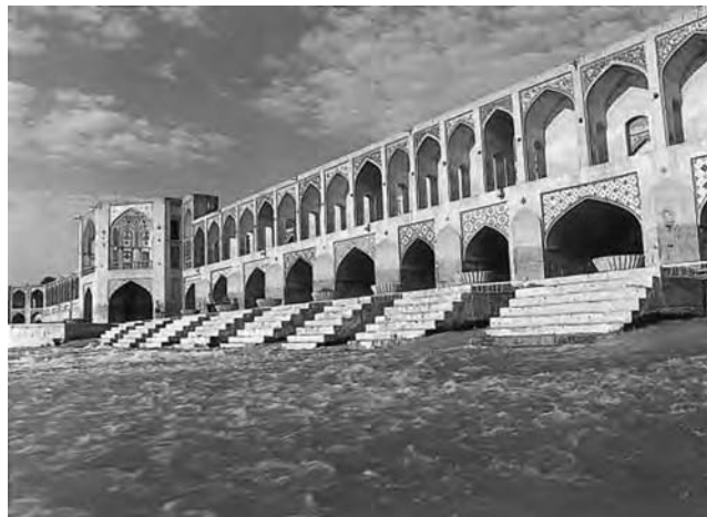
Figure 5.5 Khaju Bridge and diversion dam in Esfahan province (354 years old)
