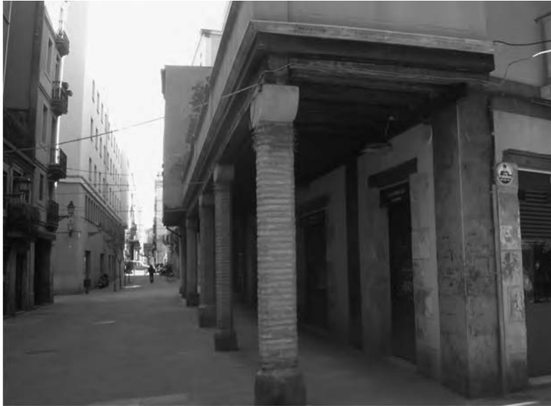
Figure 19.4 The del Rec Comtal street underneath of which the Rec Comtal is flowing (with permission of M. Salgot)
