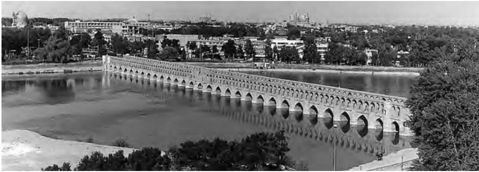
Figure 5.6 Thirty-three Arch bridge in Isfahan province (398 years old)
