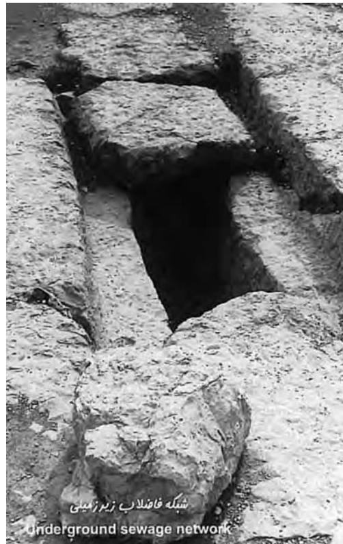
Figure 5.15 Underground sewerage networks
