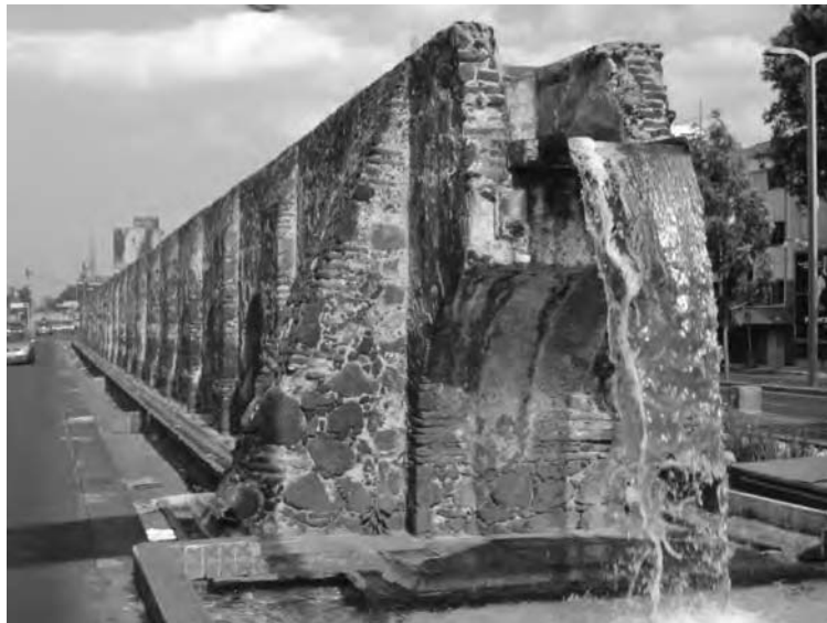
Figure 15.13 Chapultepec aqueduct. Construction of the aqueduct was started in 1620 and completed in 1790, consisting of 904 arches (with permission of Karla S. Estrada Herzfeld)
