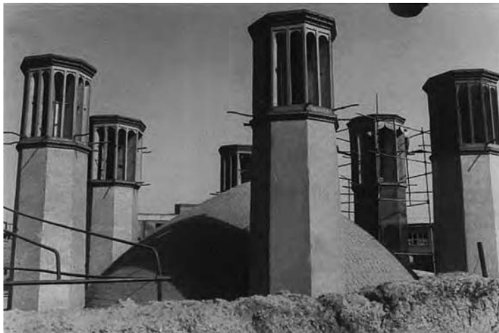
Figure 5.21 Shesh Badgir subterranean water reservoirs in Yazd province with a volume of 2000 m 3
