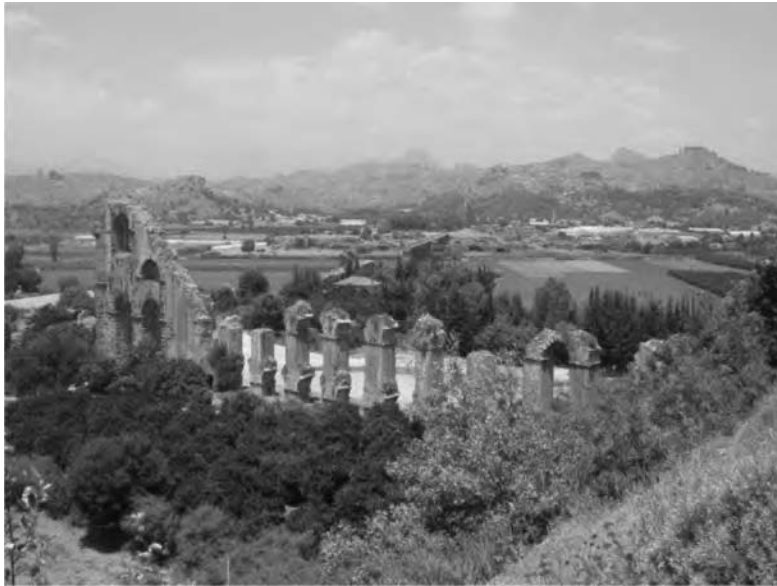
Figure 13.5 Remains of the Aspendos aqueduct (picture taken from the top of the acropolis)
