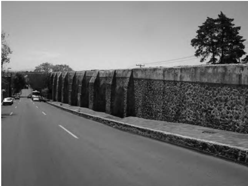
Figure 15.15 Queretaro Aqueduct, Mexico (with permission of Karla S. Estrada Herzfeld)
