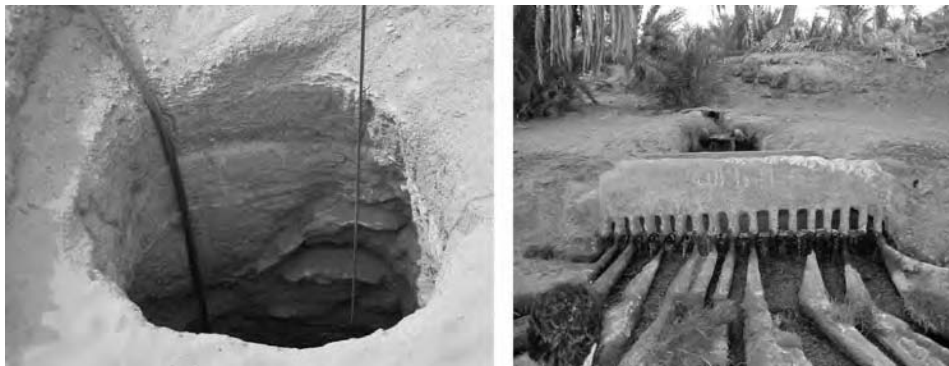
Figure 2.1 A foggara at Adrar, Algeria: (left) shaft; (right) distribution and metering weir at the foggara outlet (Mays et al. 2007)
