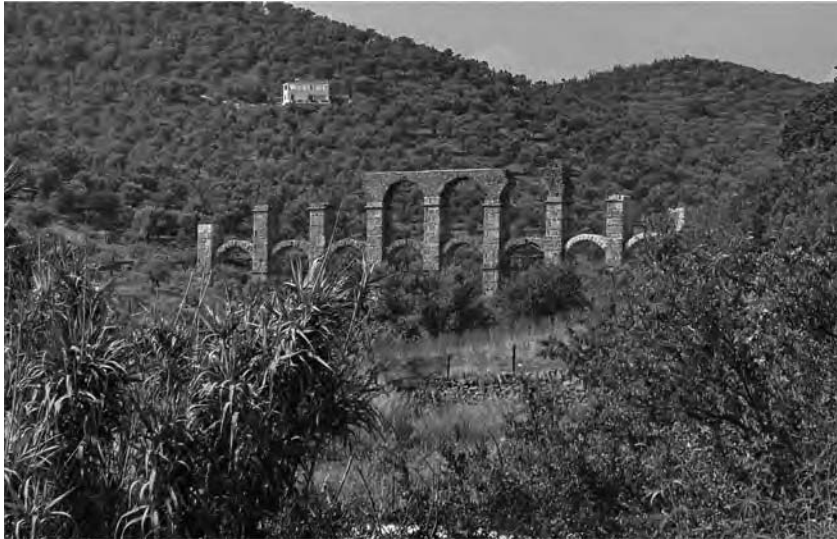
Figure 14.11 Part of the impressive Roman aqueduct rises 600 m west of Moria, a Lesvian village 6 km from Mytilene town (with permission of A. N. Angelakis)
