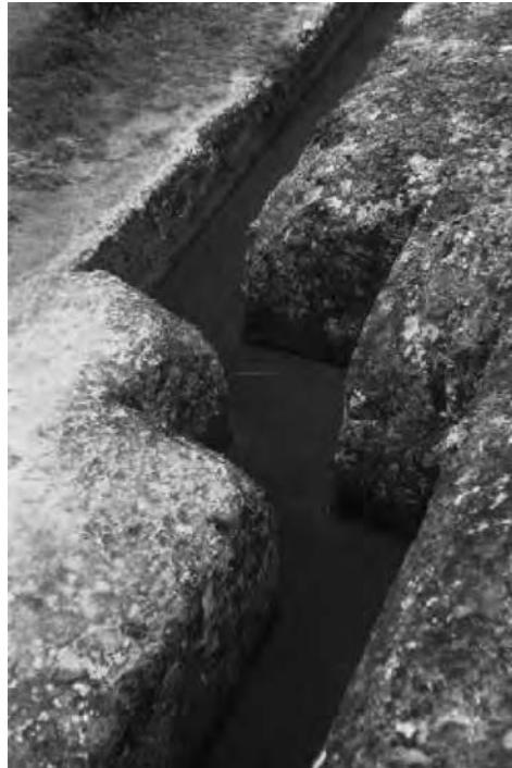
Figure 11.7 Detailed view of the first section of the Cumbe Mayo aqueduct carved on volcanic rock
