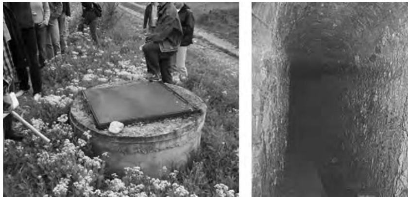
Figure 4.10 Left: The initial well (shaft) of a qanat in Nea Zichni (with permission of K. Voudouris). Right: The tunnel of a qanat at Chortiati, Thessaloniki constructed in the 18th century (with permission of K. Voudouris)
