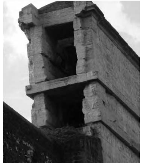
Figure 17.10 Porta Maggiore: superimposed conduits with Anius Novus at the top (photo by R. Drusiani)
