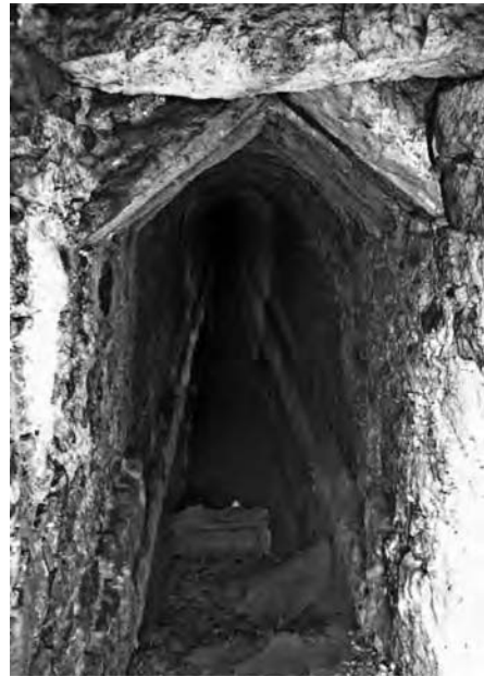
Figure 18.4 The Roman aqueduct supplying water to Knossos from the Fundana spring (with permission of N.M. Gigourtakis)
