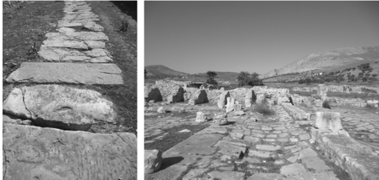
Figure 13.19 General view of slabs used to lay the street and cover the drainage canals and sewage network at Bulla Regia . The partially degraded cement between slabs let show the sewer beneath (left). Sometimes the slabs collapse or are deformed causing deformation of the street (with permission of O. Mahjoub).
