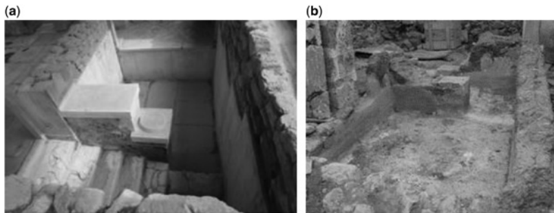
Figure 1.9 Bathrooms: (a) In the King's Megaron at Phaistos and (b) in the Da House at Malia (with permission of A. N. Angelakis).
