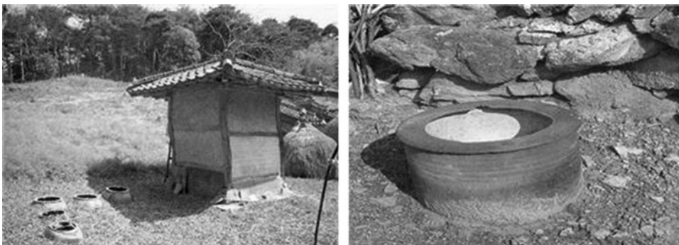
Figure 14.7 Pit latrine toilet (left) and urine jar (right) for excreta collection and storage (Kim, 2002).
