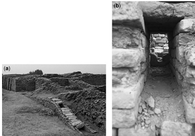
Figure 24.2 Drains in Mohenjo-Daro: (a) Covered drain emptying down slope on major street and (b) close-up view of ground floor drain outlet from the street side ( http://www.mohenjodaro.net/index.html ).
