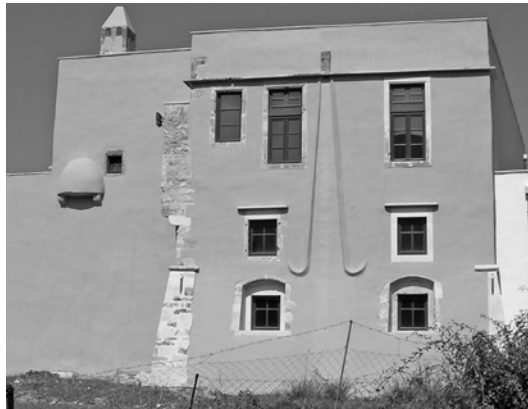
Figure 6.39 Protruding lavatory at the 2nd floor of a rural residential complex in Chromonastiri on Crete (with permission by G. Antoniou).
