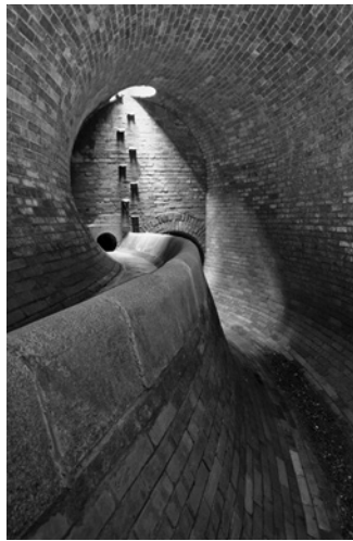
Figure 20.2 Combined sewer overflow chamber Vltavska.
