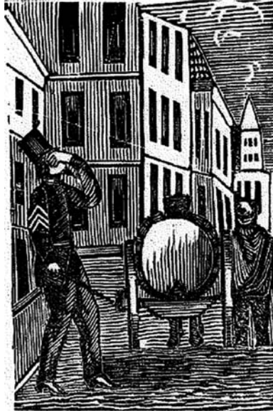
Figure 19.5 Cart used to empty cesspools. Los perfumes de Barcelona (Barcelona scents), 1875.
