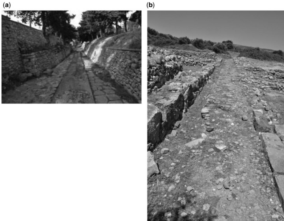
Figure 1.13 Drains in central roads: (a) The 'Royal Road' known as the 'oldest road in Europe' in the palace of Knossos and (b) at Palekastro town (with permission of A. N. Angelakis).
