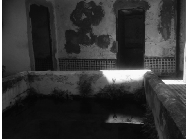
Figure 11.22 Basin of spring resurgence in the Mosque ‘Ayn Azlitan’. Latrines are supplied by the basin (with permission of H. Benqlilou).
