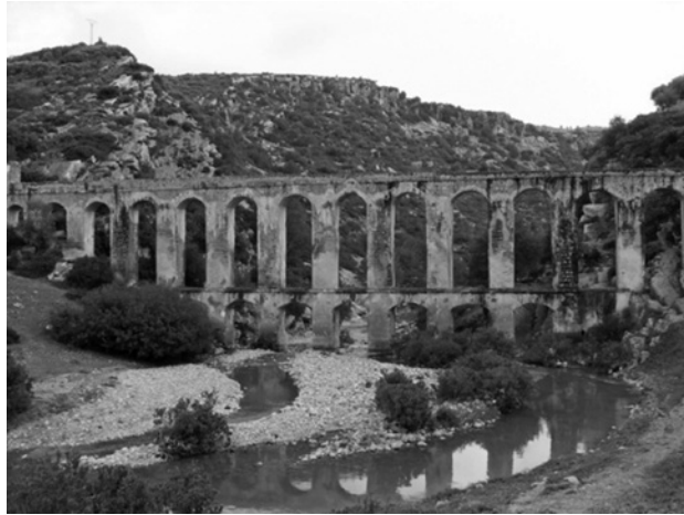
Figure 11.13 Aqueduct constructed by Idriss 1 (with permission of M. Atki). Source: Conservation of the archaeological site of Volubilis.
