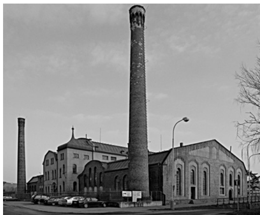
Figure 20.4 Old Lindley's WWTP in Prague.
