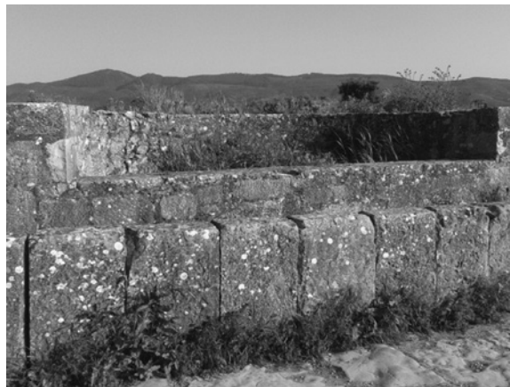
Figure 11.7 Public fountain in two floors (with permission of H. Benqilou).
