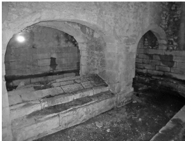
Figure 10.10 The wastewater Treatment Plant in Tomar monastery.
