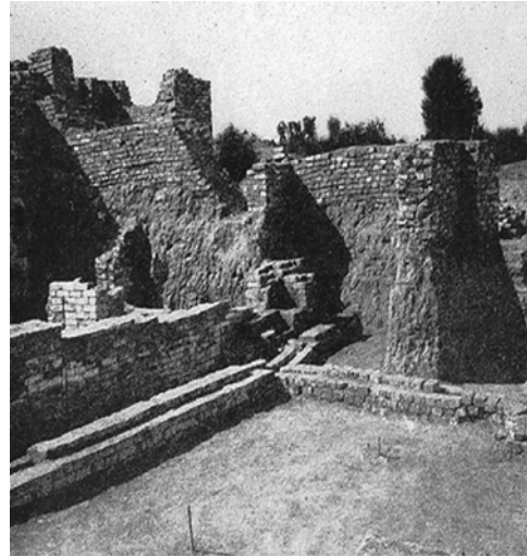
Figure 4.3 Harappan above ground sewer channel constructed of burnt brick (Kirby et al. , 1956).
