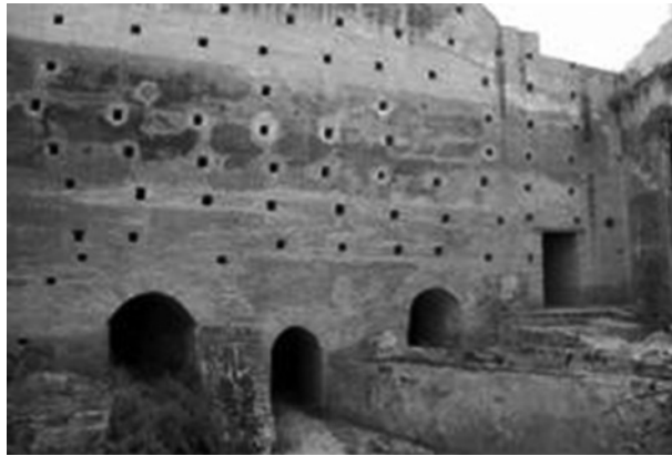
Figure 11.14 Main water splitter located in Bab Boujloud, one of the city gates (with permission of F. Serghini, ADER–FEZ).
