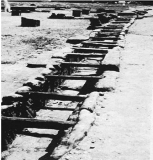
Figure 4.2 Mohenjo-Daro excavated sewer channel (Hodge,1992).
