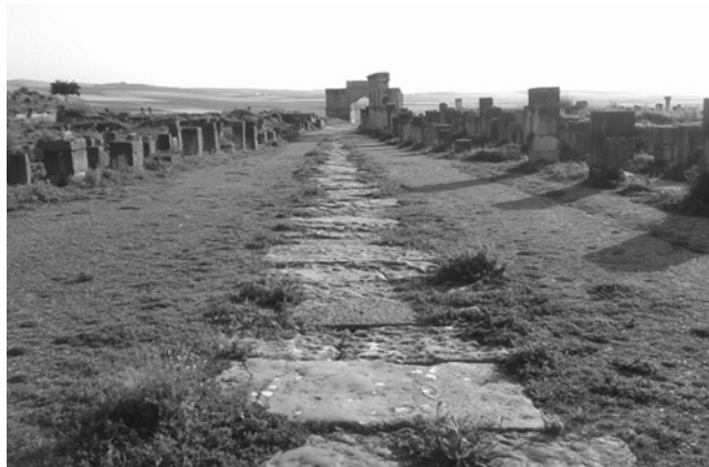
Figure 11.4 Main wastewater and stormwater sewer (with permission of H. Benqlilou).
