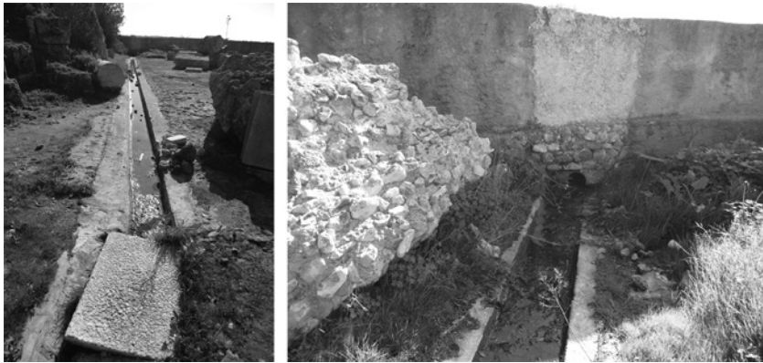
Figure 13.11 Drain canals carrying the water through the bath rooms toward to the sea (with permission of O. Mahjoub).
