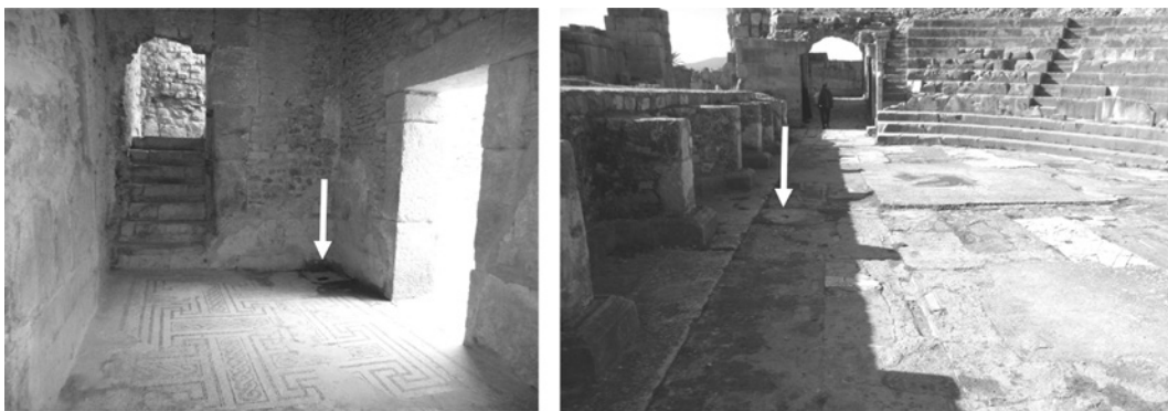
Figure 13.16 Openings of the underground canals (white arrows) on the right corner to collect water used for cleaning at the House of Amphitrite (left) and orchestra opening drain in the amphitheatre at Bulla Regia (right) (with permission of O. Mahjoub).
