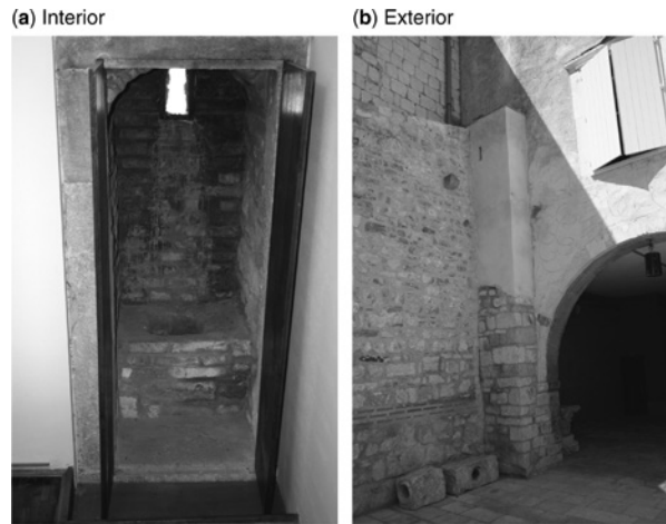
Figure 16.12 Toilet in a Romanesque house in the Diocletian's Palace with direct drainage into the Roman substructure.
