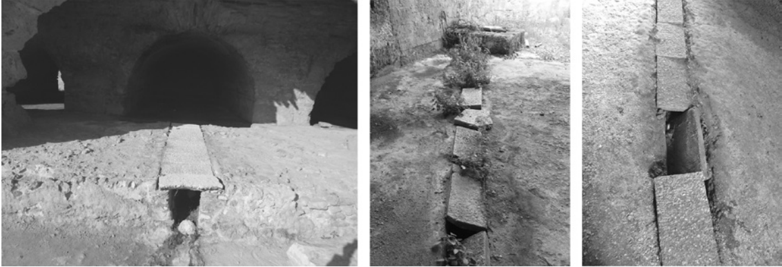
Figure 13.9 View of the hypocaust in basement of the Antonine baths. Canals are covered with pieces of stones. When following these canals upward the slope, a kind of cistern is found upstream. These canals may have been used to carry hot water (with permission of O. Mahjoub).
