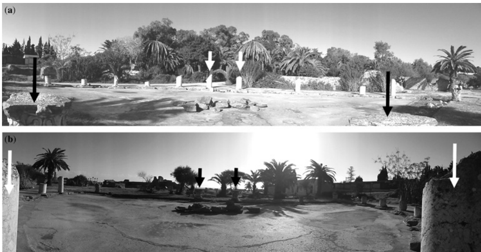
Figure 13.12 (a–b) Panoramic views of the public latrines built next to the south west portico of the Antonine baths. The latrines are hemicycle shaped with 35 m of diameter. Parts of the broken wash basin, in front of the seats, are visible in the centre. Arrows of same colour are used to indicate the same columns on both photos (with permission of O. Mahjoub).
