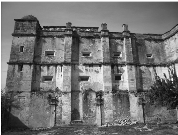
Figure 10.8 The 'Bloco das Necessarias' in Tomar containing latrines and the WWTP.
