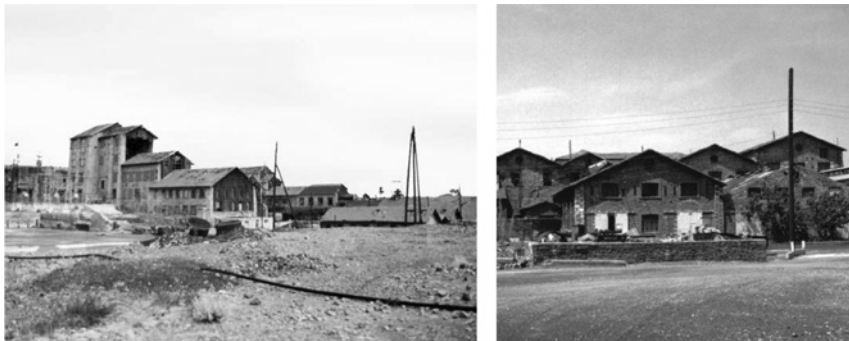
Figure 25.6 Industrial buildings of the modern era within the Lavrion metallurgical plant.
