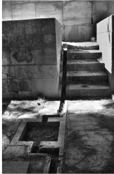
Figure 1.14 Part of restored Minoan stairway with parabolic runnels in the north eastern entrance (with permission of A. N. Angelakis).
