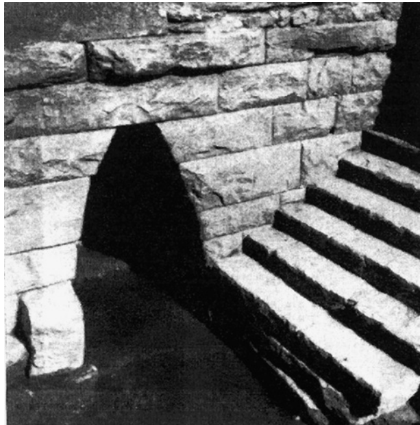
Figure 6.14 Thassos. Drainage opening on city walls (Grandjean, 1994).
