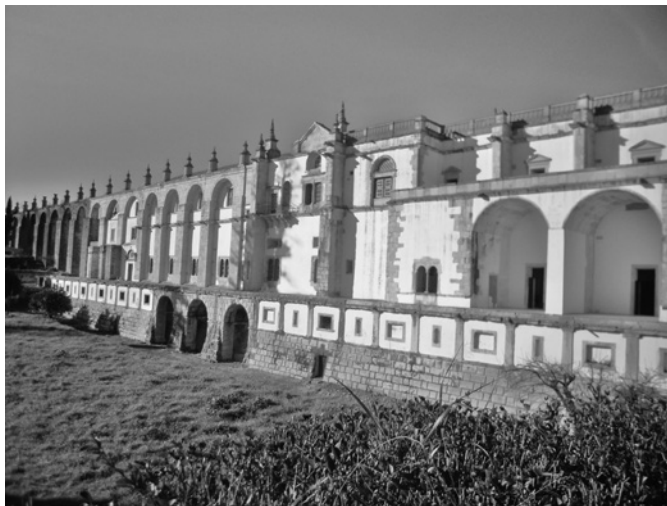
Figure 10.5 Convent aqueduct in Tomar.
