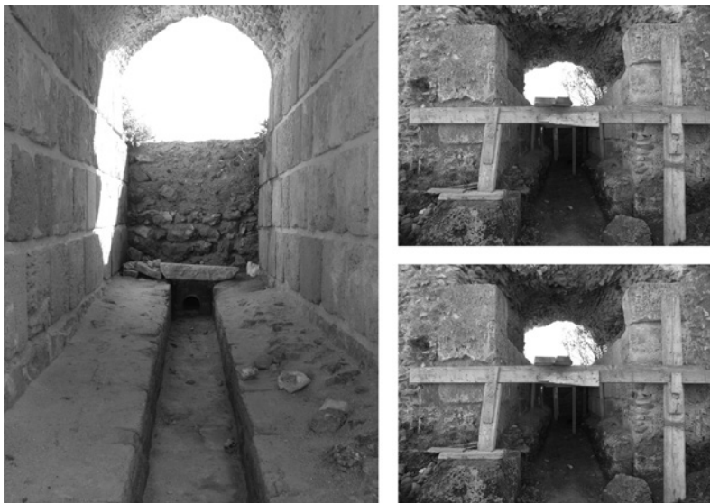
Figure 13.10 View of 2 drains at the Antonine baths, one of them is being restored. The photos are taken toward the sea (with permission of O. Mahjoub).
