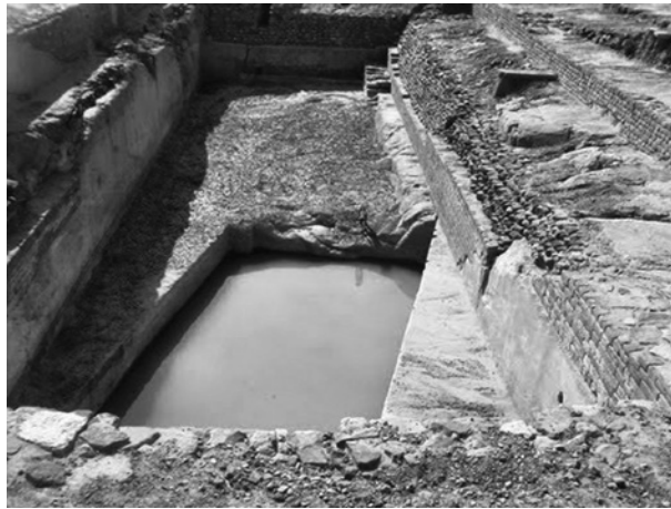
Figure 2.11 Hydraulic Engineering Indus Civilization at Dholavira, Rann at Gujrat (Wales, 2010).
