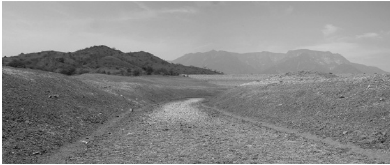
Figure 5.7 View of a section of the pre-Columbian Racarumi intervalley channel ( Mochica , northern coast) normally submerged under the water body of the Tinajones reservoir since 1968. The pre-Columbian channel continues its course behind the earth dam in the picture, placed perpendicular to its axis. The reason why the reservoir was considerably empty could not be ascertained with exactitude. Most likely high water demands for agricultural needs (e.g., Ethanol production) coupled with sporadic water distribution usages of the competent water resources management authorities and/or delay of the replenishing rains at the water source in the nearby Andean Region may have been the reasons. (Picture taken during investigation field works by Reyes-Knoche, November 2011; Reyes C. & Reyes-Knoche, 2012).
