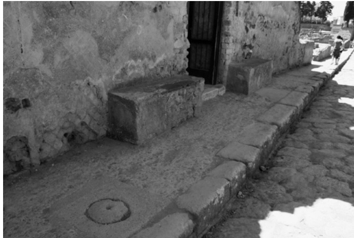
Figure 12.6 Herculaneum, House of the Skeleton ( Insula III, 3, Cardine III inf. ), inspection sump of the conduit used to convey wastewater into the sewer.
