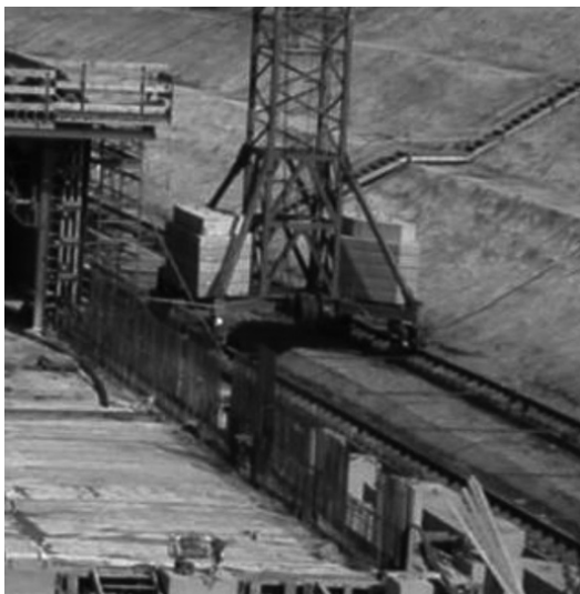
Figure 2.29 Crane runway
