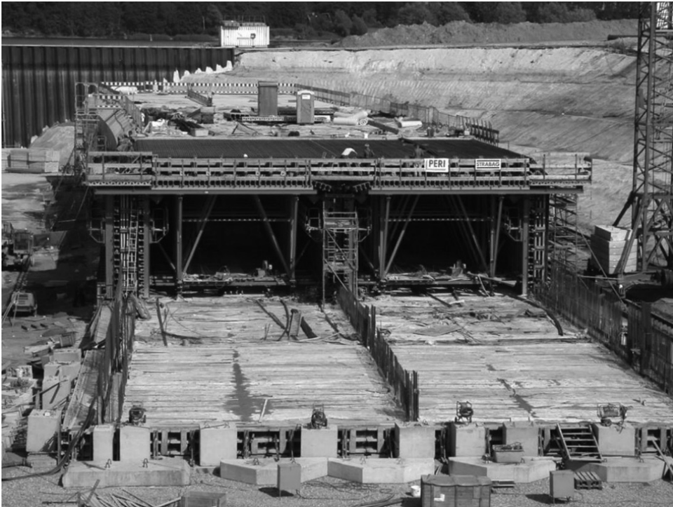
Figure 2.26 Assembly of tunnel segments
