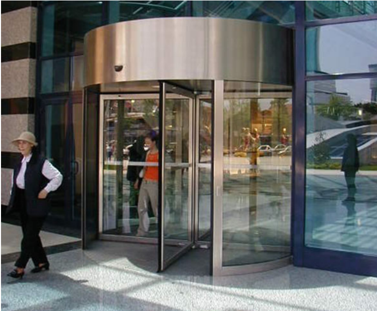
Fig. 1 International revolving door in Turkey. The door adds emphasis to the building entrance. Photo by Moberg/Wikimedia commons. Detail of URL: https://commons.wikimedia.org/wiki/File:Revolving_Door.jpg#/media/File:Revolving_Door.jpg
