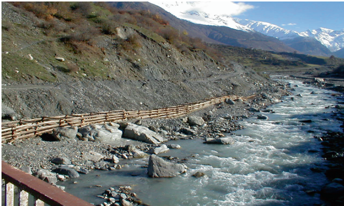
Figure 2. Eroded banks of the R. Mudkhuri near v. Jamushi (Svaneti)
