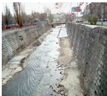
Figure 6. The riverbed of the Getar River in an open section
