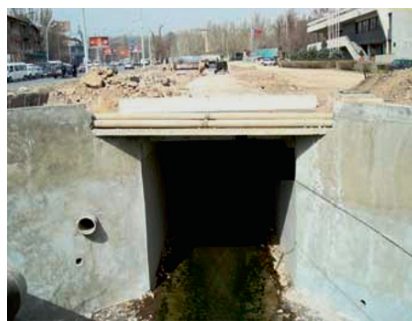
Figure 7. Covered section of the riverbed of the Getar River
