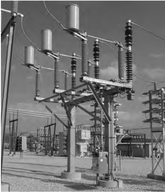
Figure 22.20 Mark V three-phase circuit switcher for capacitor applications. (Courtesy of S&C Electric Company, Chicago.)
