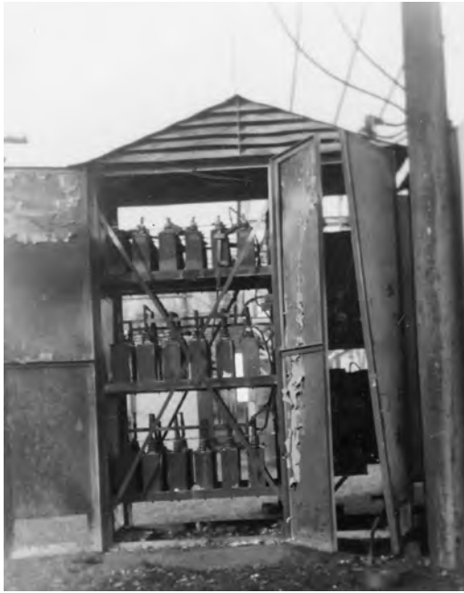
Figure 19.3 A failed capacitor bank due to fire. (Courtesy of Duke Energy, Charlotte, NC.)
