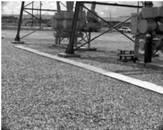
Figure 23.16 Control wire conduit in a substation location. (Courtesy of U.S. Department of Labor, OSHA website, Reference [5].)
