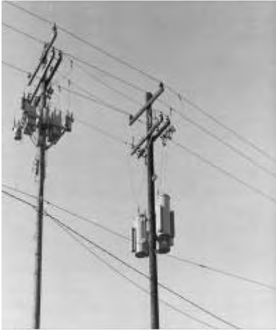
Figure 7.4 A pole-mounted harmonic filter bank. (Courtesy of Gilbert Electrical Systems and Products, Beckley, WV.)
