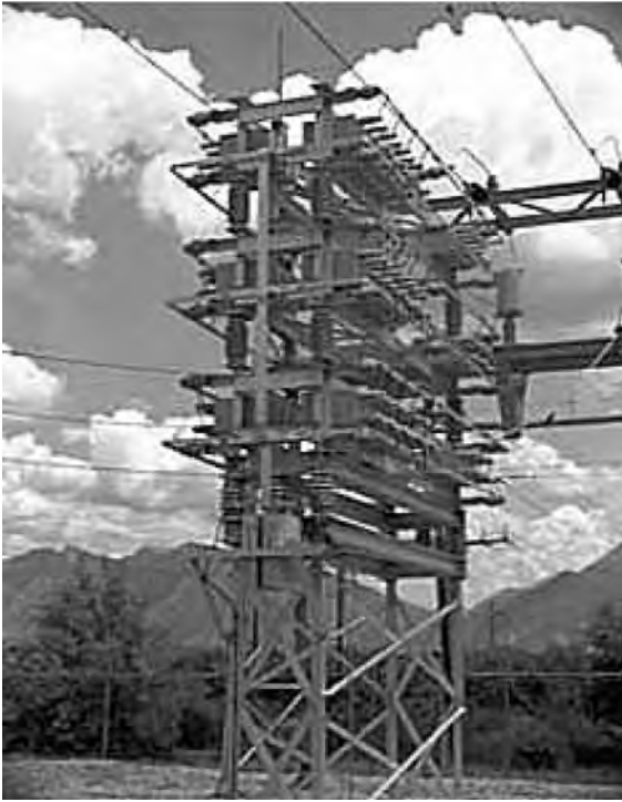
Figure 7.6 Substation capacitor bank. (Courtesy of U.S. Department of Labor, OSHA website.)
