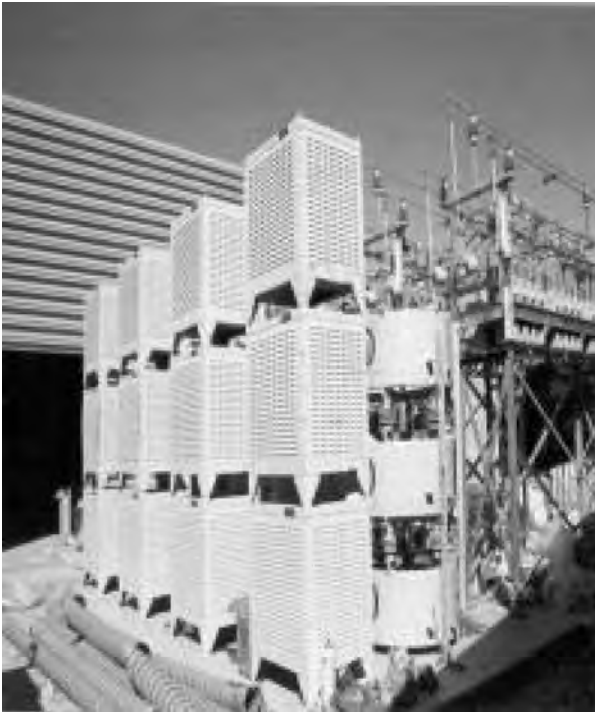
Figure 7.5 A high voltage filter bank. (Courtesy of Gilbert Electrical Systems and Products, Beckley, WV.)
