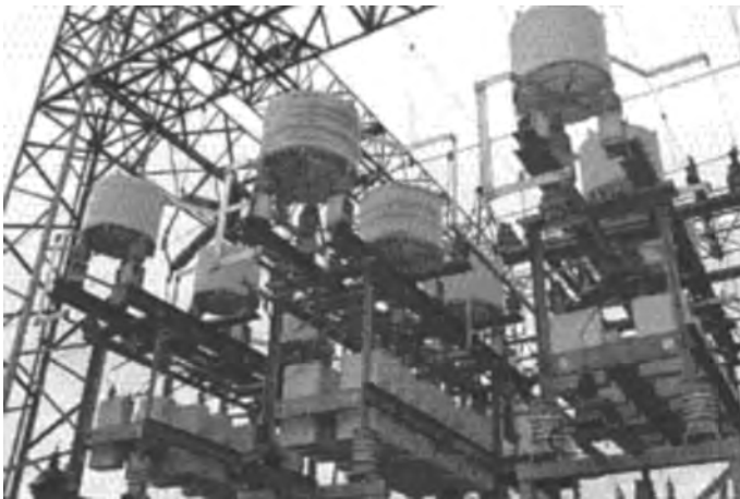
Figure 20.13 A typical filter installation at a chemical factory. (Courtesy of IEEE, Reproduced from Reference [8].)
