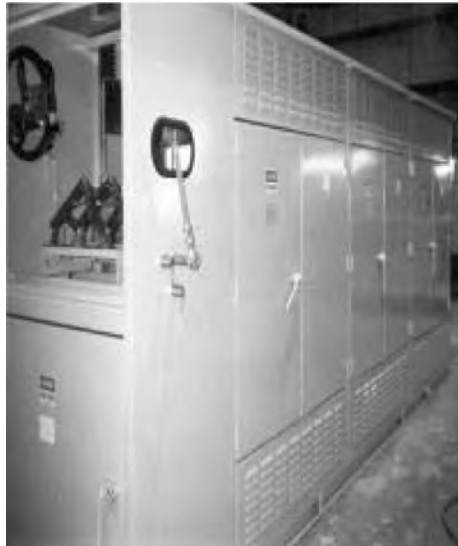
Figure 7.7 A metal-enclosed harmonic filter bank. (Courtesy of Gilbert Electrical Systems and Products, Beckley, WV.)
