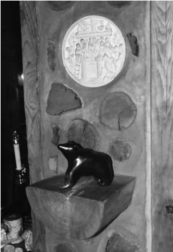
9.5: This small display shelf is a 24-inch-long half-round log-end extending 8 inches out from the 16-inch cordwood wall. Above the shelf, an inch-thick replica of a 14 th -century ivory carving is backed by a shortened (15-inch) log-end of the same diameter.
