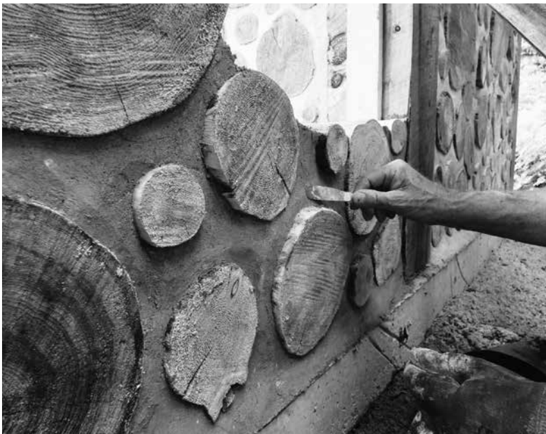
8.22: I draw the knife along the mortar joint with a fairly quick motion and with some pressure, smoothening the mortar. I take my glove off my pointing hand only, for better “feel” of the knife, but I am careful not to touch the mortar. Jaki points beautifully with her glove on.
