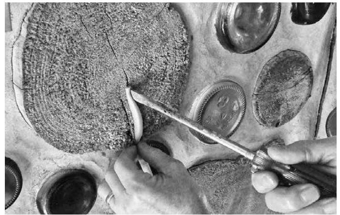
10.2: Push backer rod into the check with a flathead screwdriver.
