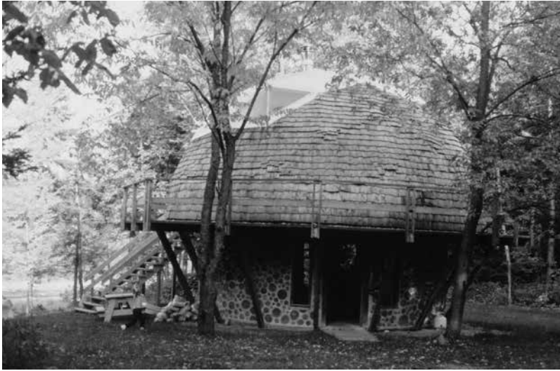
6.5: We built the first story of our 22-foot diameter Mushwood Cottage under a 29-foot diameter geodesic dome, then re-erected the dome at the second level and lived in the mushroom-shaped cottage for 25 years.
