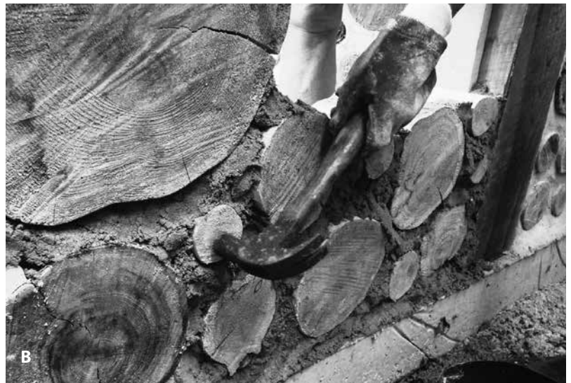
8.15: (A) The author eyeballs from post to post in search of errant log-ends. He spots a small one sticking out too far. (B) The sharp impact of a hammer will allow log-ends to be brought back into line.
