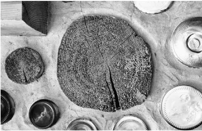
10.1: A large primary check needs to be filled.
