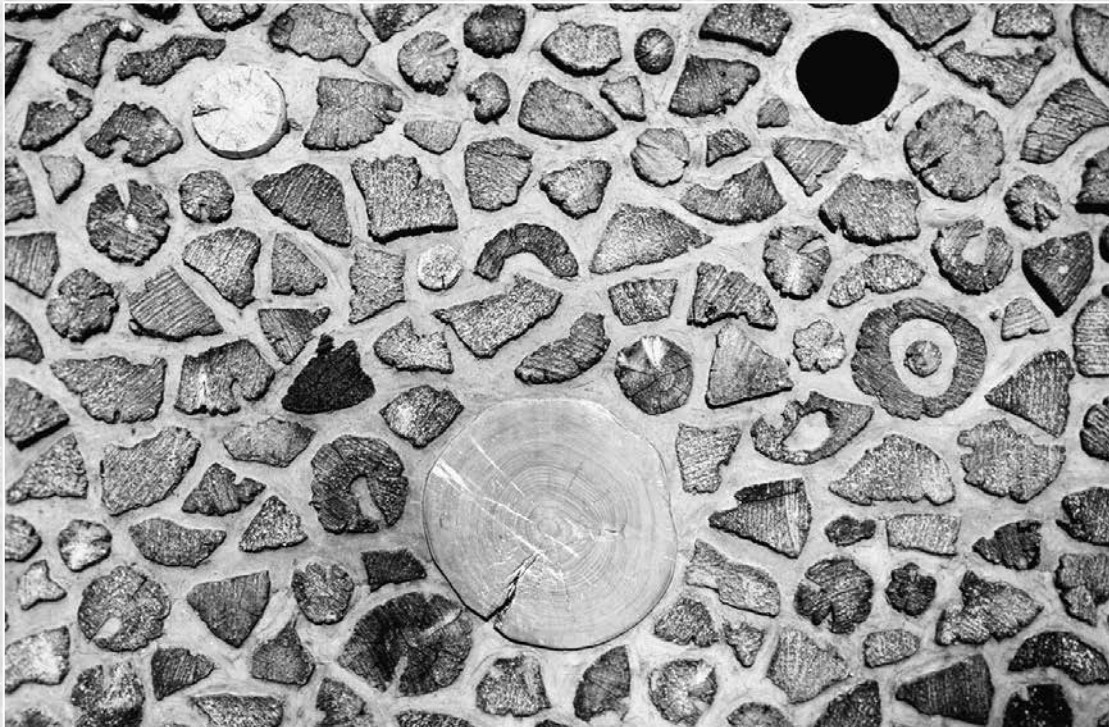
5.11: Our Log End Sauna walls were mixed rounds and old split cedar fence rails. The large log-end was a varnished elm. It stayed nice for over 30 years on the inside, but the sun's UV rays wore the varnish off on the exterior within a year or two. The two rounds at the top had handles on the inside and could be removed for ventilation.
