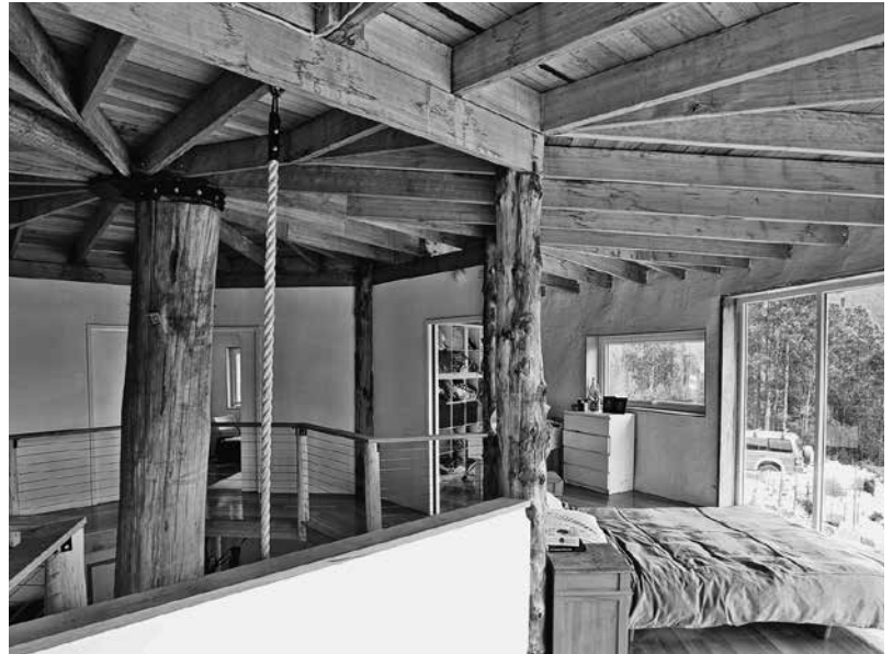
9.18: The cordwood masonry is covered with plaster rendering.
