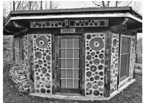
6.21: Stoneview is an octagonal guesthouse with eight 8-inch by 8-inch girts joined over eight special posts. Both the door jambs and the long window frames (all 4-inch by 8-inch stock) extend from the floating slab to the underside of the girts. Full framing details are in my book Stoneview: How to Build an Eco-friendly Little Guesthouse (New Society Publishers, 2008).
