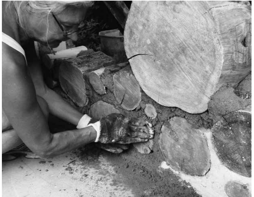
8.20: Jaki rough points the wall, using just her rubber gloves, assuring that the “reveal” will be the same throughout the panel, about a quarter inch.
