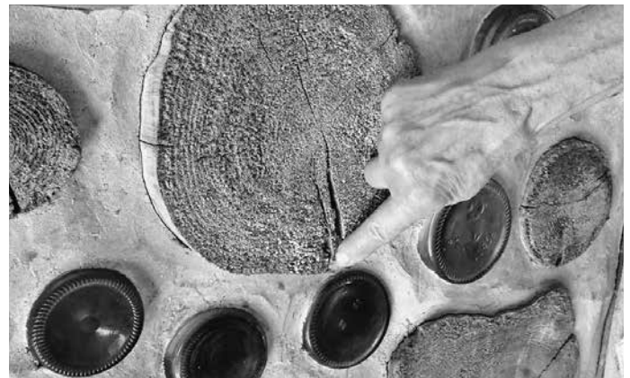
10.4: Jaki seals the caulk with her finger. The end result looks very much like a round log with a check in it. In fact, it looks exactly like Figure 10.1.
