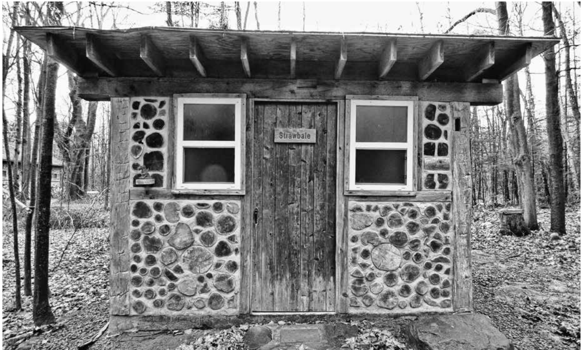
6.19: Strawbale (and cordwood) guest house at Earthwood. The door is exactly framed by the 4-inch by 8-inch jambs which extend from the foundation to the 8-inch by 8-inch girt.
