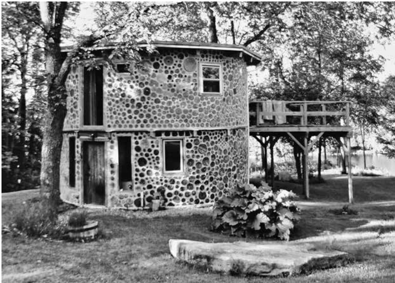
6.6: When the dome began to deteriorate, we built a second story of cordwood masonry with a conventional roof. It can be seen on the cover of my book, Cordwood Building (New Society Publishers, 2016).
