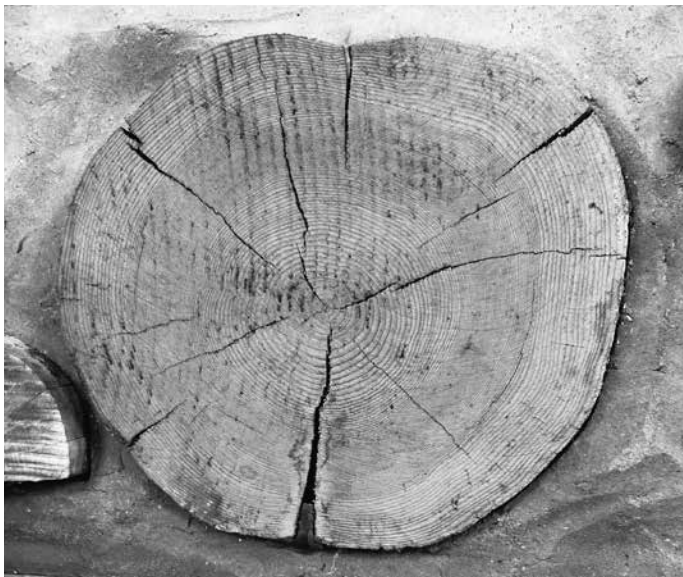
5.2: Several checks began to form during the initial drying, but one wins out, becoming the primary check; this can be filled with clear caulking down the road.
