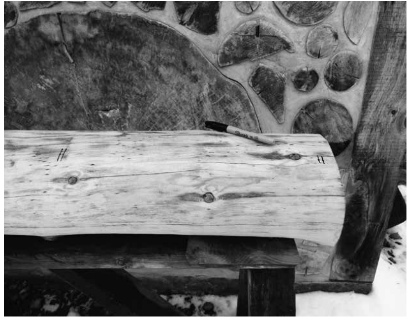
12.1: This 50-inch log is marked into 16-inch log-ends, with the quarter-inch chainsaw kerf clearly showing. The first cut cleans and trims the end. Make sure the log is supported in a sturdy manner and well clear of the ground before cutting.
