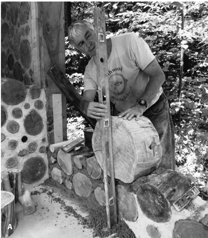
8.13: Setting a big one. (A) A likely spot presents itself in the wall, and it's about time for a big one; in this case, 13 inches in diameter. No big ones? An alternative here would be to place a little mound of mortar just over the log-end below, breaking the space up nicely for two medium logs. (B) I try the big one different ways — seldom
