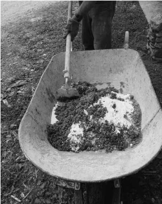
8.2: After introducing the materials into the wheelbarrow, I dry-mix it with a garden hoe, pulling it in each direction two or three times.
