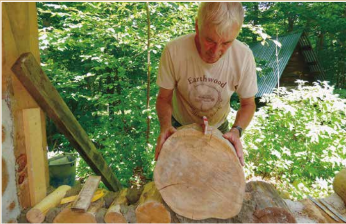
Top left: A student builds cordwood as Jaki Roy looks on, near New Norfolk, Tasmania, Australia.
