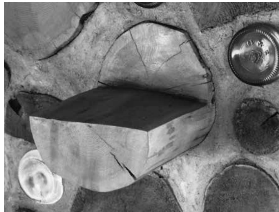
9.6: Use a log-end 6 inches or so longer than the wall thickness. Cut it half way through with a chainsaw and split off a piece with a hammer and chisel. Sand it up with a circular sander like the one in Figure 9.14. I put two or three coats of water-based urethane on shelf pieces.
