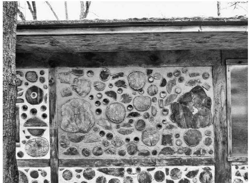
5.16: Our cobwood panel in the garage, well protected by overhang, still looks good after 16 years.
