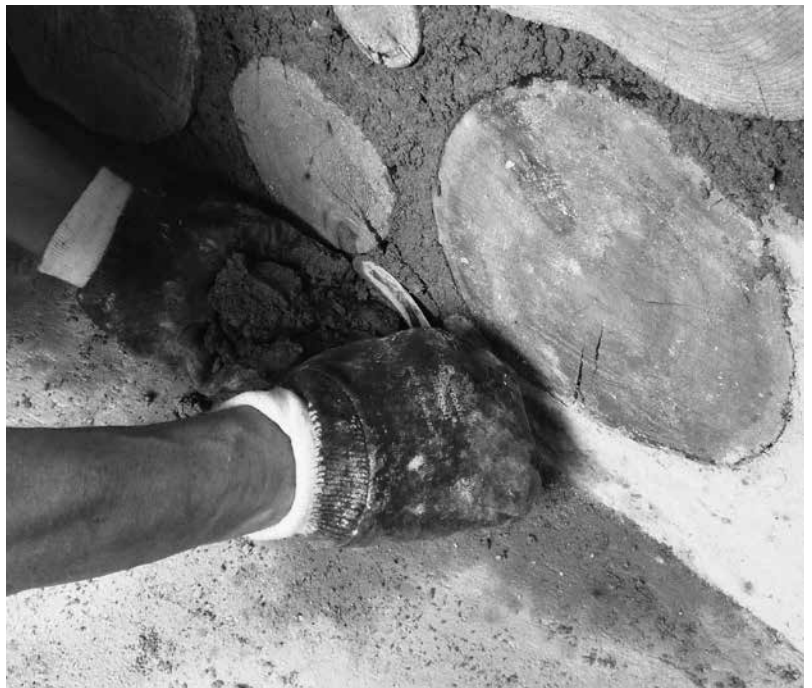
8.21: Rob rough points a little differently. He cuts away excess mortar with his knife, catching it in his gloved hand. Then he pushes this mortar into any needy cavities. He, too, looks for a consistent quarter-inch reveal. Try both methods to see which works best for you.
