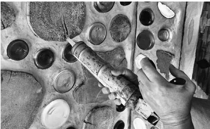
10.3: Caulk with clear siliconized caulking.
