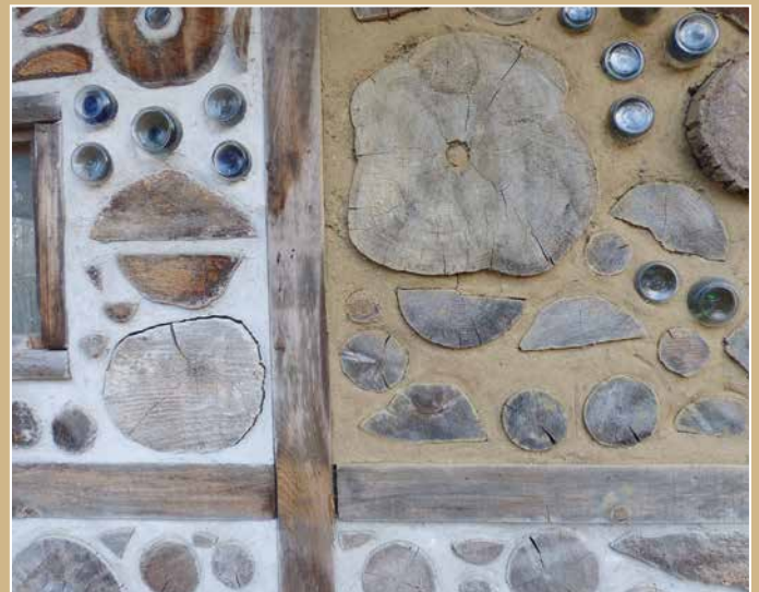
Top: Demonstration "cobwood" wall built by Rob, Jaki, and volunteers at the Natural Building Colloquium, Kingston, New Mexico.
