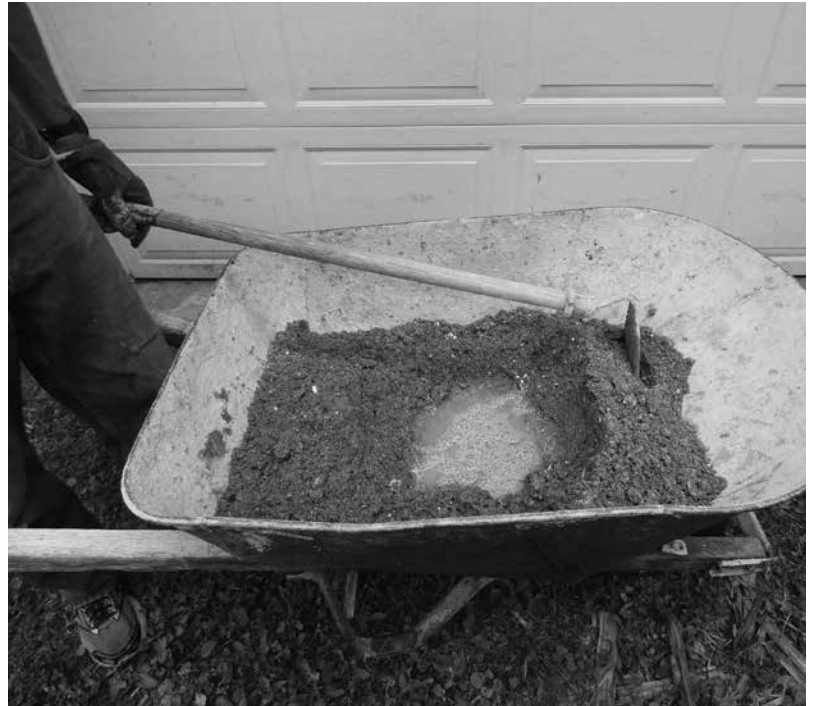
8.3: After everything is a consistent color — remember to scrape up the sand at the bottom of the barrow—make a crater of water and commence wet mixing, back and forth with the hoe until the consistency is right.
