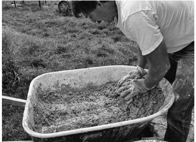
5.14: Kneading the lime putty mortar.
