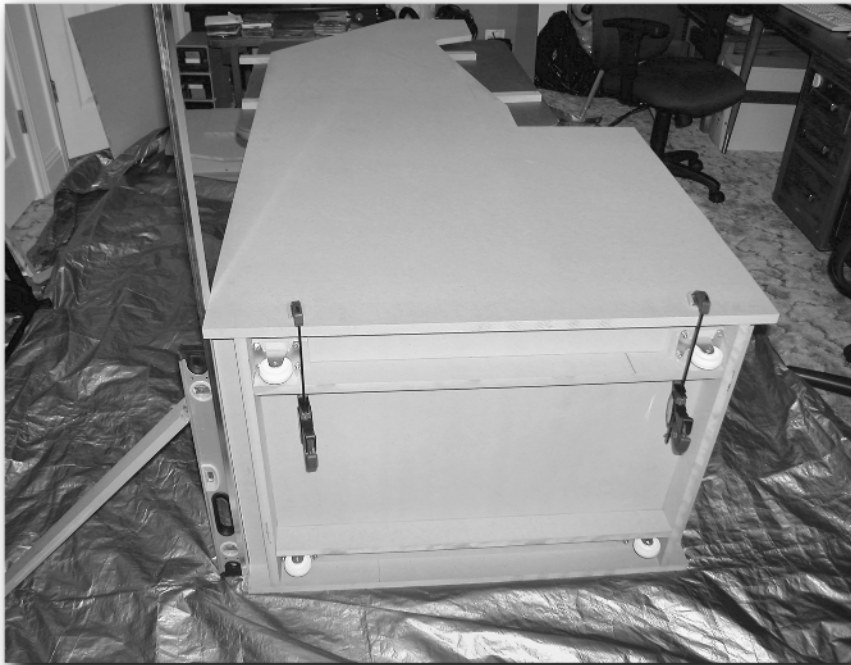
FIGURE 2-13: Making sure the cabinet base and cabinet side are square.
