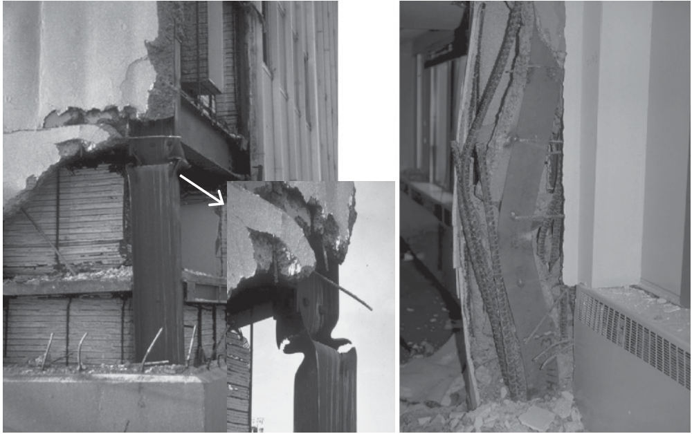
Figure B.29 Buckling in columns of the Cordova Building during the 1964 Alaska earthquake: local buckling ( left ) and member buckling ( right ) (courtesy of National Information Service for Earthquake Engineering, University of California, Berkeley) Reproduced from: Left: Image: Karl V. Steinbrugge Collection: S2202 Right: Image: Karl V. Steinbrugge Collection: S2201 URL: http://nisee.berkeley.edu/elibrary/
