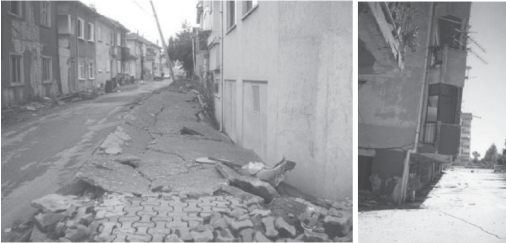
Figure 1.29 Damage observed during the 17 August 1999 Kocaeli ( left ) and the 12 November 1999 Düzce ( right ) earthquakes in Turkey
