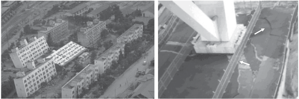
Figure 1.27 Collapses due to soil liquefaction: settlement and tilting of buildings in the 1964 Niigata (Japan) earthquake ( left ) and soil boils and cracks at pier foundations of Nishinomiya-ko bridge in the 1995 Kobe (Japan) earthquake ( right ) ( courtesy of National Information Service for Earthquake Engineering, University of California, Berkeley )
