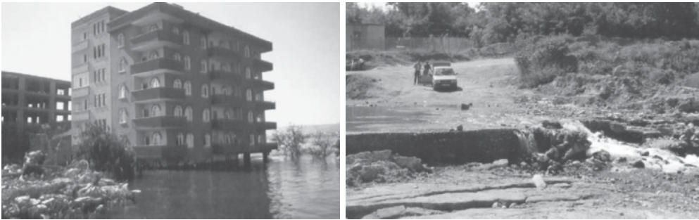
Figure 1.25 Effects of ground settlements and uplift during the 1999 Kocaeli (Turkey) earthquake: flooding ( left ) and artificial waterfalls ( right )
