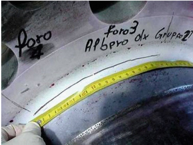
Fig. 3 Surface crack revealed by dye penetrant inspection
