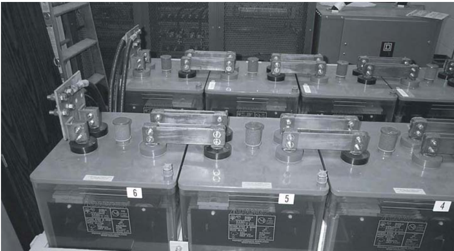
Fig. 6.31 Cell interconnecting straps.
