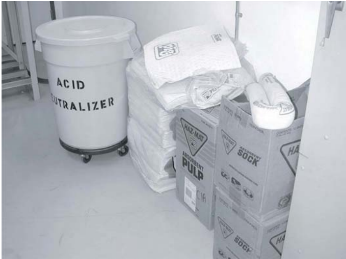
Fig. 6.35 Spill management kits. (Upper photo ( Whitham D. Reeve; lower photo courtesy M.W. Migliaro.)
