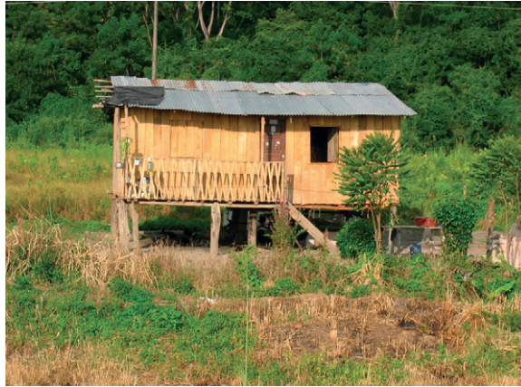
FIGURE 4-1 House built on stilts above annual flood levels in Guayas Province, Ecuador.
