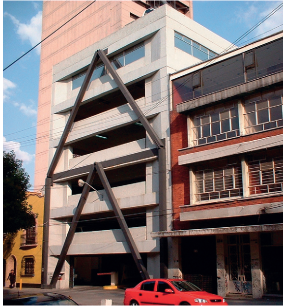
FIGURE 4–2 Mexico City parking garage with external steel frame retrofit.
