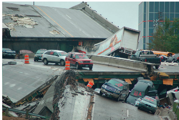
FIGURE 2–31 Collapse of the I-35 Mississippi Bridge in Minneapolis, Minnesota, August 4, 2007. (Photo courtesy of Kevin Rofidal, U.S. Coast Guard)
