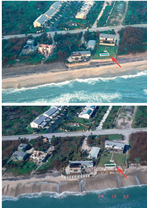
FIGURE 4-3 Example of a seawall failure following Hurricane Jeanne in 2004, Melbourne Shores, Florida. (Photo courtesy of USGS, 2004)
