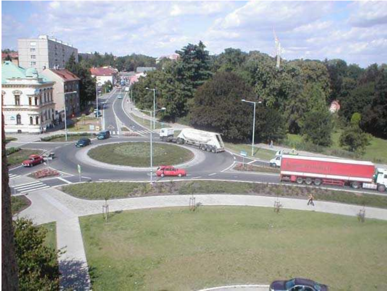
Figure 4.6. Roundabout in Chrudim (Czech Republic)
