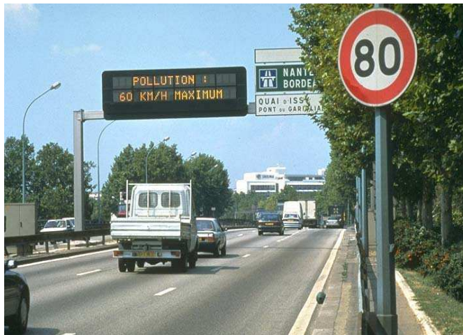
Figure 6.2. Example of inconsistency between fixed and variable message signs
