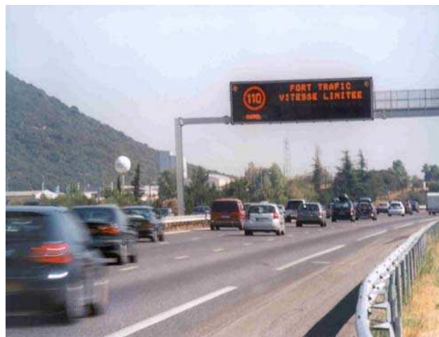
Figure 5.4. Variable speed limits on the A7 motorway (France)
