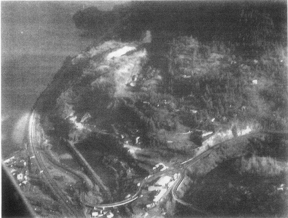
Figure 13. Highway 35 just south of I-84 is susceptible to landslide failure.
