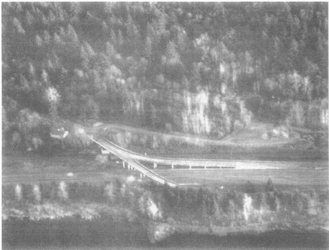
Figure 12. The Bridal Veil exit 28 off-ramp on I-84 is susceptible to earthquake damage.
