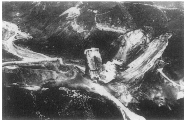
Figure 5. 1928 failure of St. Francis Dam.
