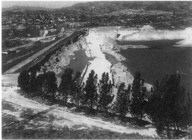
Figure 13. Lower San Fernando Dam, looking to the west from the east abutment area, showing upstream slope slide into the reservoir.
