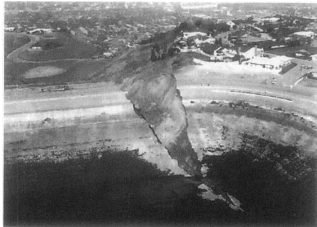
Figure 34. 1963 Baldwin Hills Reservoir failure through the dam abutment [73].
