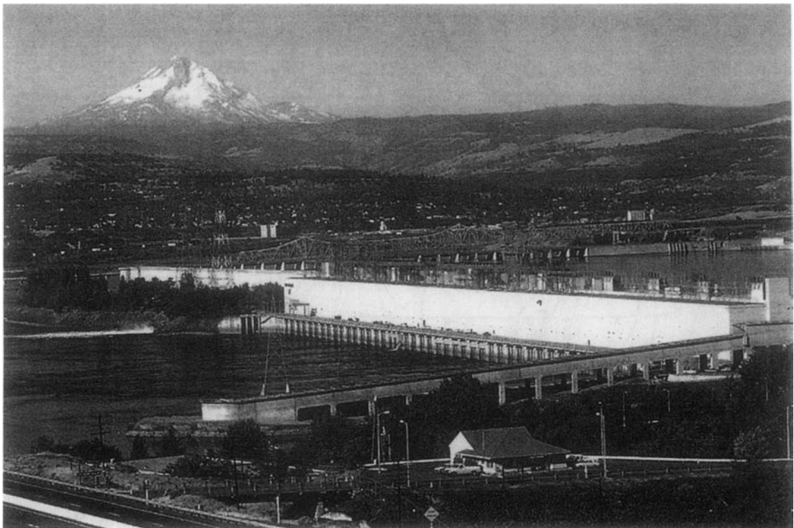
Figure 10. View of The Dalles hydroelectric facilities and Mount Hood, an active volcano, in the background (USACE photo).
