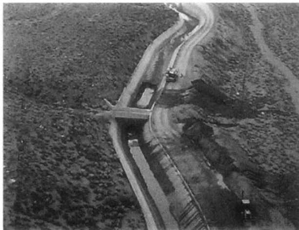
Figure 28. Typical overcrossing of LAA.
