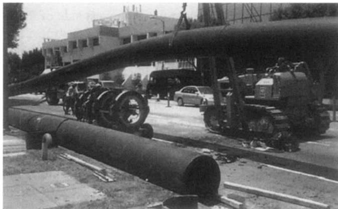
Figure 27. HDPE lining of 36-inch (900 mm) diameter Pico Boulevard riveted steel pipe.
