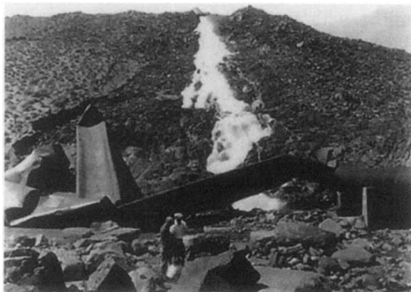
Figure 35. LAA bombing damage during 1920’s “Water Wars.”
