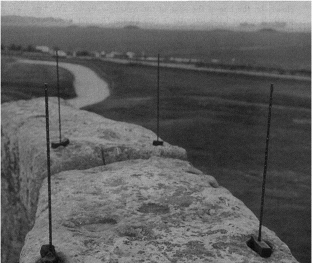
Marker holes discovered on top of the lintels.
