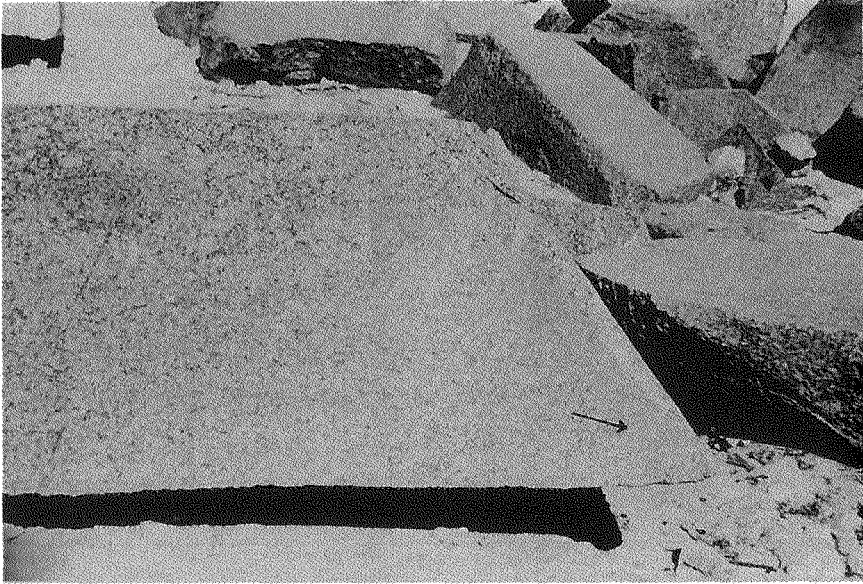
Granite block from the base of the Great Pyramid showing the slope angle.
