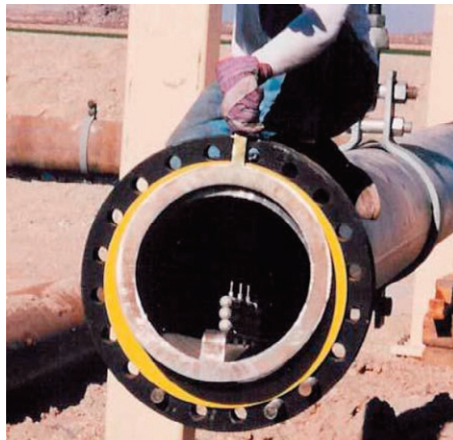
Figure 10.3 Insertion of the “coupon tree” into the pipeline (Moore et al., 2002).
