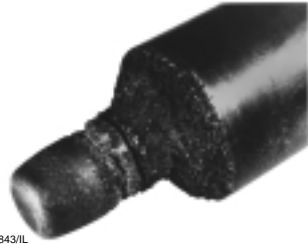
Figure 5-7. Typical Appearance of Cavitation Damage
