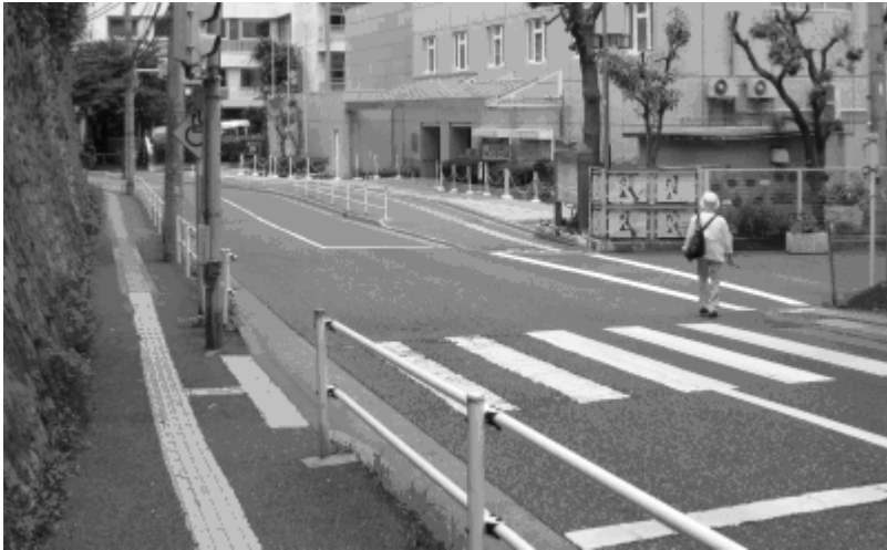
Fig. 1. Braille blocks paved on a side walk in Japan. The blocks have two types, one of them is “directional blocks” which indicate its direction and the other one is “warning blocks” which indicate end point or intersection point or a kind of caution.
