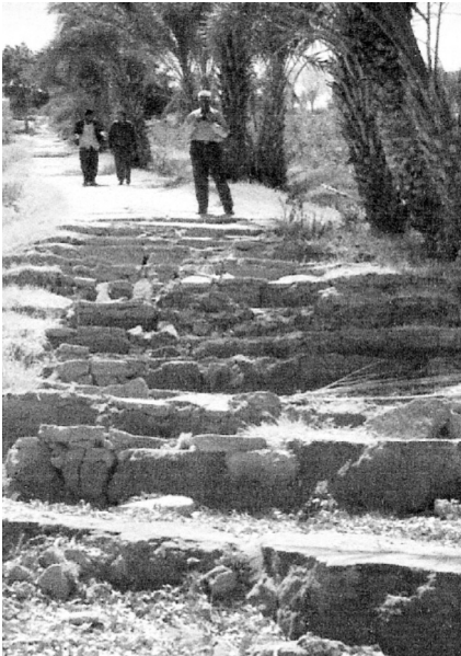
Fig. 11.1 Extensional ground cracking (photo by James Hengesh)
