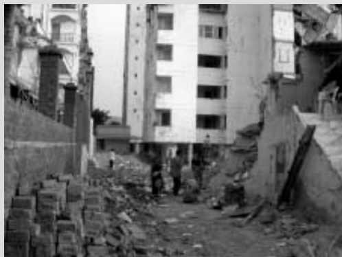
Fig. 11.6 Failure due to soft storey
