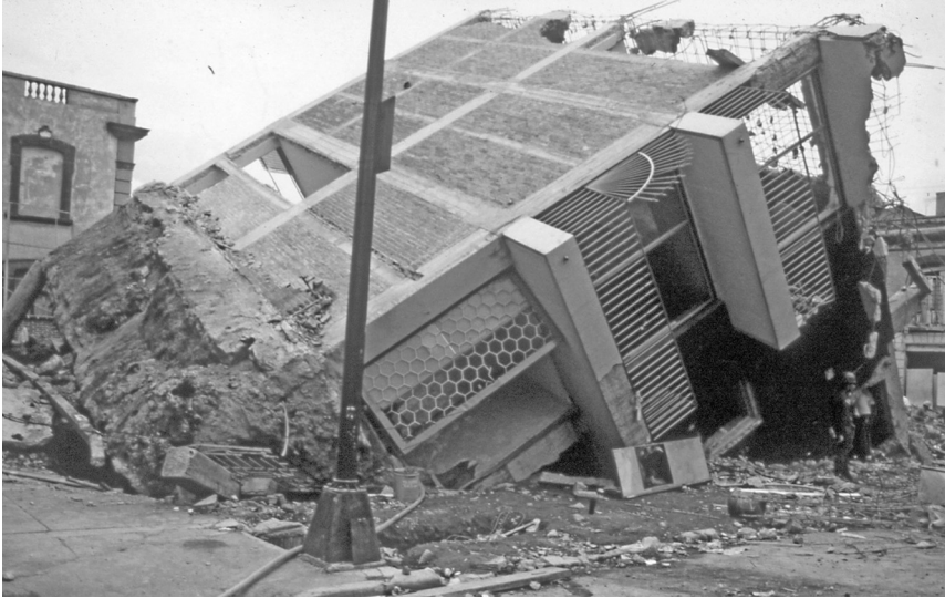
Figure 7.2 Bearing capacity failure in Mexico City, 1985 (photograph courtesy of J. Pappin)
