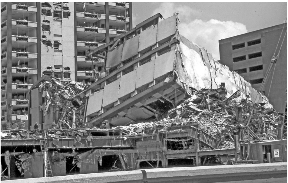
Figure 9.1 Collapse of Pinot Suarez building, Mexico City, 1985 (© E Booth)
