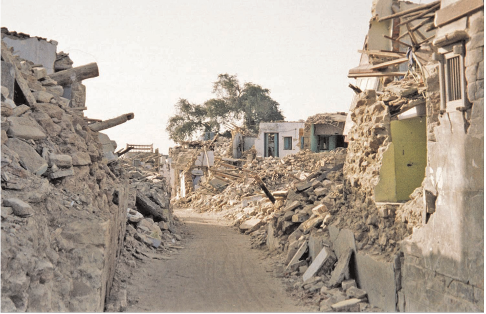
Figure 10.1 Failure of weak masonry buildings in Gujarat, 2001 (© E Booth)
