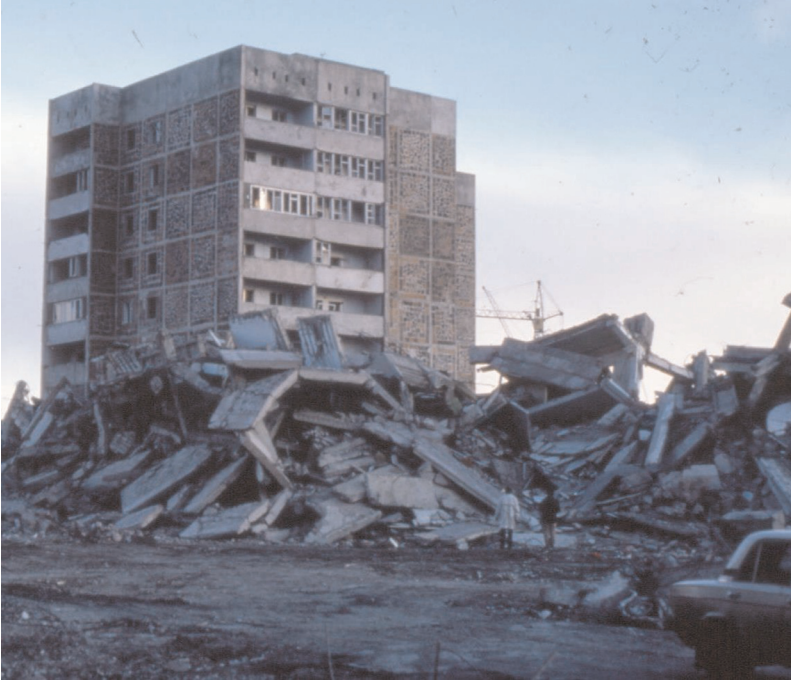
Figure 5.3 Collapsed precast concrete frame buildings (foreground) with precast wall building behind, Spitak Armenia, 1988 (photograph source unknown)
