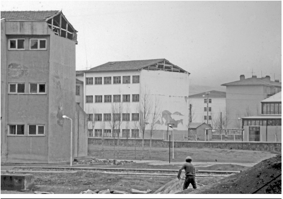
Figure 10.6 Gable end failure in the Erzincan, Turkey earthquake of 1992. Note that the sloping (hipped) gable on the farthest building on the right has not failed (© E Booth)
