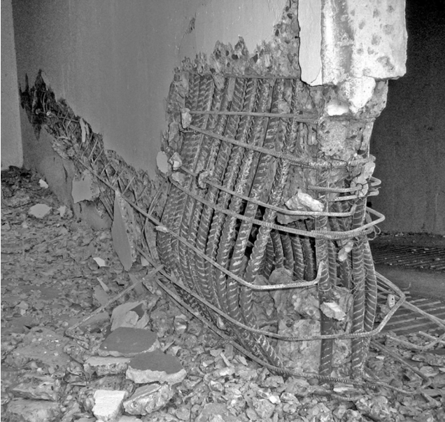
(a) Compression failure of outside edge of shear wall, Chile 2010
