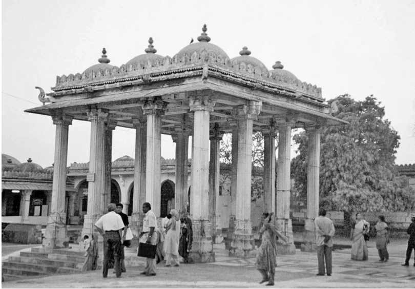
Figure 10.11 Unreinforced masonry structure which survived the Gujarat, India earthquake of 2001 (© E Booth)
