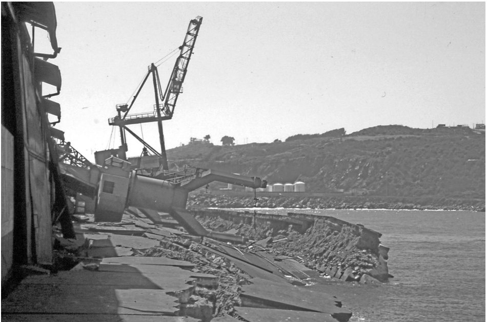
Figure 7.6 Failure of a quay wall, San Antonio, Chile, 1985 (© E Booth)
