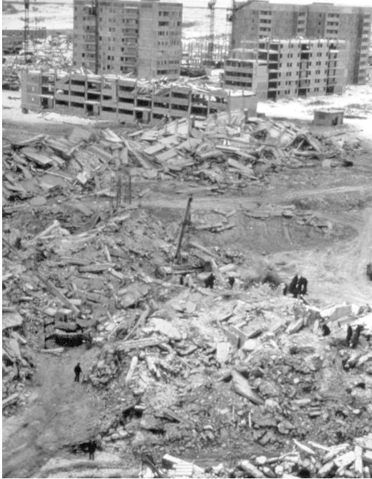
Figure 8.10 Survival of precast panel buildings adjacent to razed precast frame buildings, Spitak, Armenia, 1988 (courtesy ABS Consulting, photograph from Peter Yanev, EQE, San Francisco)
