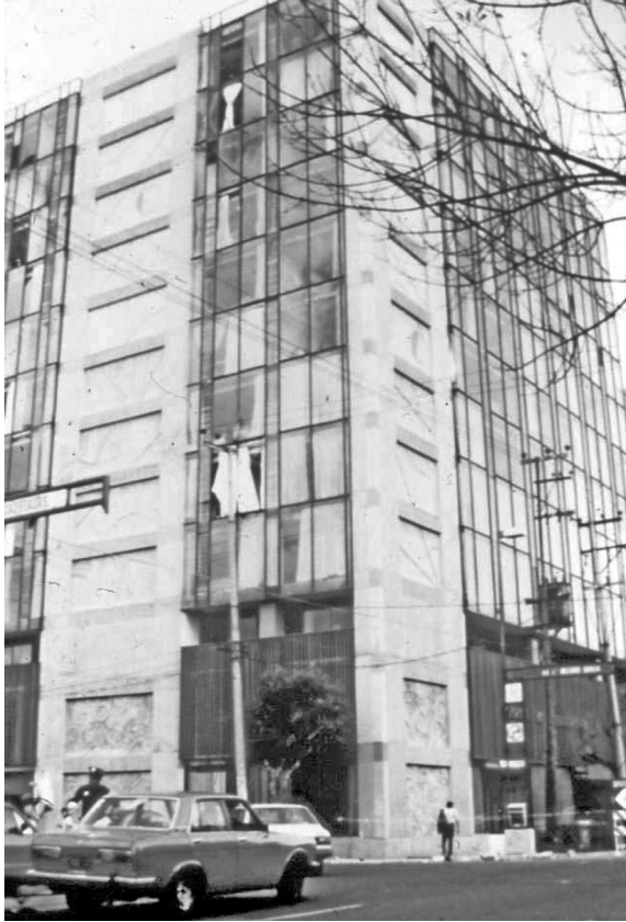
Figure 14.2 Building in Mexico City after the 1985 earthquake. The building had previously been strengthened by the addition of the external shear walls seen in the photograph
