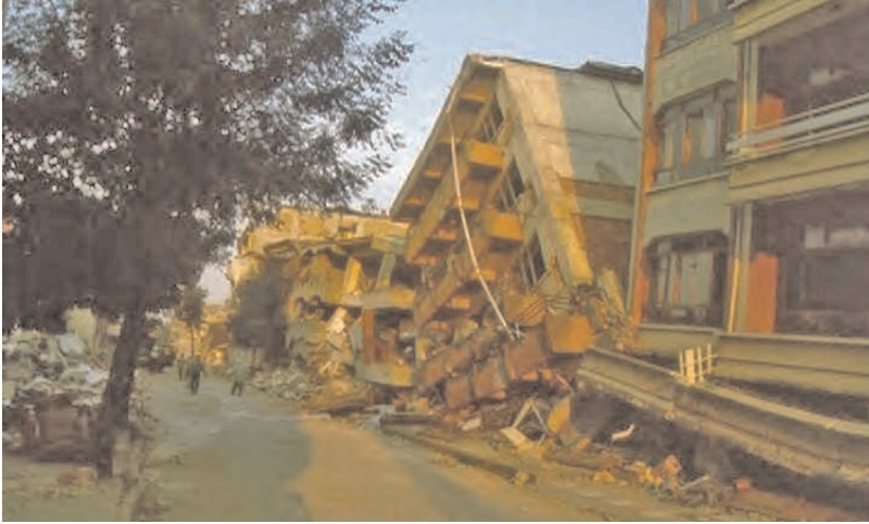
Figure 8.4 Ground storey (soft storey) collapse of buildings in Kocaeli, Turkey, 1999 (courtesy Earthquake Engineering Field Investigation Team (EEFIT), UK)
