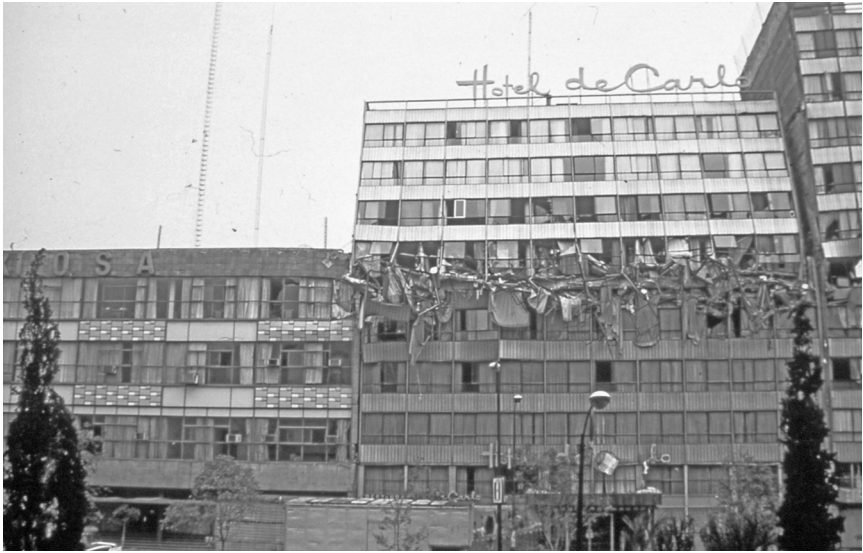
Figure 8.8 Failure in Mexico, 1985, caused by impact between adjacent buildings (© E Booth)
