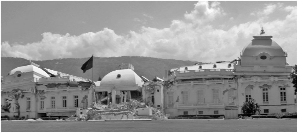
Figure 1.3 Presidential palace, Port-au-Prince, Haiti after the 2010 Haiti earthquake (photograph courtesy of G. Madabhushi)
