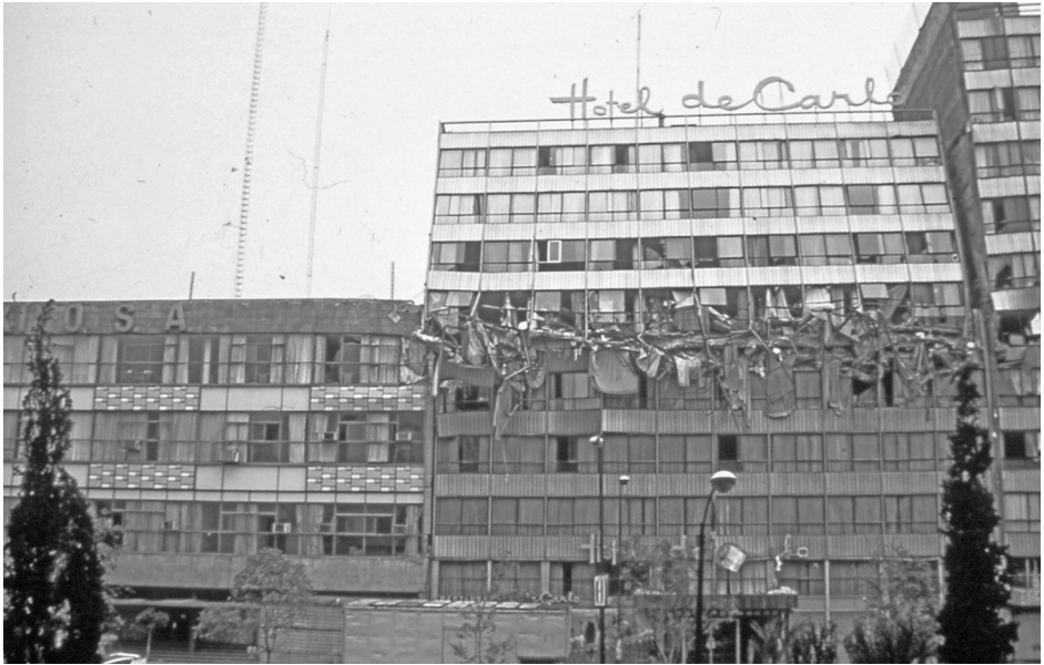
Figure 5.1 Buffeting damage, Mexico City, 1985
