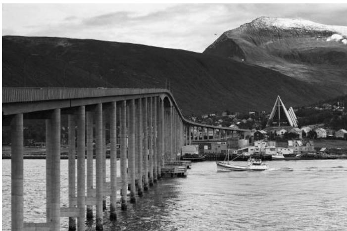
*Figure 1.4* The Tromsø Bridge (1960) is a cantilever bridge with a total length of 1016 m. (Courtesy of Johan Brun.)
