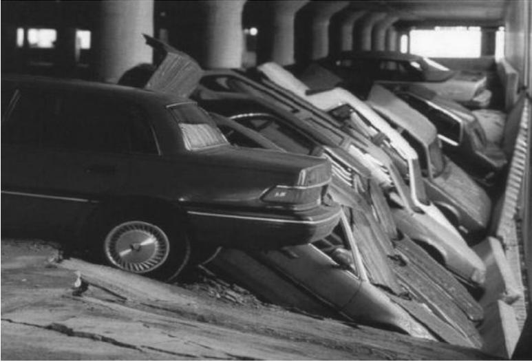
Figure 2.63 The consequences of rebar corrosion in parking garages exposed to de-icing salt contamination have occasionally been quite severe. (From Simon, P., Improved Current Distribution due to a Unique Anode Mesh Placement in a Steel Reinforced Concrete Parking Garage Slab CP System, in *NACE Corrosion 2004*, Paper 04345, 2004.)
