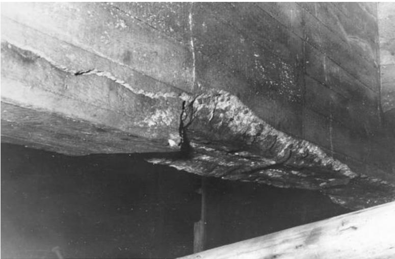
Figure 2.10 The lower parts of the deck beams were typically more vulnerable to steel corrosion than the deck slabs in between. (From Gjørnv, O. E., *Durability of Reinforced Concrete Wharves in Norwegian Harbours*, Ingeniørforlaget AS, Oslo, Norway, 1968.)
