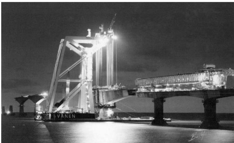
Figure 5.8 Installation of cantilever girders for the Northumberland Strait Bridge. (From Malhotra, V. M., *Proceedings, Third International Conference on Performance on Concrete in Marine Environment*, ACI SP-163, 1996.)
