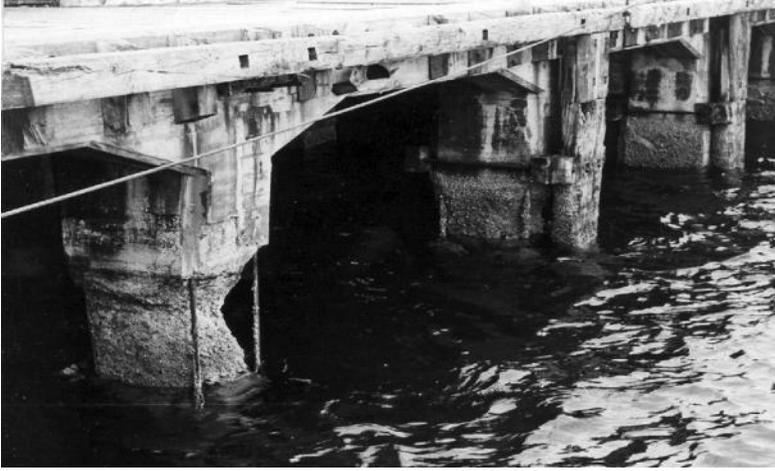
Figure 2.9 Uneven deterioration in the tidal zone due to high scatter and variability of achieved concrete quality from one pillar to another. (From Gjørnv, O. E., *Durability of Reinforced Concrete Wharves in Norwegian Harbours*, Ingeniørforlaget AS, Oslo, Norway, 1968.)
