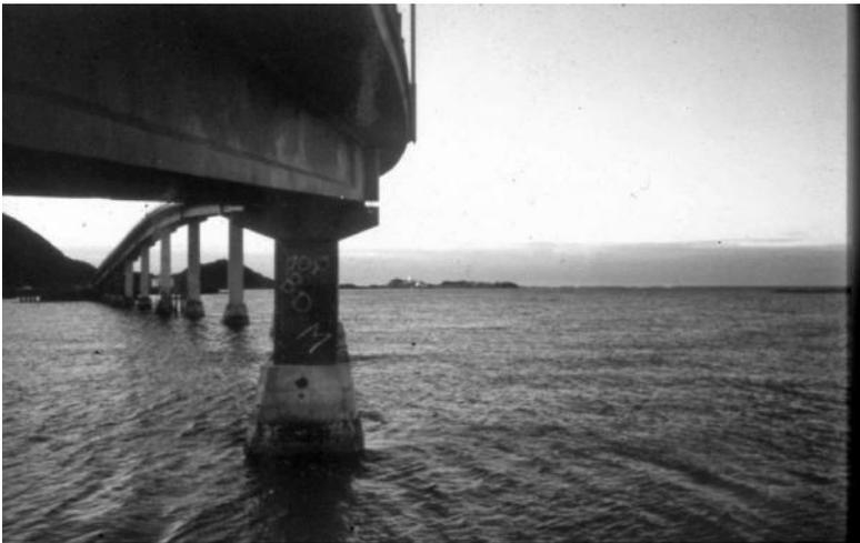
*Figure 2.35* Ullasundet Bridge (1970) was demolished after 25 years of service due to heavy corrosion of embedded steel. (Courtesy of Jørn A. Hasselø.)
