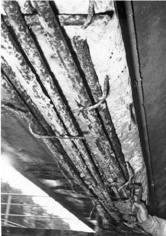
*Figure 2.12* When the concrete cover in the lower parts of the deck beams had cracked or spalled off at a very early stage, the steel bars were more uniformly corroded, while the vertical beam stirrups typically showed a more severe pitting and were often rusted through. (From Gjørnv, O. E., *Durability of Reinforced Concrete Wharves in Norwegian Harbours*, Ingeniørforlaget AS, Oslo, Norway, 1968.)
