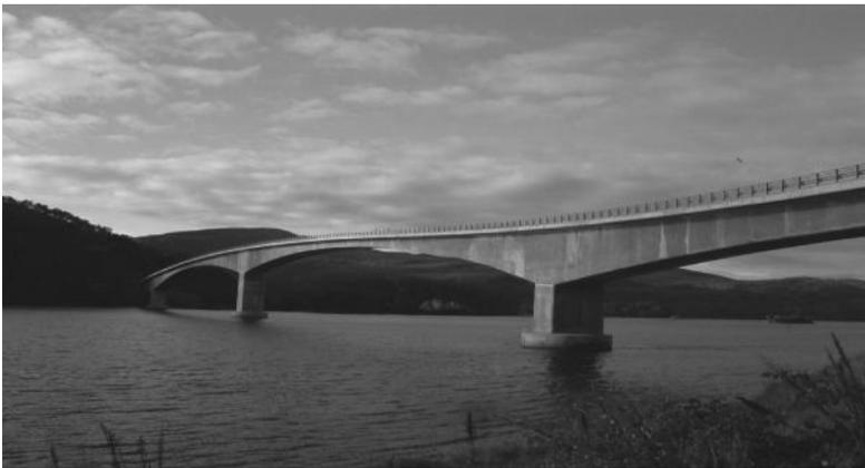
Figure 2.48 The Aursundet Bridge (1995) is a cantilever bridge with a total length of 486 m.
