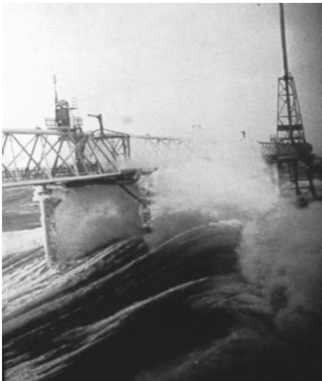
*Figure 2.51* All the concrete platforms in the North Sea are exposed to heavy wave loading and splashing of seawater.
