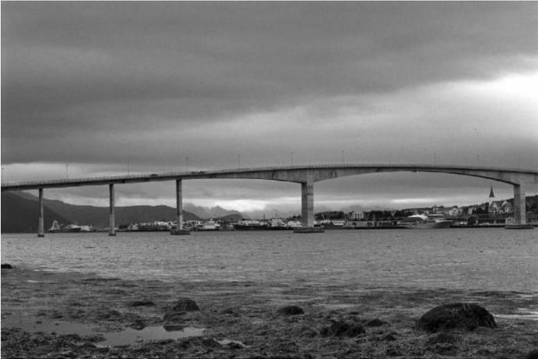
*Figure 2.1* The Sortland Bridge (1975) is a 948 m long cantilever bridge in the northern part of Norway. (Courtesy of Johan Brun.)
