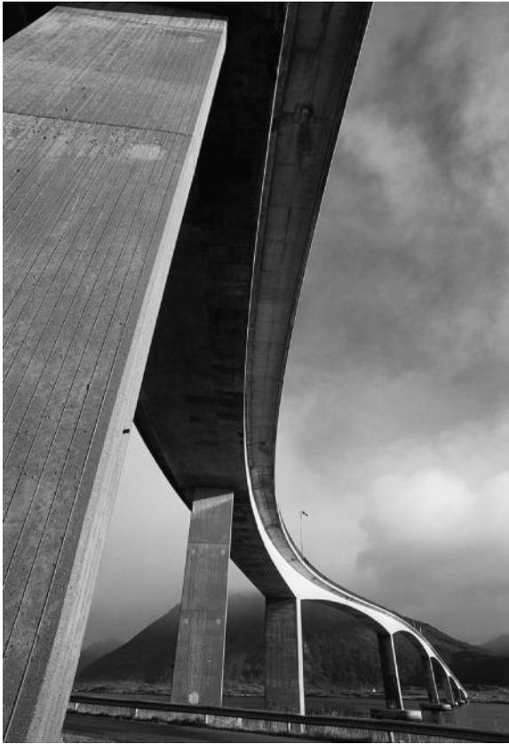
*Figure 2.36* Gimsøystraumen Bridge (1981) is a cantilever bridge, which is a very common type of bridge along the Norwegian coastline. (Courtesy of Johan Brun.)
