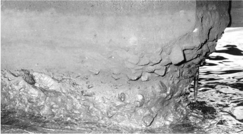
Figure 2.7 Deterioration in the tidal zone mostly due to freezing and thawing. (From Gjrrv, O. E., *Durability of Reinforced Concrete Wharves in Norwegian Harbours*, Ingenirforlaget AS, Oslo, Norway, 1968.)
