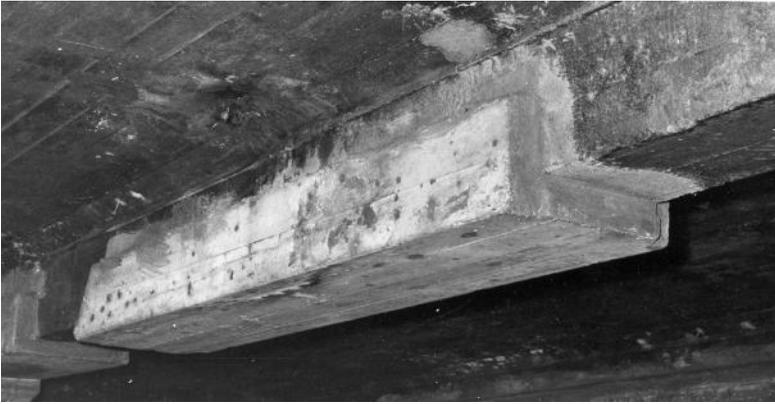
Figure 2.14 Typical patch repair of a corroded deck beam. (From Gjrv, O. E., *Durability of Reinforced Concrete Wharves in Norwegian Harbours*, Ingenirforlaget AS, Oslo, Norway, 1968.)
