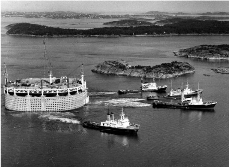
Figure 1.8 The first offshore concrete platform, the Ekofisk Tank, on its way out from Stavanger in 1973. (Courtesy of Norwegian Contractors.)
