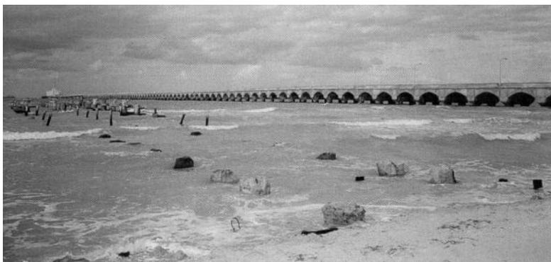
*Figure 2.31* Different durability and long-term performance of the two concrete piers on the Yucatán Coast built with black steel in the 1960s (front) and with stainless steel reinforcement during 1937–1941, respectively. (Courtesy of Rambøll Consulting Engineers.)
