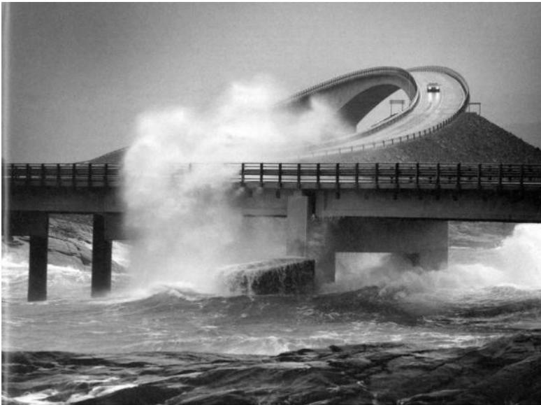
*Figure 2.42* During stormy winter periods, Storseisund Bridge (1988) is heavily exposed to splashing of seawater. (Courtesy of Rolf Jarle Ødegaard.)
