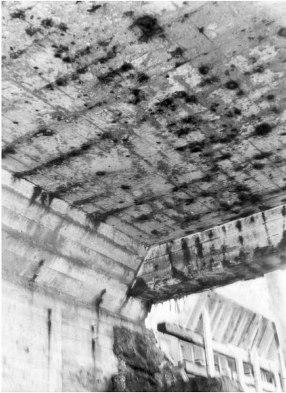
*Figure 2.11* The rear parts of the concrete deck adjacent to the seawall were typically more vulnerable to steel corrosion than the rest of the deck. (From Gjørsv, O. E., *Durability of Reinforced Concrete Wharves in Norwegian Harbours*, Ingeniørforlaget AS, Oslo, Norway, 1968.)
