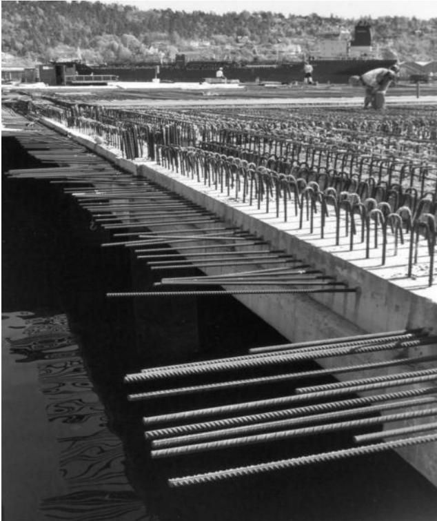
Figure 9.5 Protruding bars in the construction joints of the concrete deck.
