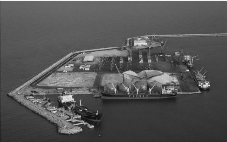
*Figure 2.34* The outer part of the Progreso Pier is an important extension of the old concrete pier that was produced with stainless steel reinforcement during 1937–1941. (Courtesy of Progreso Port Authorities.)
