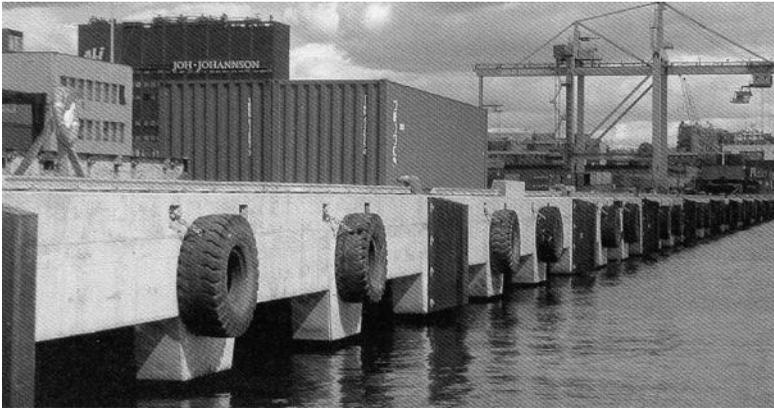
Figure 9.1 Container Terminal I (2002) in Oslo Harbor consists of an open concrete deck on top of driven steel tubes filled with concrete.
