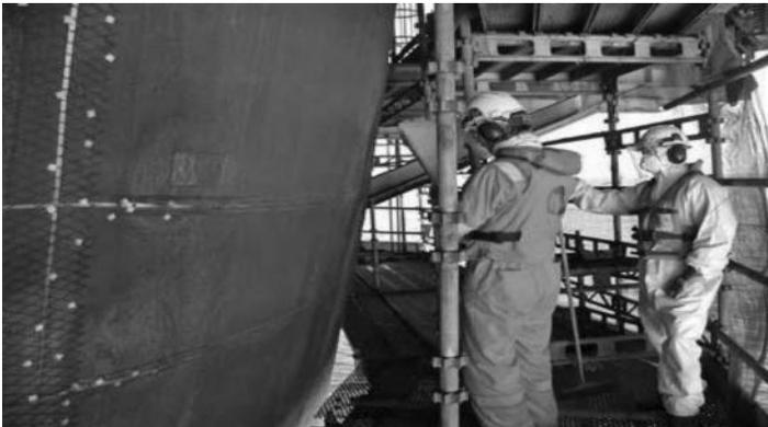
Figure 2.53 After 13 years of service, extensive and very costly repairs based on cathodic protection of the Oseberg A Platform (1988) were carried out. (Courtesy of Trond Østmoen.)
