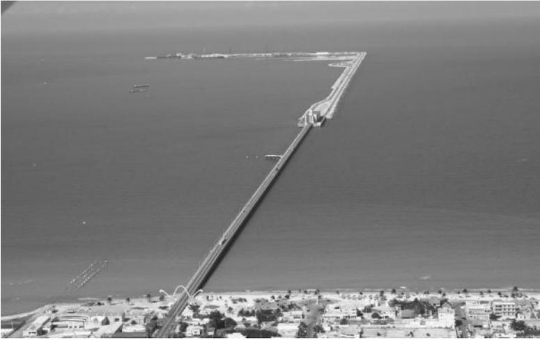
*Figure 2.33* Overview of the Progreso Pier with stainless steel reinforcement still in good condition after about 70 years of operation. (Courtesy of Progreso Port Authorities.)
