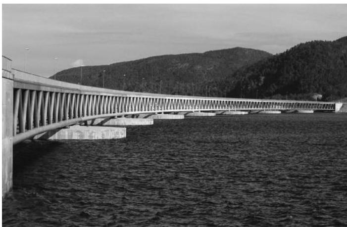
*Figure 1.5* The Bergsøysund Bridge (1992) is a floating bridge with a total length of 914 m. (Courtesy of Johan Brun.)
