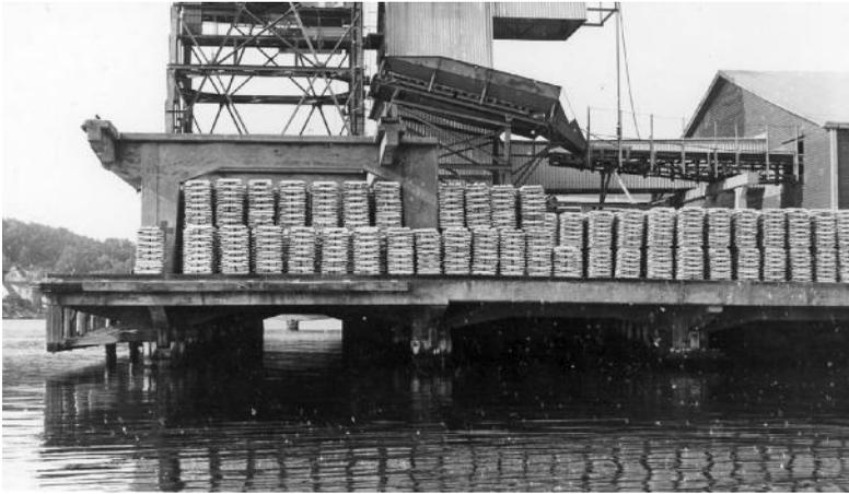
Figure 2.6 A 50-year-old industrial harbor structure (1913) with storage of raw aluminum bars representing an evenly distributed deck load of approximately six times that of the original design load. (From Gjørsv, O. E., *Durability of Reinforced Concrete Wharves in Norwegian Harbours*, Ingeniørforlaget AS, Oslo, Norway, 1968.)
