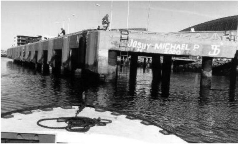
Figure 2.20 The cruise terminal Turistskipskaia (1993) in Trondheim Harbor with steel corrosion in most of the deck beams after eight years of service. (From Gjørsv, O. E., *Durability and Service Life of Concrete Structures*, in *Proceedings, The First FIB Congress*, 8, 6, Japan Prestressed Concrete Engineering Association, Tokyo, Japan, 2002, pp. 1–16.)
