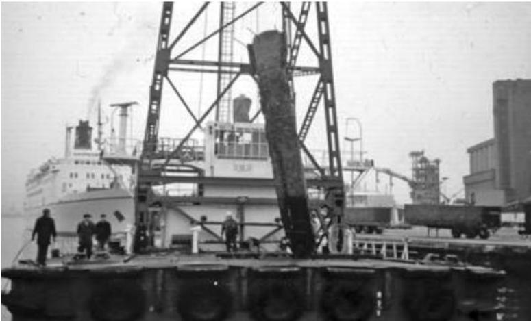
Figure 2.18 Four of the tremie-cast concrete pillars from the concrete jetty in Oslo Harbor (1922) were pulled up on shore for a very detailed condition assessment of the embedded steel.
