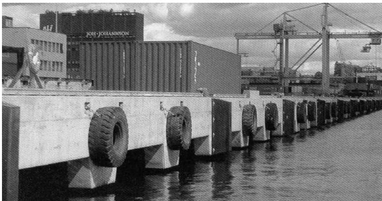
Figure 2.27 During concrete construction of the container terminal Nye Filipstadkaia (2002) in Oslo Harbor, a deep chloride ingress in several of the freshly cast deck beams took place due to heavy wind and high tides. (Courtesy of Oslo Harbor KF.)
