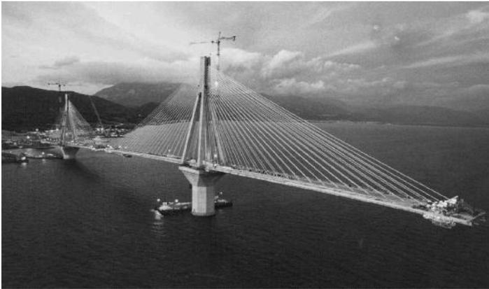
Figure 1.14 The Rion–Antirion Bridge (2001), for which a concrete with an extremely high resistance against chloride ingress was applied. (Courtesy of Gefyra S.A.)
