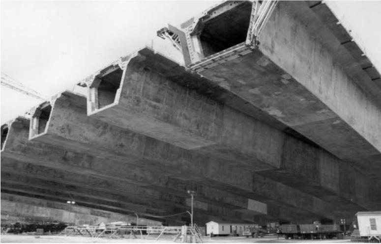
Figure 5.6 Precast cantilever girders for the Northumberland Strait Bridge.
