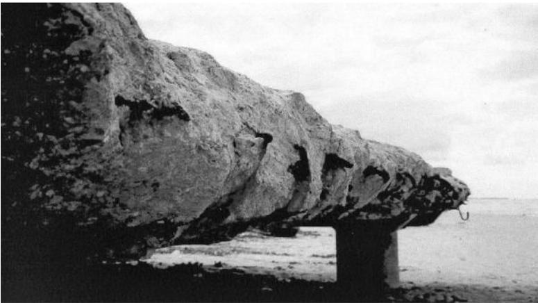
*Figure 2.30* Remaining part of the deck from the concrete pier built on the Yucatán Coast in the 1960s. (Courtesy of Rambøll Consulting Engineers.)
