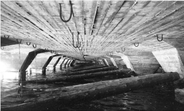
Figure 2.13 Harbor structures with a concrete deck of the flat type typically showed a much better performance than structures with a beam and slab type of deck. (From Gjørsv, O. E., *Durability of Reinforced Concrete Wharves in Norwegian Harbours*, Ingeniørforlaget AS, Oslo, Norway, 1968.)
