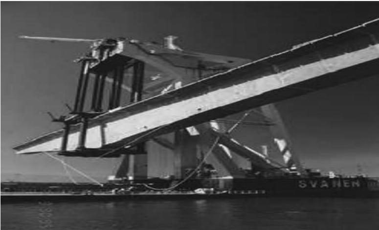
Figure 5.7 Precast cantilever girder for the Northumberland Strait Bridge.
