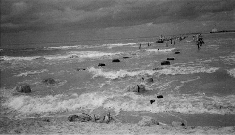
*Figure 2.29* Remaining parts of a concrete pier built with black steel reinforcement on the Yucatán Coast in Mexico in the 1960s. (Courtesy of Rambøll Consulting Engineers.)
