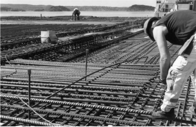
Figure 9.6 The concrete deck had very congested reinforcement.
