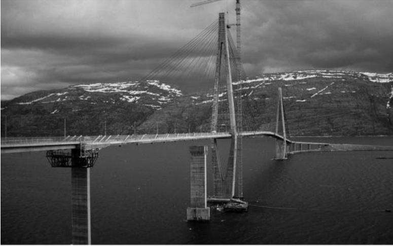
Figure 2.45 The Helgelands Bridge (1991) is a 1065 m long cable-stayed bridge with the largest span of 425 m. (Courtesy of Hallgeir Skog)
