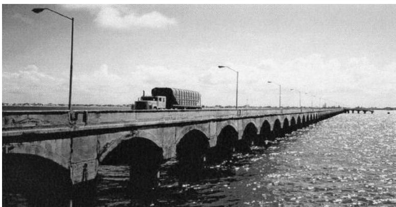
*Figure 2.32* Progreso Pier on the Yucatán Coast built with stainless steel reinforcement during 1937–1941. (Courtesy of Rambøll Consulting Engineers.)
