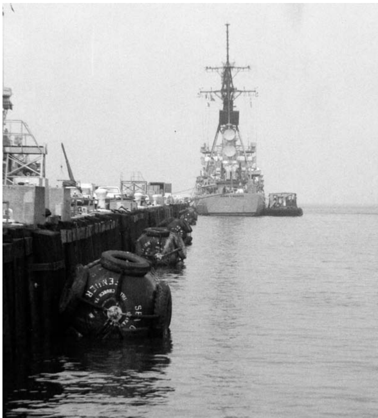
Fig. 5-15. Pneumatic-type floating fenders alongside pier
