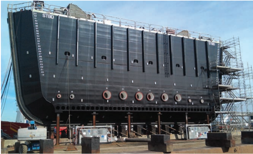
Fig. 10-15. Floating caisson gate under construction
