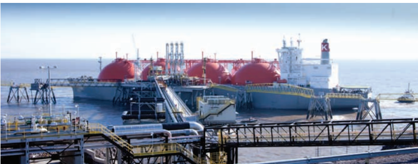
Fig. 1-2. The Canaport LNG terminal in the Bay of Fundy, Saint John, New Brunswick, Canada, is capable of receiving the world’s largest LNG vessels
