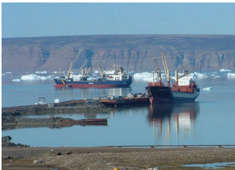
Fig. 1-9. The world's most northern seaport at Thule, Greenland, constructed of float-in jack-up steel-hulled barges
