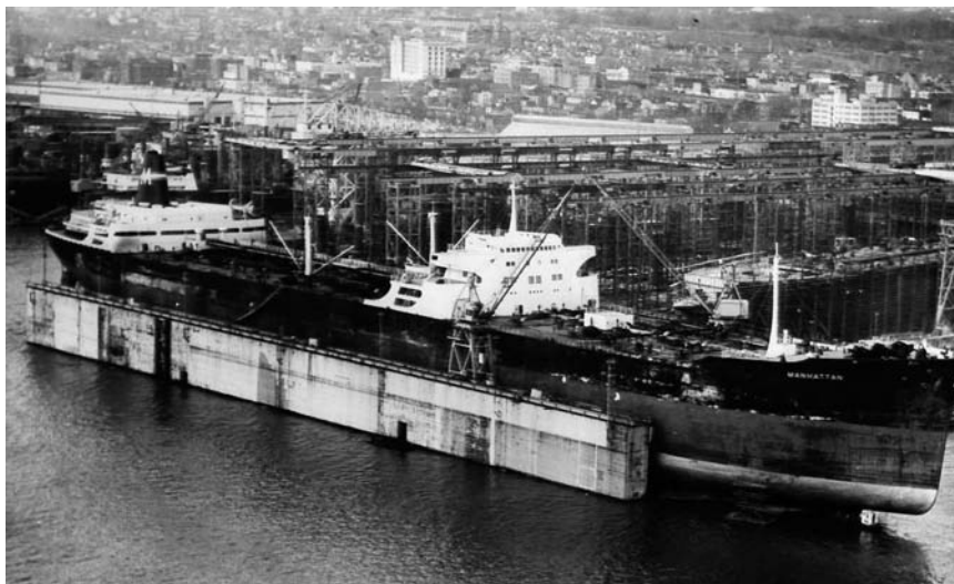
Fig. 10-2. Floating dry dock with large vessel overhang
