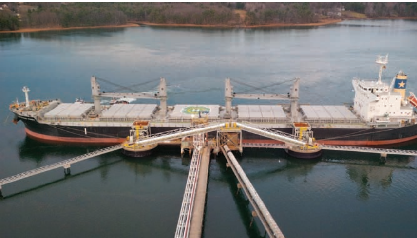
Fig. 7-28. Service platform at combination liquid/bulk handling facility with approach trestle supporting product lines and roadway and catwalks to access mooring dolphins
