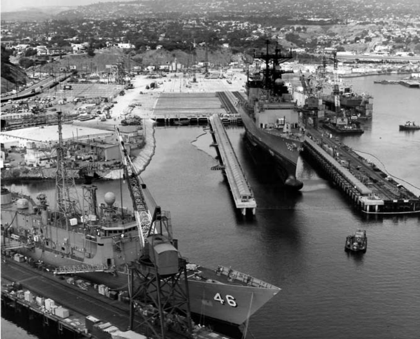
Fig. 10-43. Original largest Sychrolift installation
