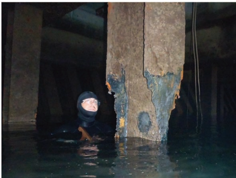
Fig. 12-4. Inspector evaluating steel H-pile within high corrosion zone near low water
