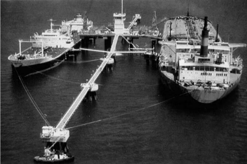
Fig. 1-1. An offshore “sea-island” type tanker berth. Crude oil transshipment terminal off Grand Bahama Island, Bahamas
