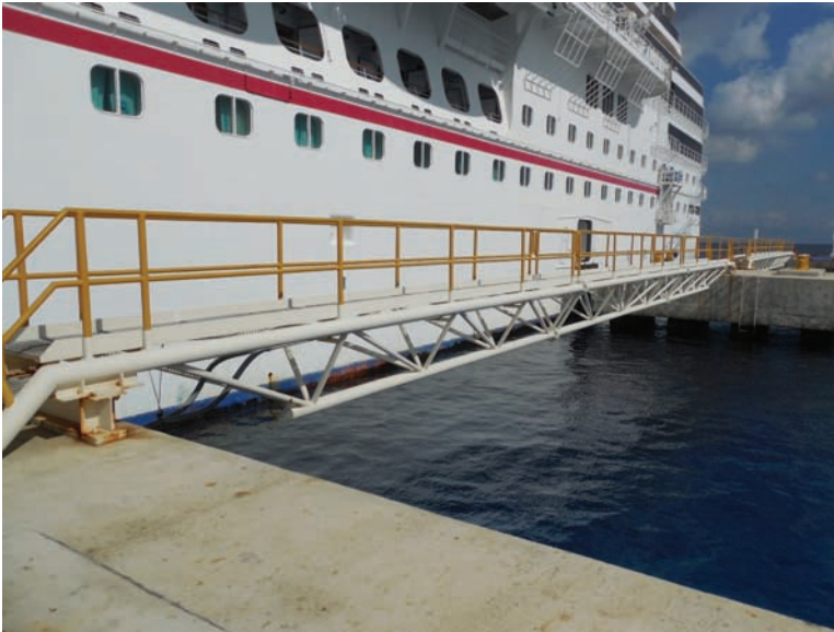
Fig. 7-30. Steel catwalk with triangular pipe truss for dolphin access
