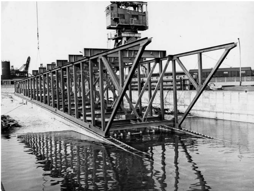
Fig. 10-22. Photograph of built-up cradle under construction
