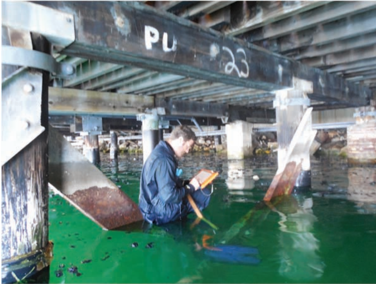
Fig. 12-10. Engineer-diver using a tablet to document conditions during a waterfront inspection
