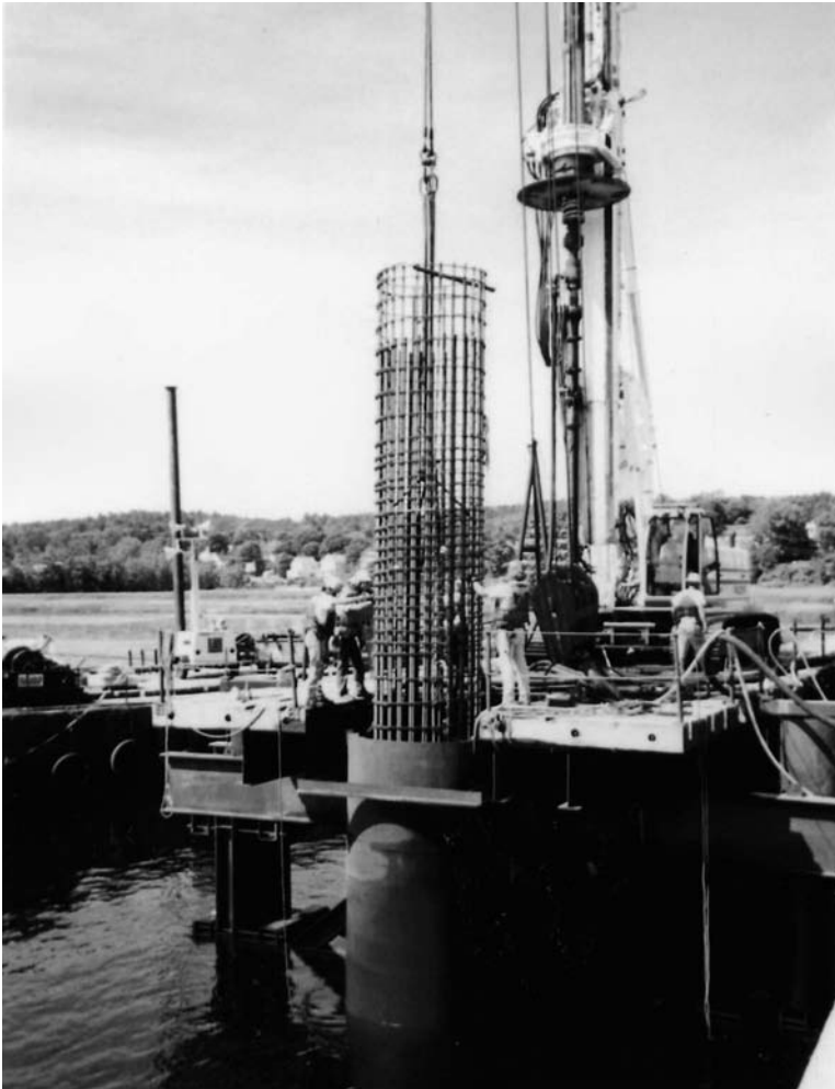
Fig. 8-21. Steel reinforcing cage being installed in a 6-ft-diameter drilled shaft
