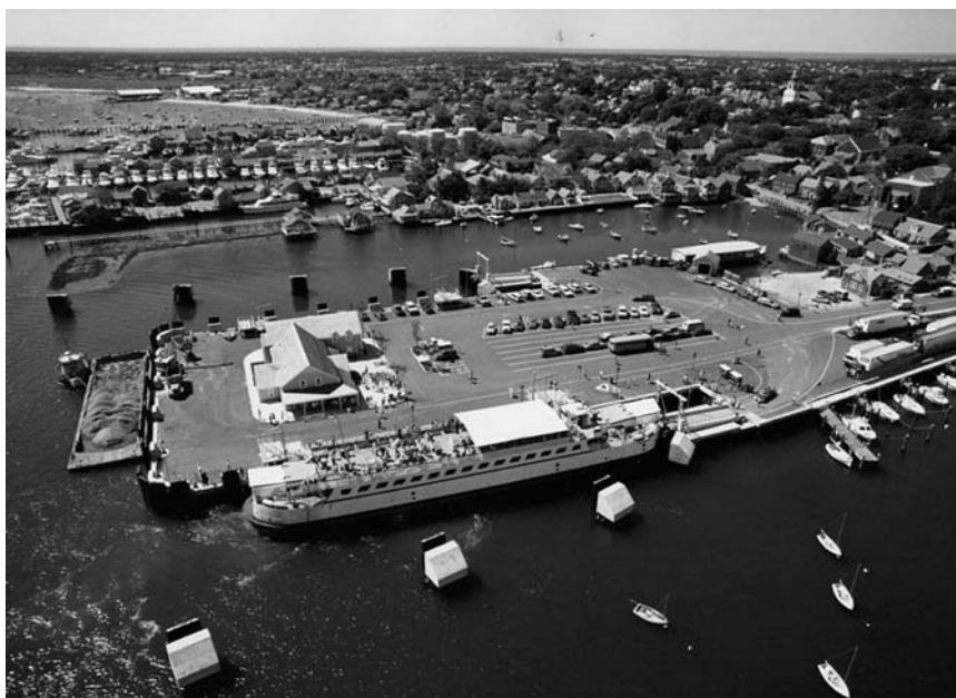
Fig. 1-6. A passenger and vehicle ferry terminal with two ferry slips at Nantucket Island, Massachusetts. Note guide-in dolphins and wharf corner fenders for “warping” of vessel. Also note queuing areas for cars and tractor trailers
