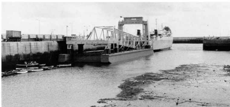
Fig. 9-4. Submersible-type movable link-span alongside quay at Douglas, Isle of Man
