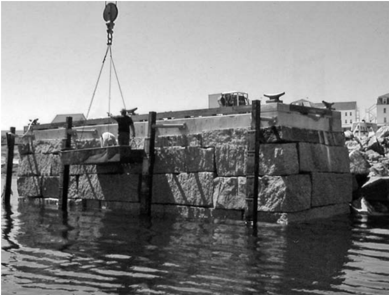
Fig. 11-16. Granite masonry pier reconstruction
