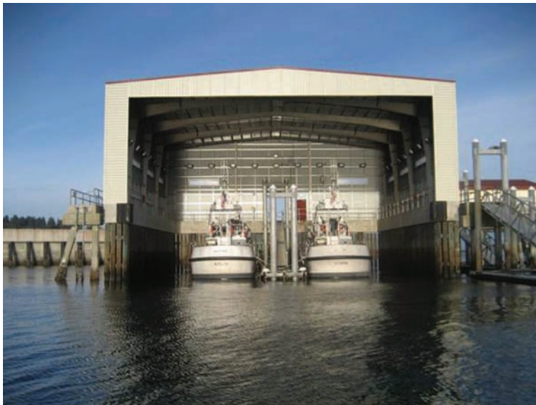
Fig. 4-10. Prefabricated metal boat house founded on pile-supported concrete finger piers at U.S. Coast Guard Search and Rescue (SAR) Station
