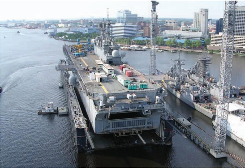
Fig. 10-32. Modern floating dry dock at Norfolk, Virginia
