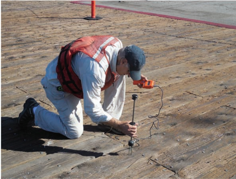
Fig. 12-5. Inspector completing moisture measurement on timber deck
