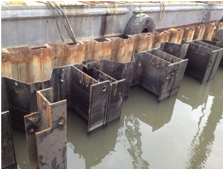
Fig. 8-8. Installation of H-Z steel sheeting using double king piles
