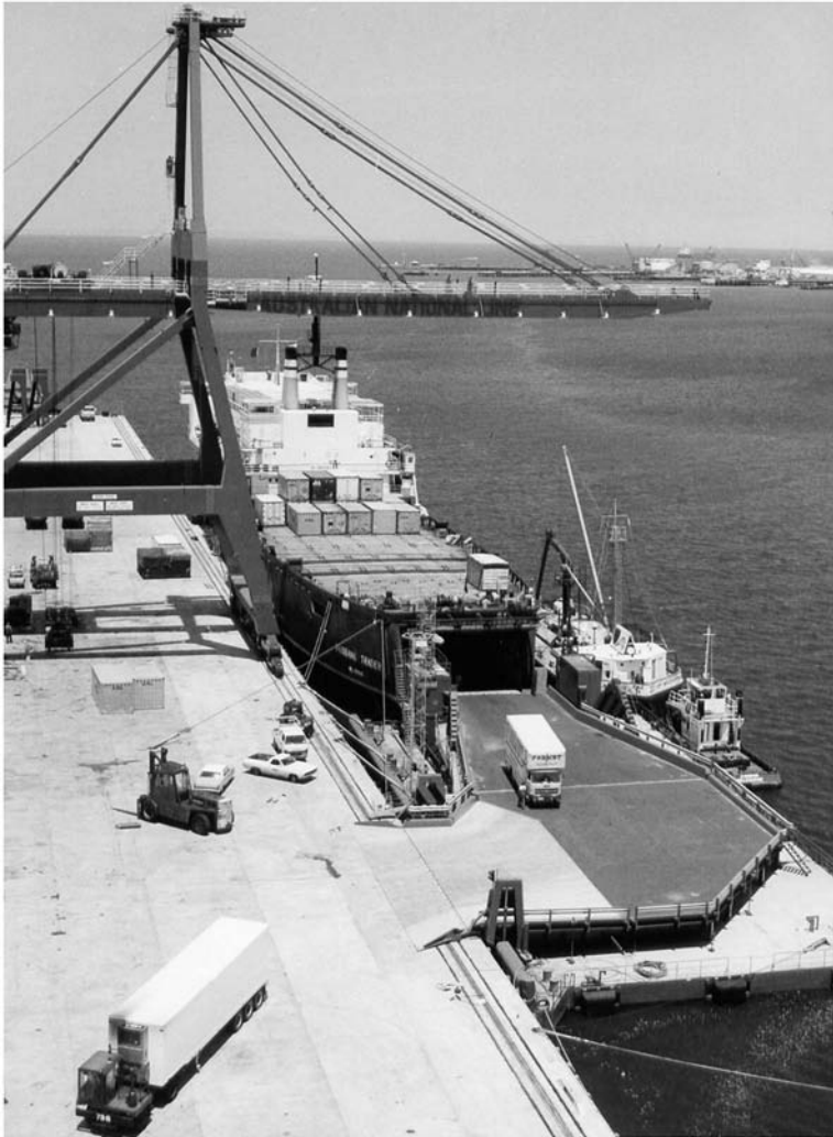
Fig. 9-3. Dockside movable “link-span” pontoon mounted transfer bridge for Ro/Ro cargo transfer at Melbourne, Australia
