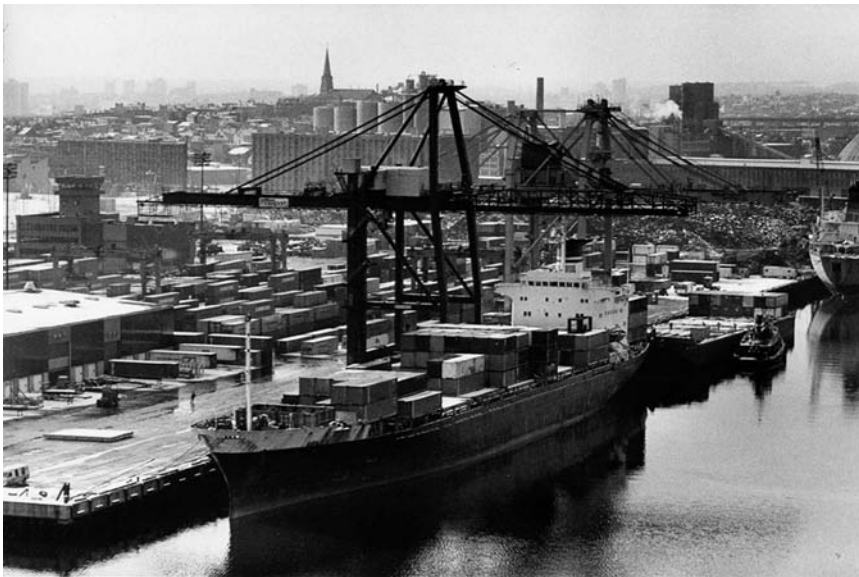
Fig. 1-4. A contemporary small- to medium-sized container terminal with dual container cranes. Note stacking area and control tower in background
