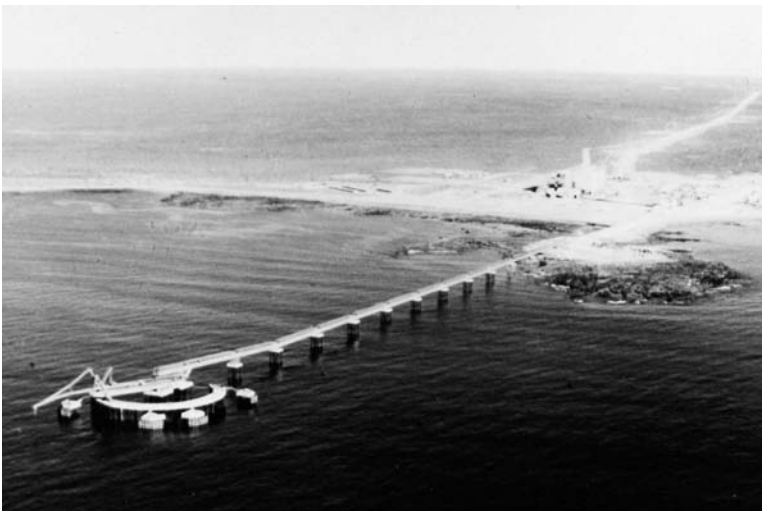
Fig. 6-4. Variable orientation. Offshore loading terminal at Punta Colorada, Argentina
