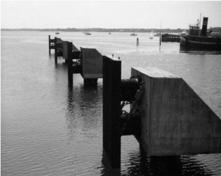
Fig. 7-24. Concrete cap breasting dolphins with resilient rubber fender units and face panels
