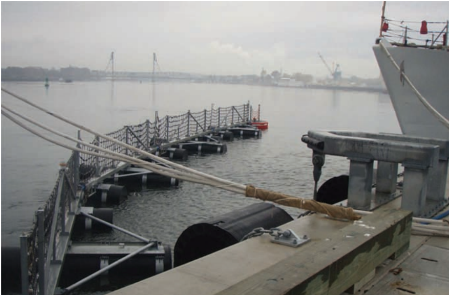
Fig. 9-5. Port security barrier
