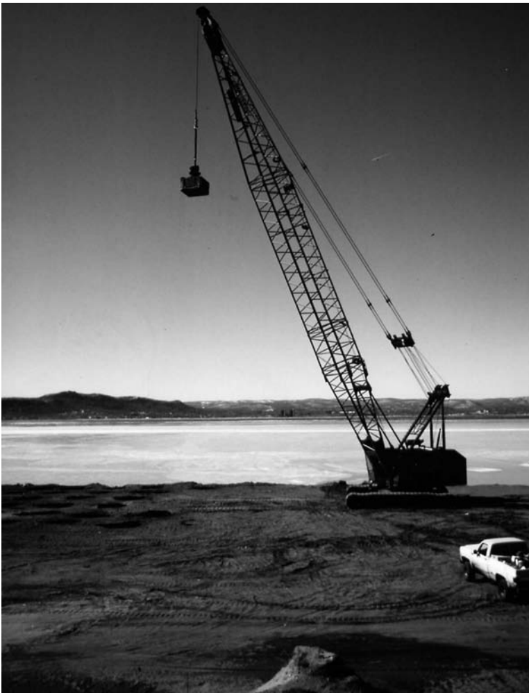
Fig. 8-38. Deep dynamic compaction
