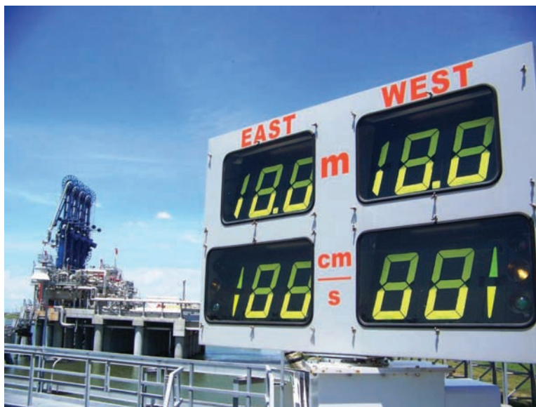
Fig. 5-5. Docking aid system (DAS) display board mounted on mooring dolphin showing vessel distance off and approach speed at fore and aft locations. Note red, yellow, and green warning lights
