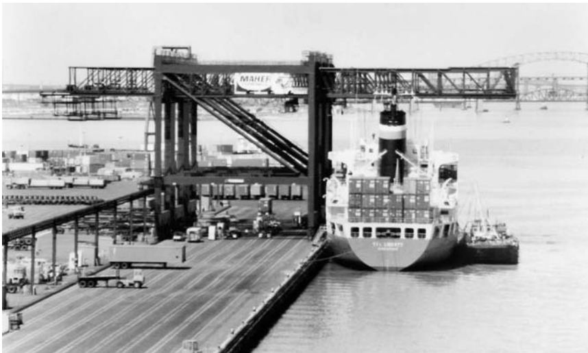
Fig. 4-8. Low-profile-type container crane in use at Port Elizabeth, NJ
