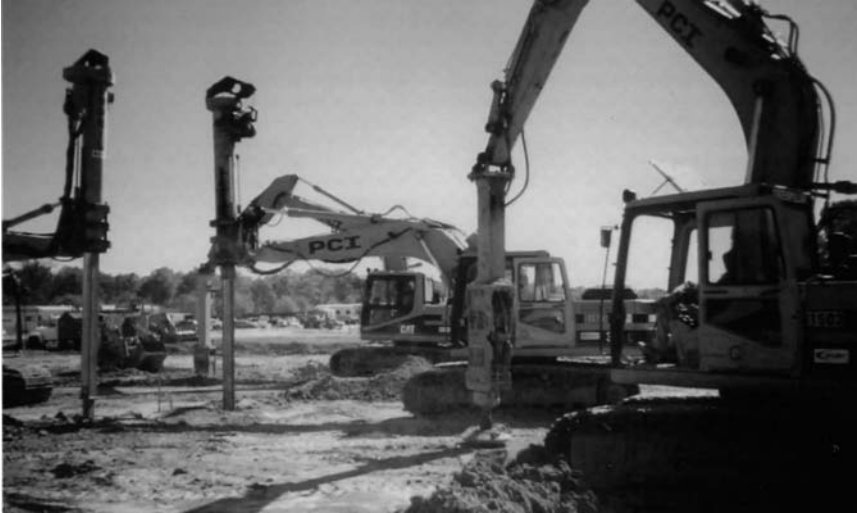
Fig. 8-36. Rammed aggregate pier installation
