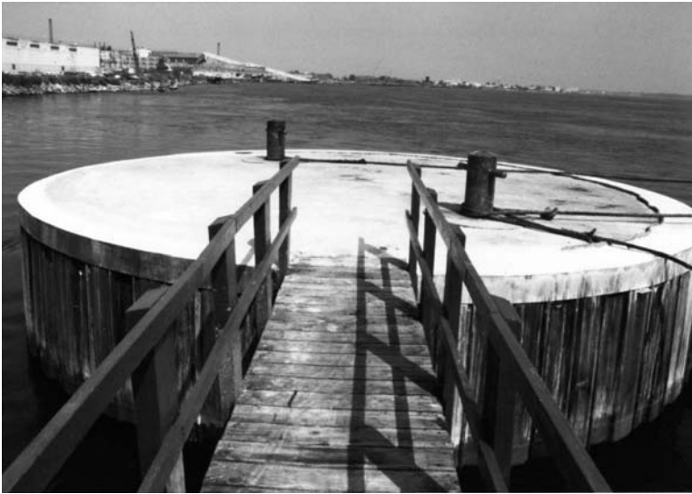
Fig. 8-18. Solid-fill steel-sheet-pile dolphin
