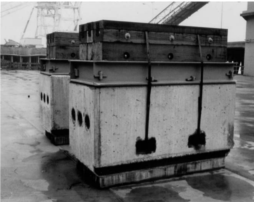
Fig. 10-1. Block with sand frame for easy removal
