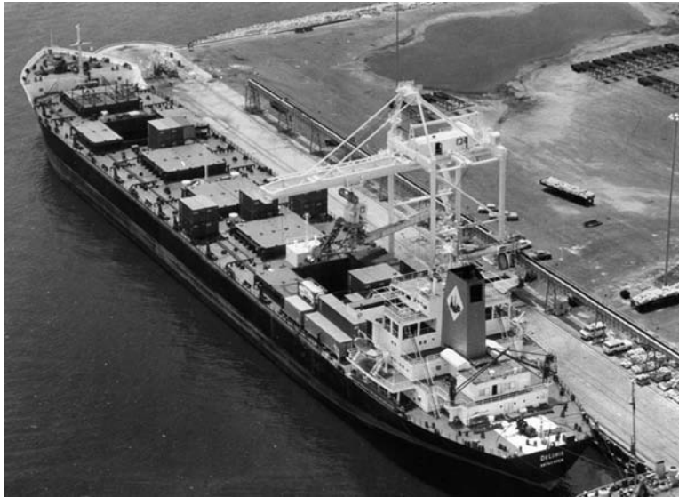
Fig. 1-5. A bulk cargo terminal facility equipped with a catenary continuous unloader, multipurpose Portainer crane
