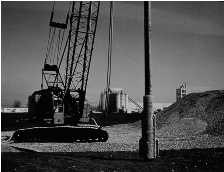
Fig. 8-33. Stone column vibro-replacement equipment
