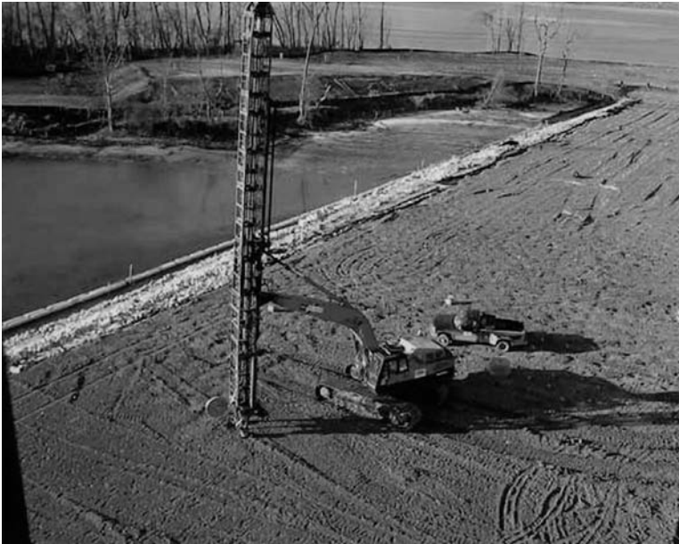
Fig. 8-39. Typical wick drain installation equipment
