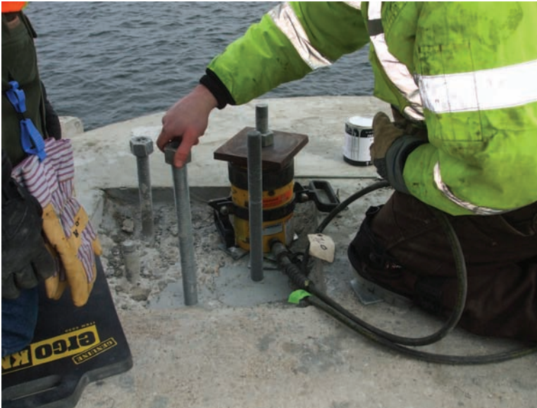
Fig. 11-24. Testing of postinstalled anchor bolts using a hydraulic jack
