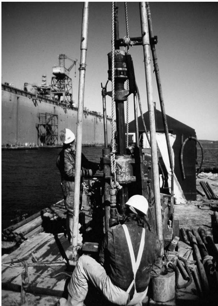
Fig. 8-2. Typical float-mounted drill rig
