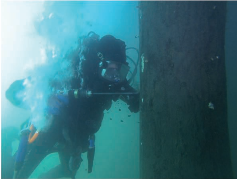
Fig. 12-8. Engineer-diver drilling into a timber pile
