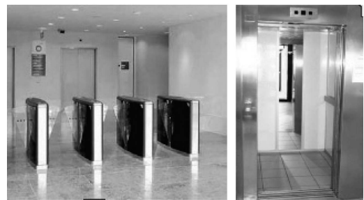
Figure 5. Access control with RFID.
